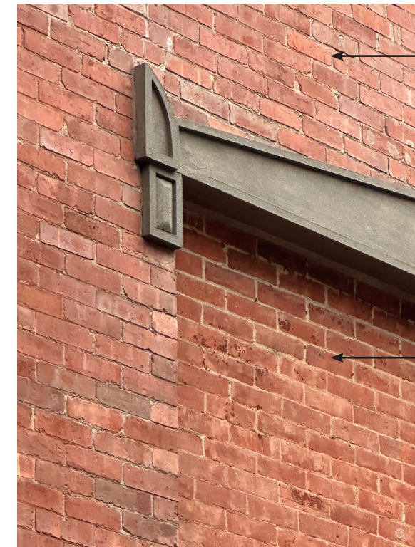
Existing Stone Lintel Detail
