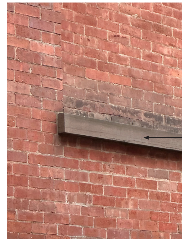
Existing Stone Sill Detail
