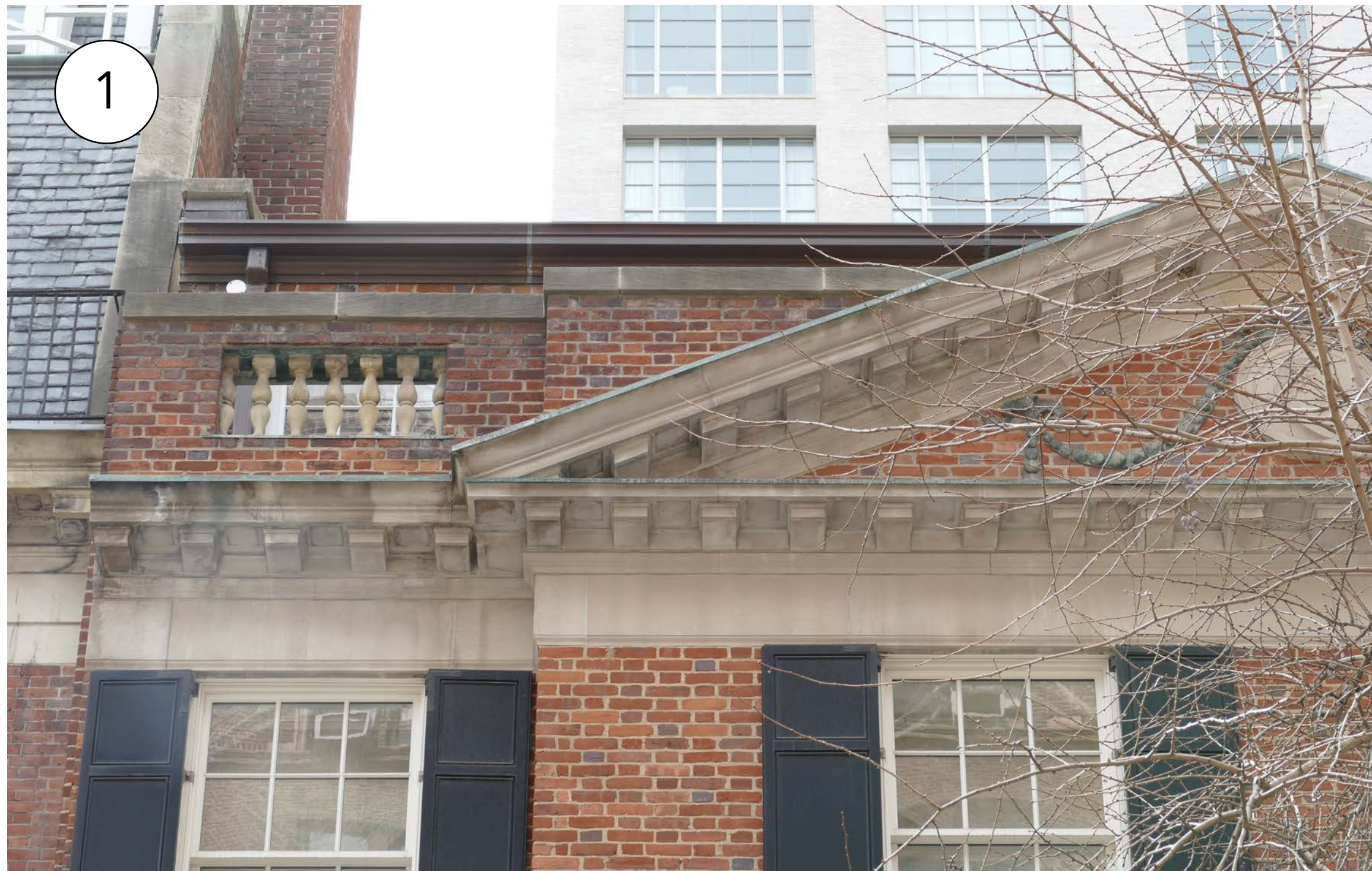
1 Limestone pediment and cornice in good condition; areas of minor soiling
