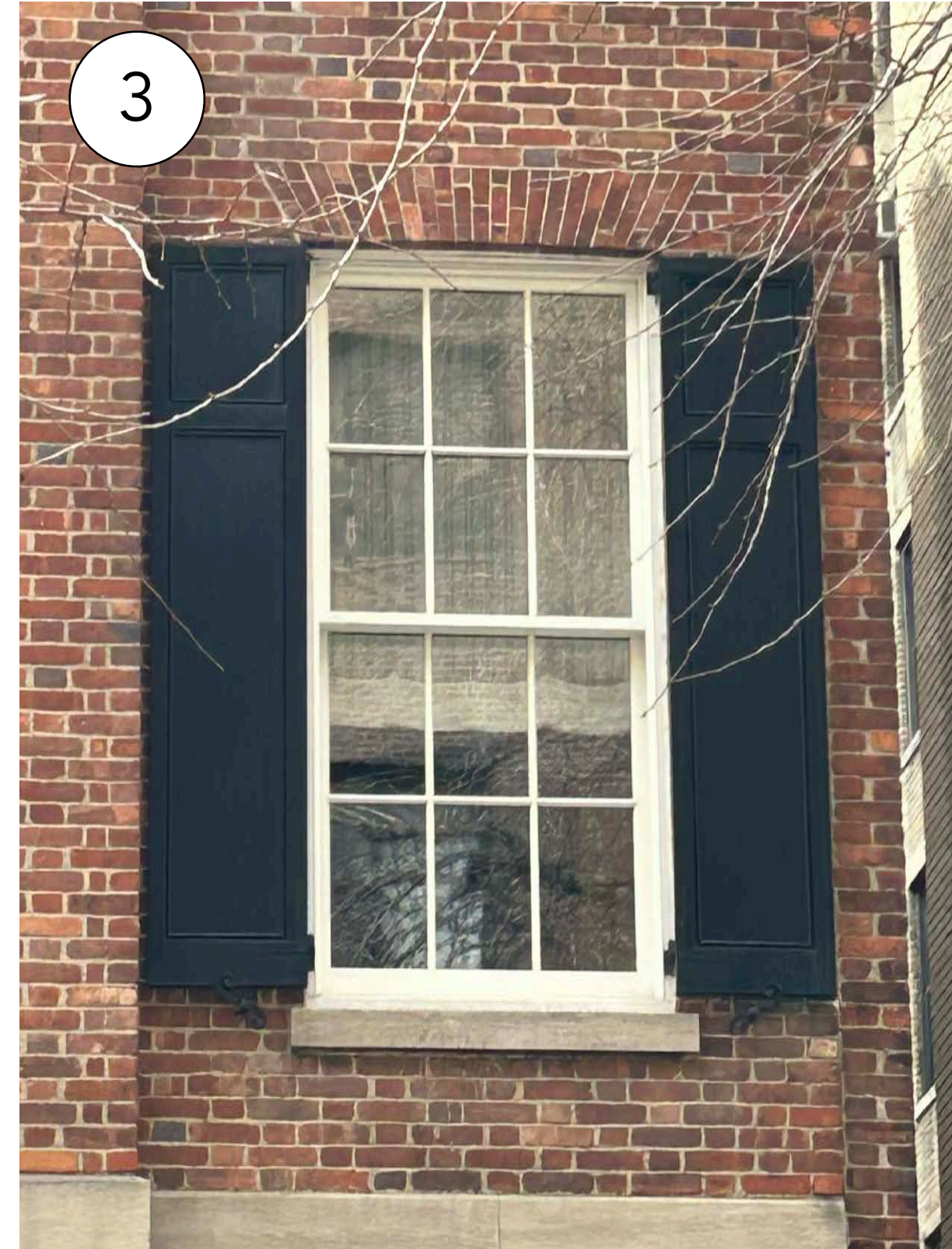
3 Second-floor, six-over-six wood windows with existing shutters.
