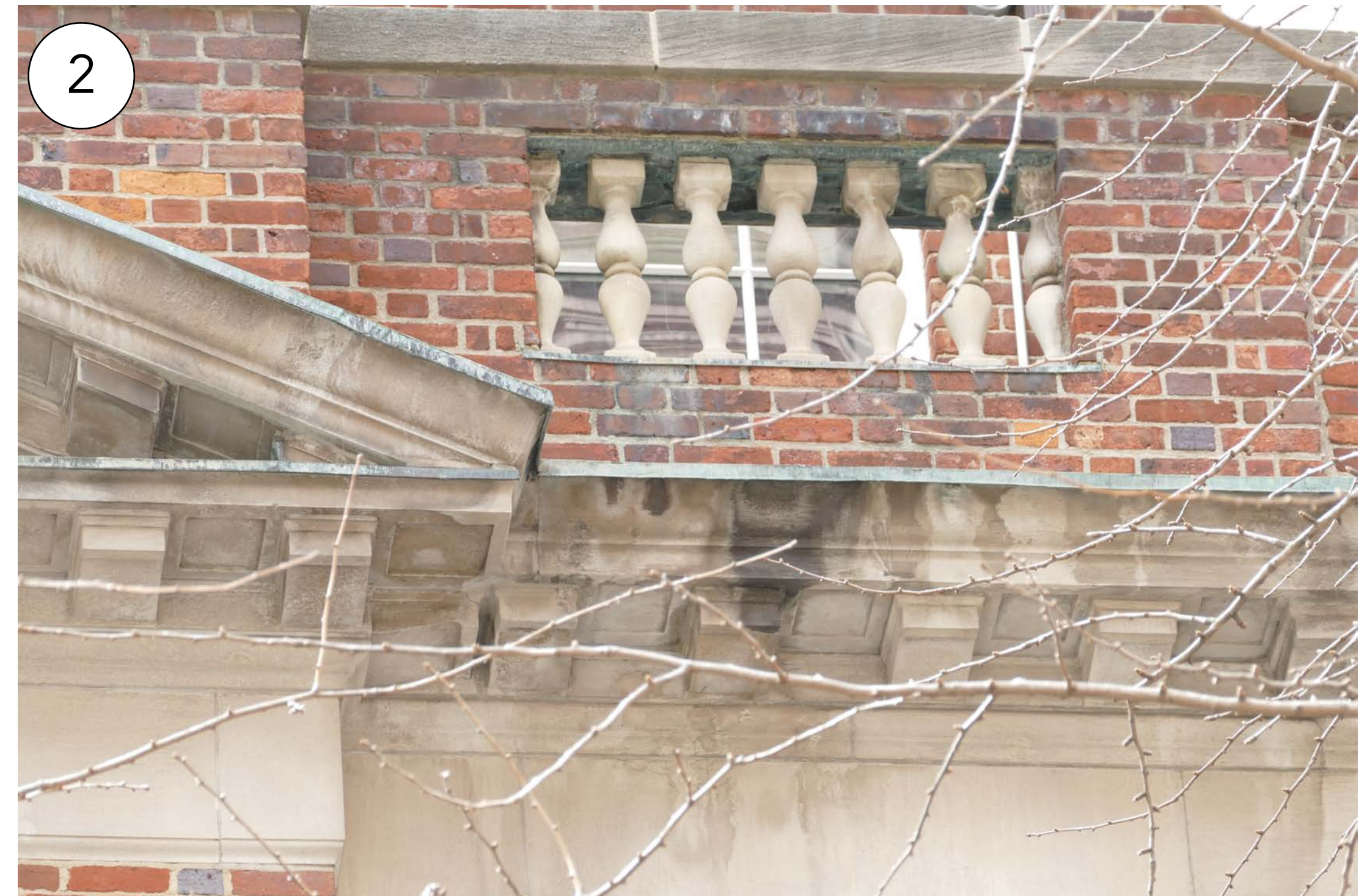
2 Balusters and cornice in good condition; some areas of soiling and water staining
