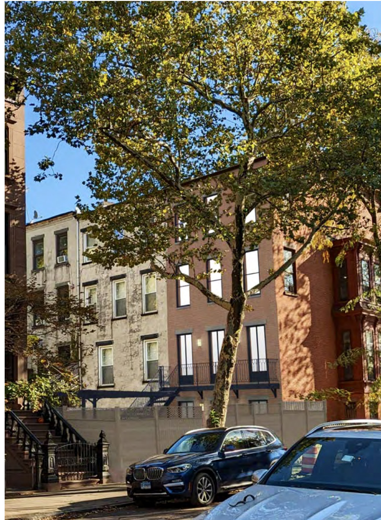
109 Halsey St, Brooklyn (left) Bedford Historic District Docket No.: LPC-19-09977 Approved: 2017 (C of A)
