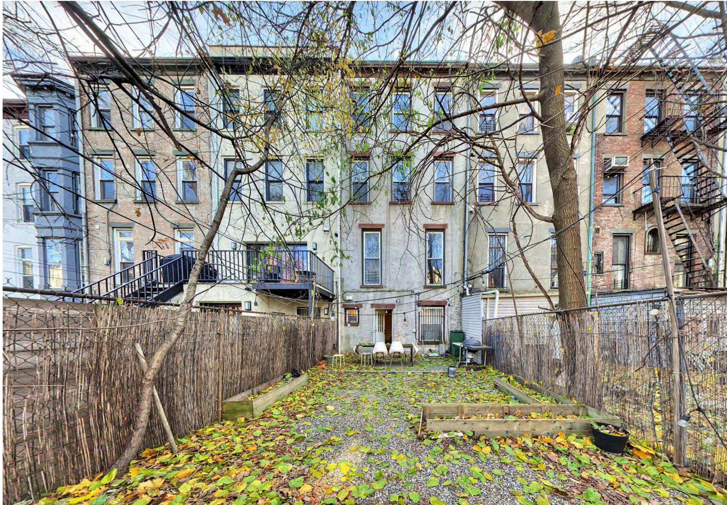
Existing Rear Facade and Adjacent Context
