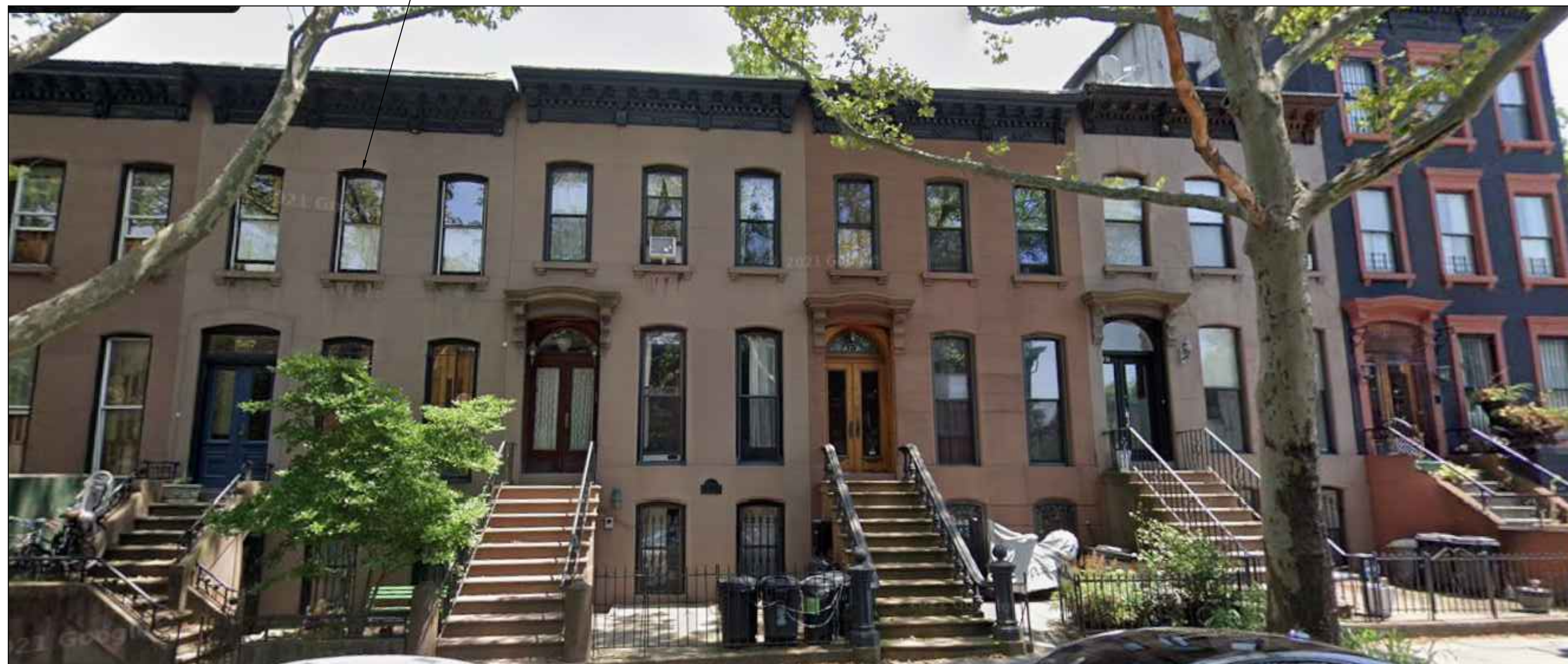
BLDG. # 567 RECTANGULAR WINDOWS WITHIN ARCH OPENING
