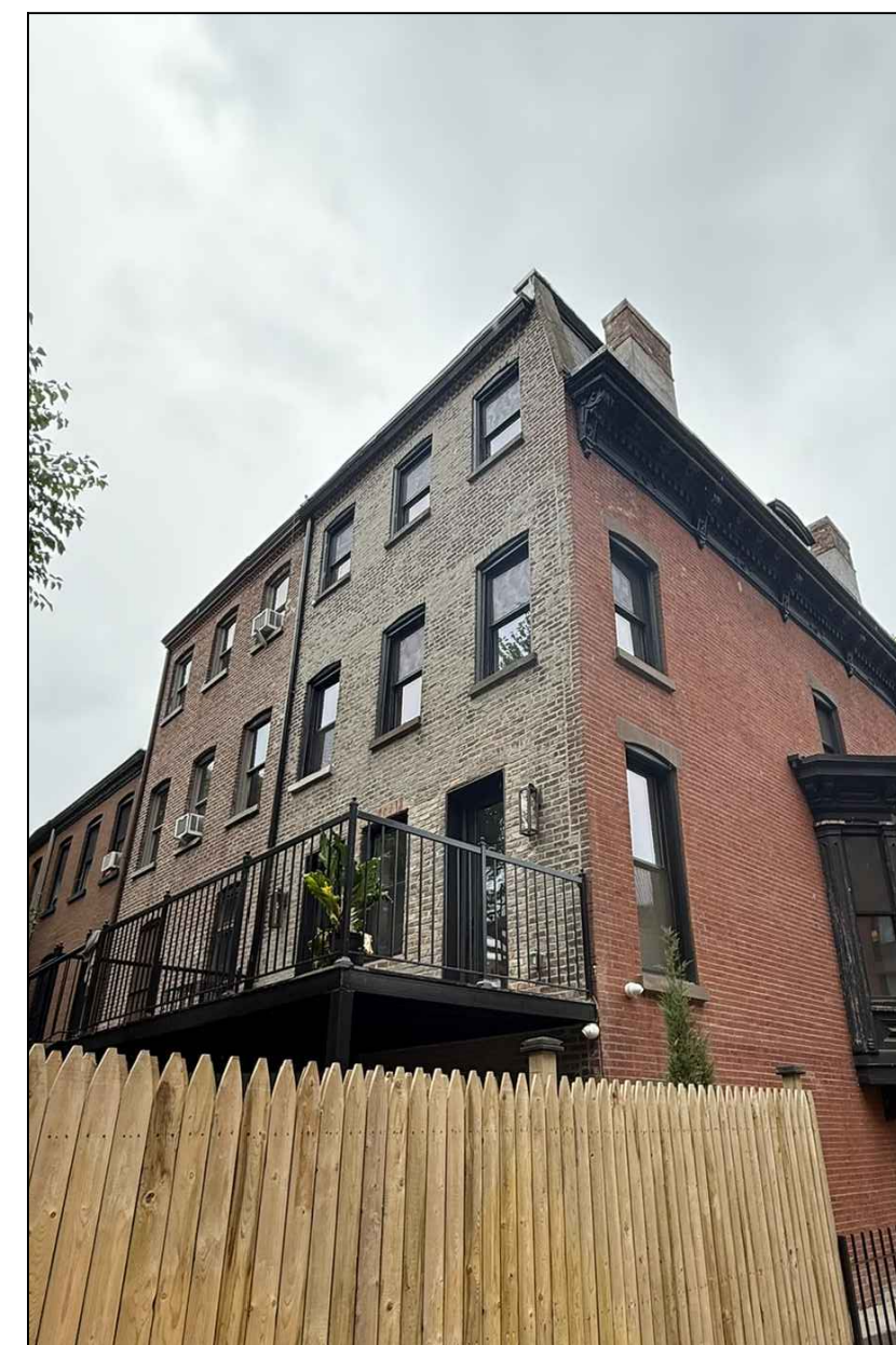
**VIEW 4 AS BUILT CONDITION WITH AC UNITS ON ROOF REAR VIEW - EASEMENT SCALE: N.T.S.
