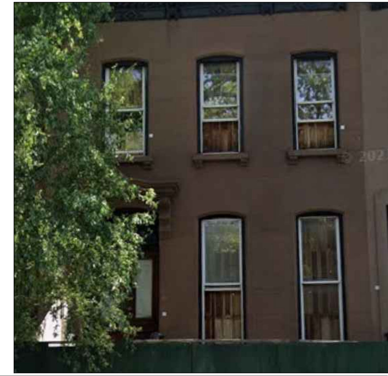
BLDG. # 567 RECTANGULAR WINDOWS WITHIN ARCH OPENING
