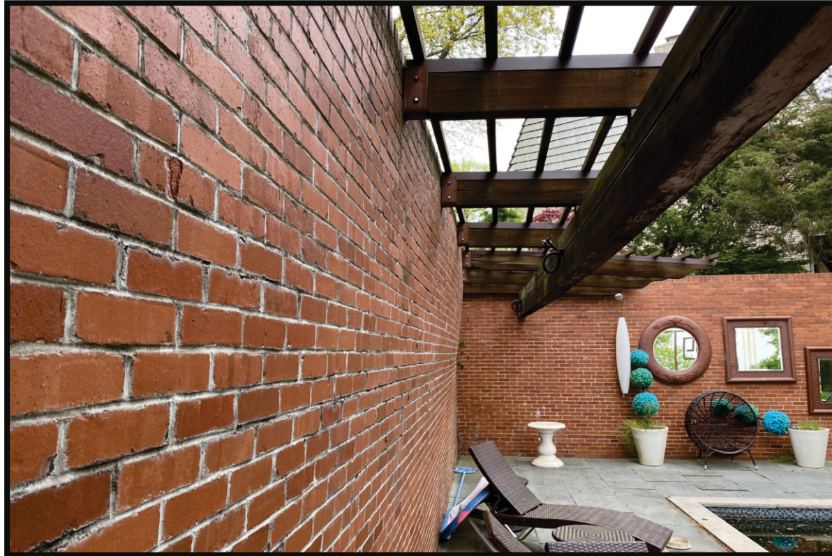
Photograph showing brick retaining wall.
