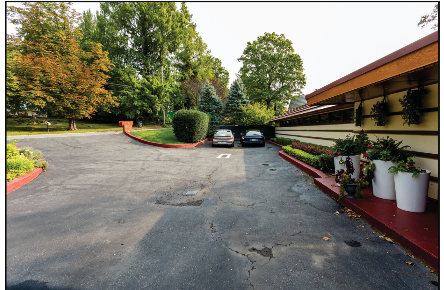
Photograph showing modified driveway
