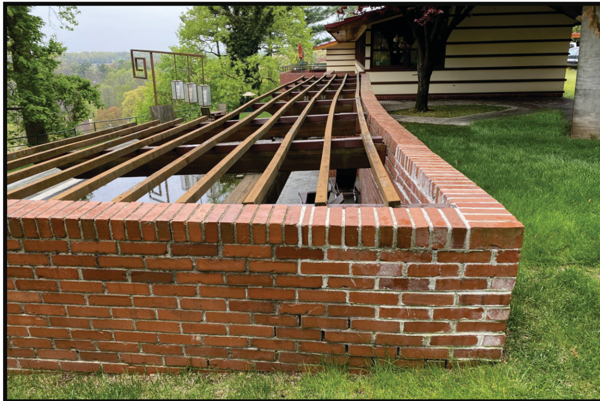
Extended brick wall to be replaced with railing.
