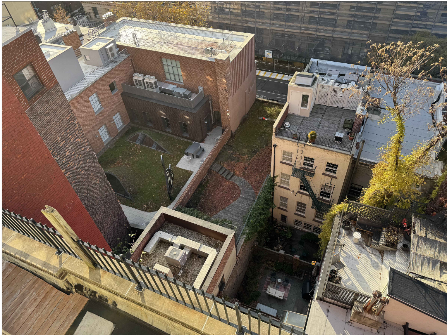
Photo 4: From 35 Bethune Street Looking Southwest towards Washington Street
