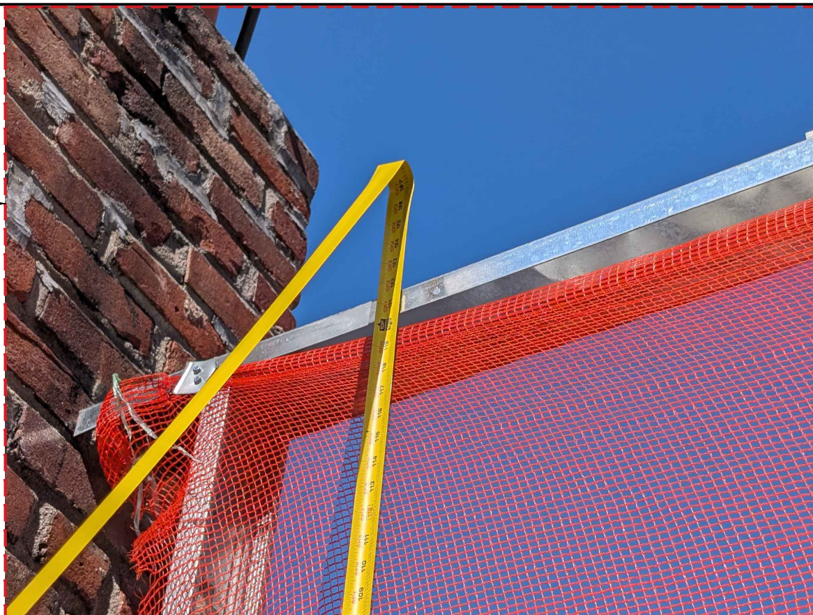
CLOSE UP OF ADDITION VIEW 1
