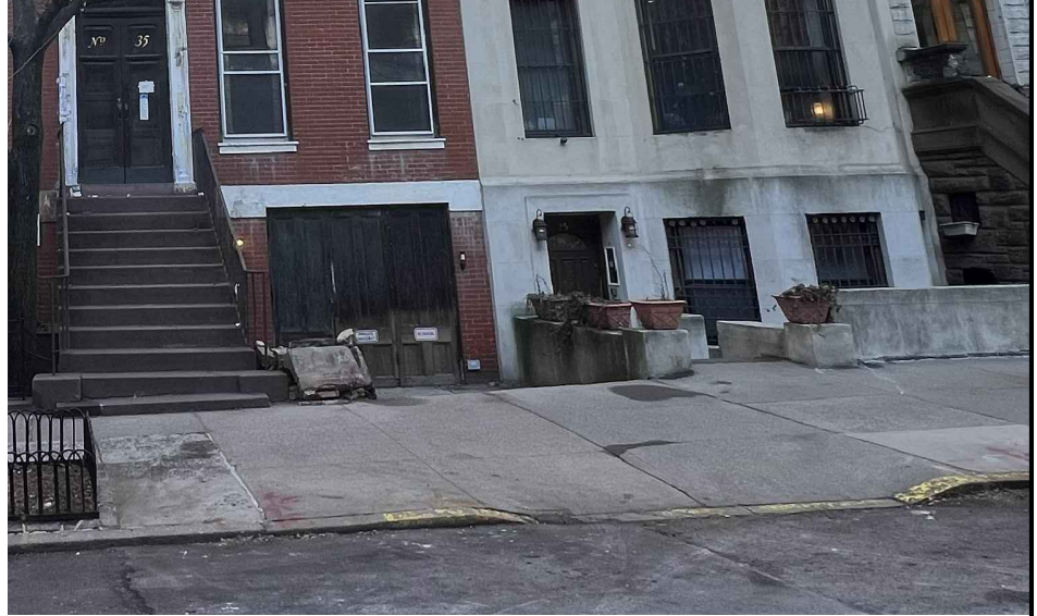
VIEW OF CONCRETE SIDEWALK & CURB CUT
