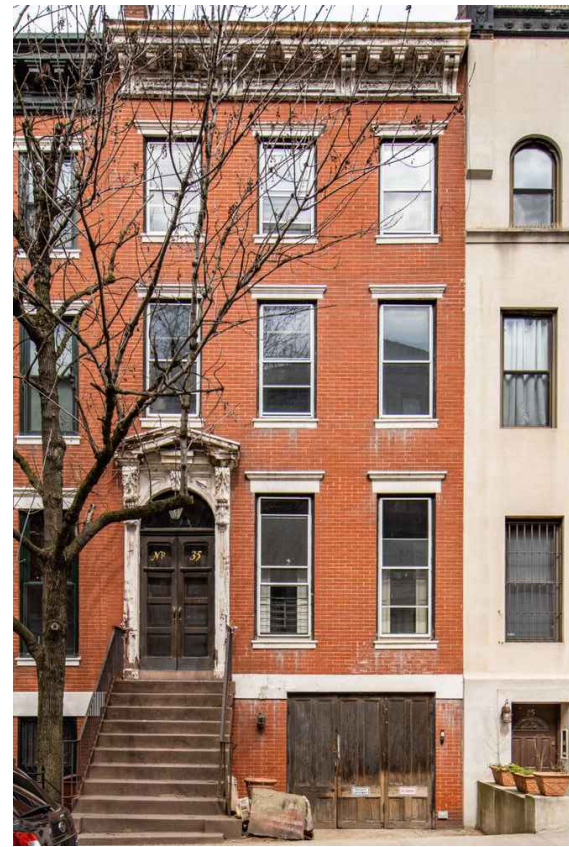
SUBJECT SITE FRONT FACADE
