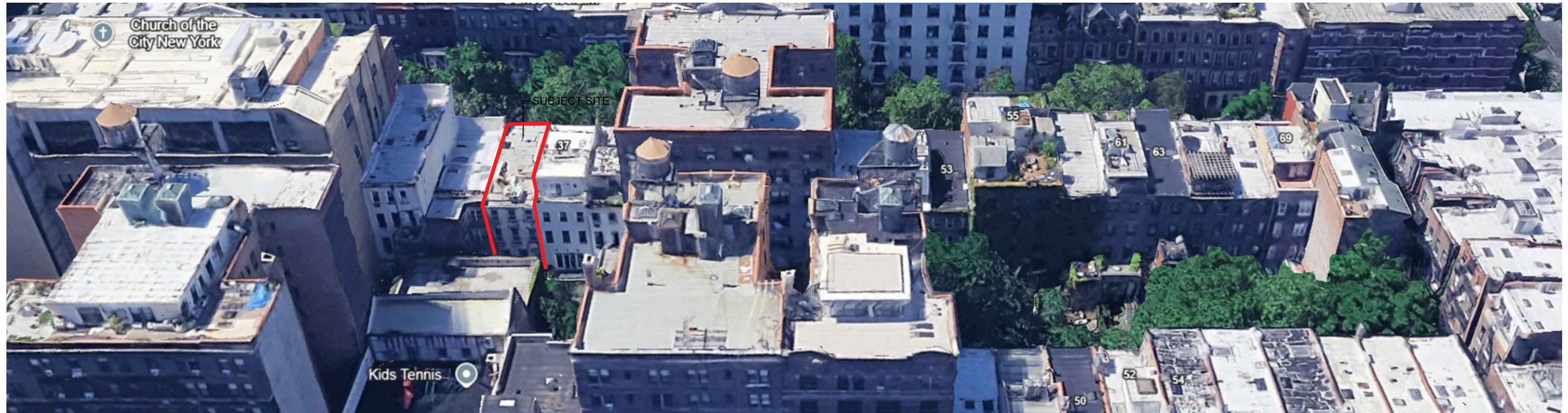
AERIAL PHOTO SHOWING REAR VIEW OF TOP FLOORS WITHIN THE BLOCK
