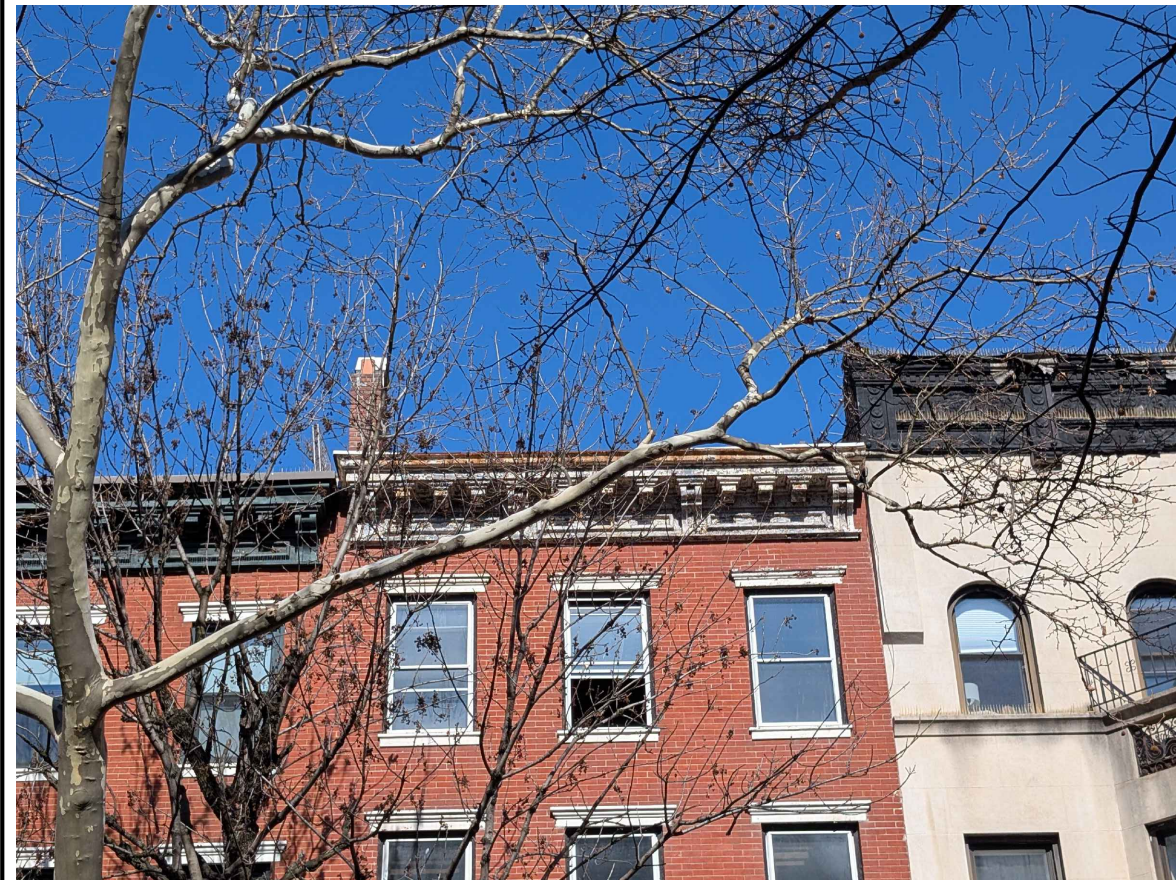
FRONT VIEW - CLOSE UP MOCK UP - NO VISIBILITY
