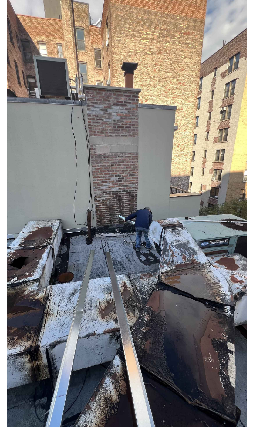
PHOTO 3: NORTH VIEW (#37 ADJ PROPERTY)
