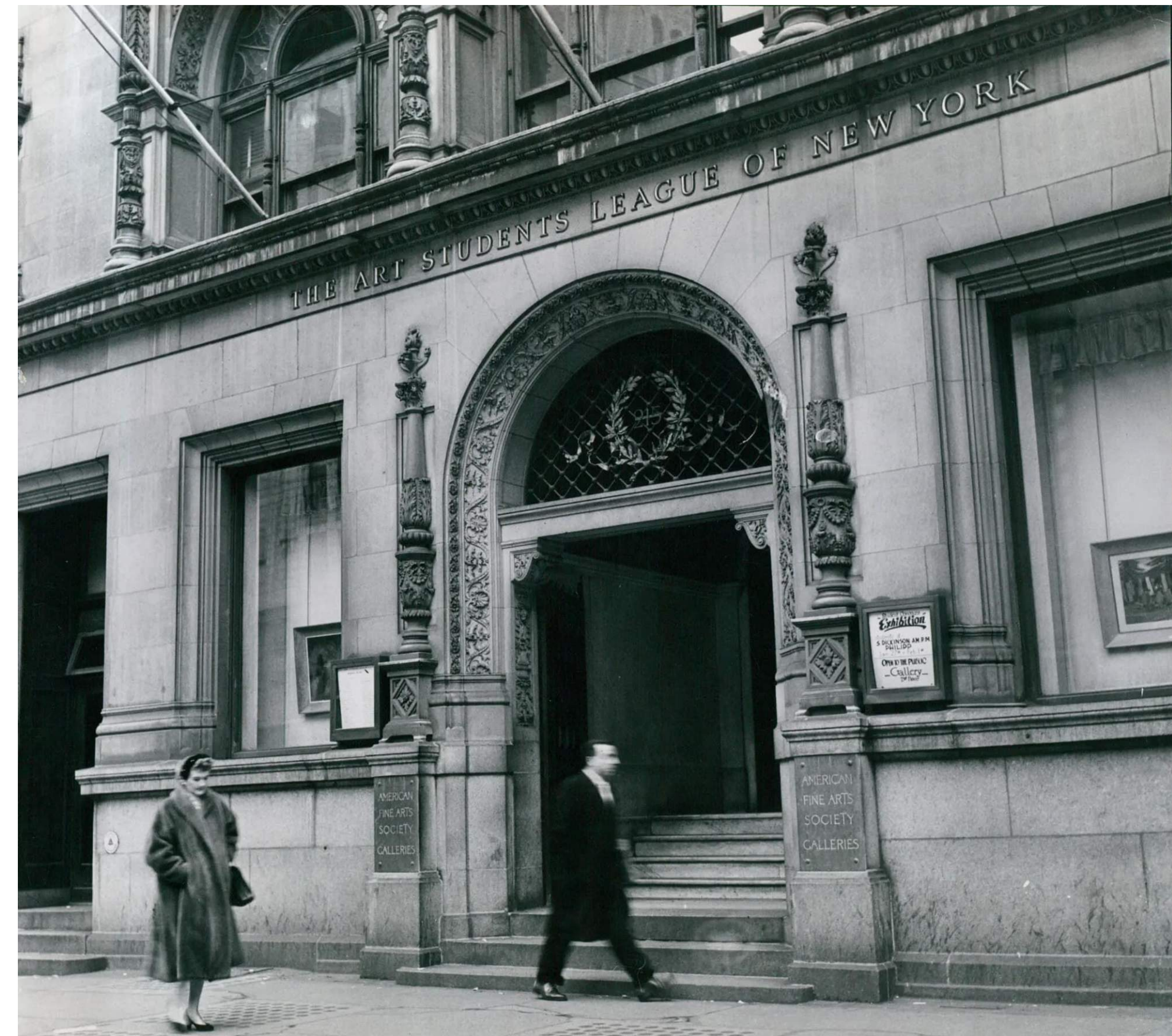
SIGNAGE: Detail view of the American Fine Arts Society building (above) with wood lettering affixed to the main entrance entablature ca. 1950s. The 1968 LPC designation photo shown at left. View of main (south) facade on West 57th Street.
