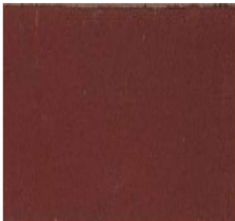
SIDEWALL STUCCO MATCHES BRICK RED
