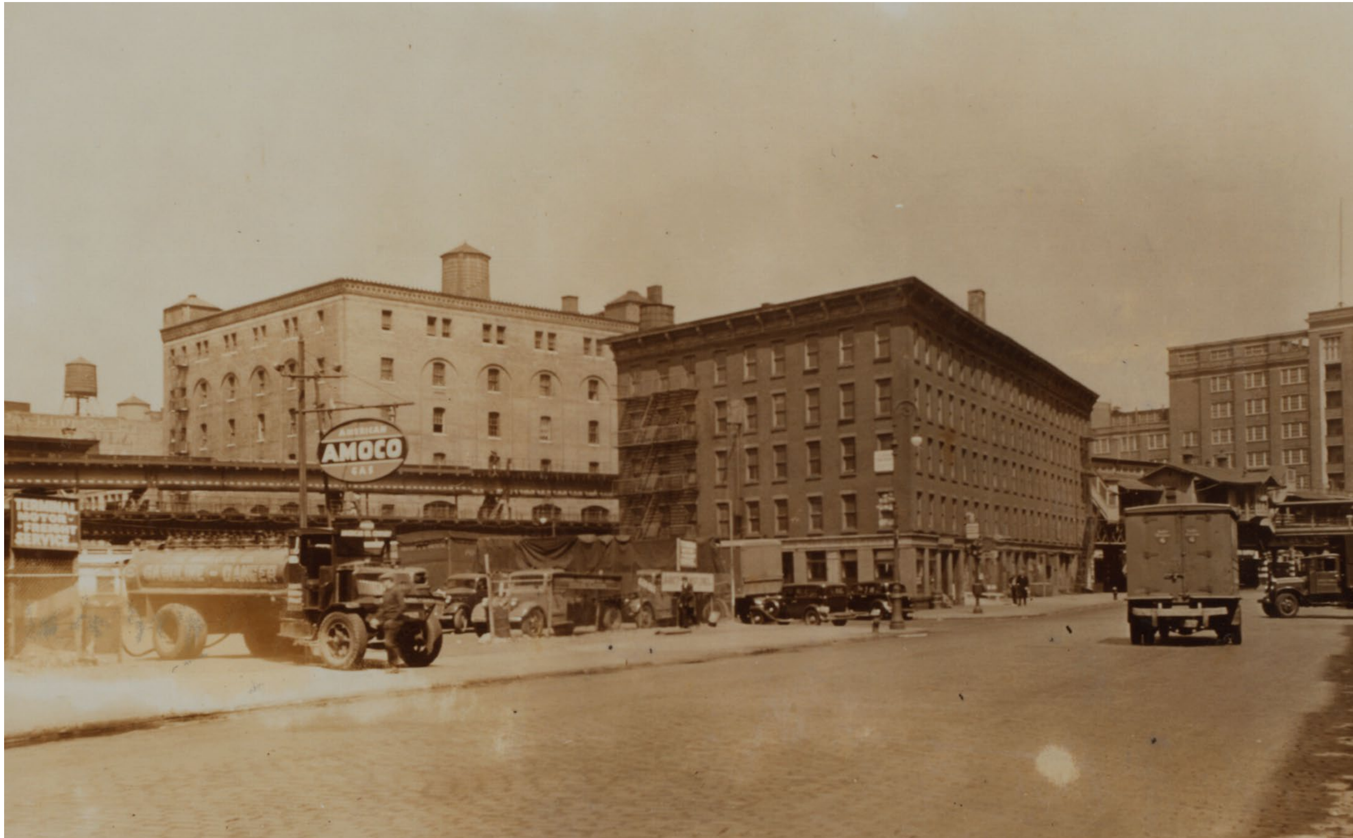
VIEW NORTH ALONG HUDSON STREET FROM WEST 12TH STREET ca 1937 (NYPL)
