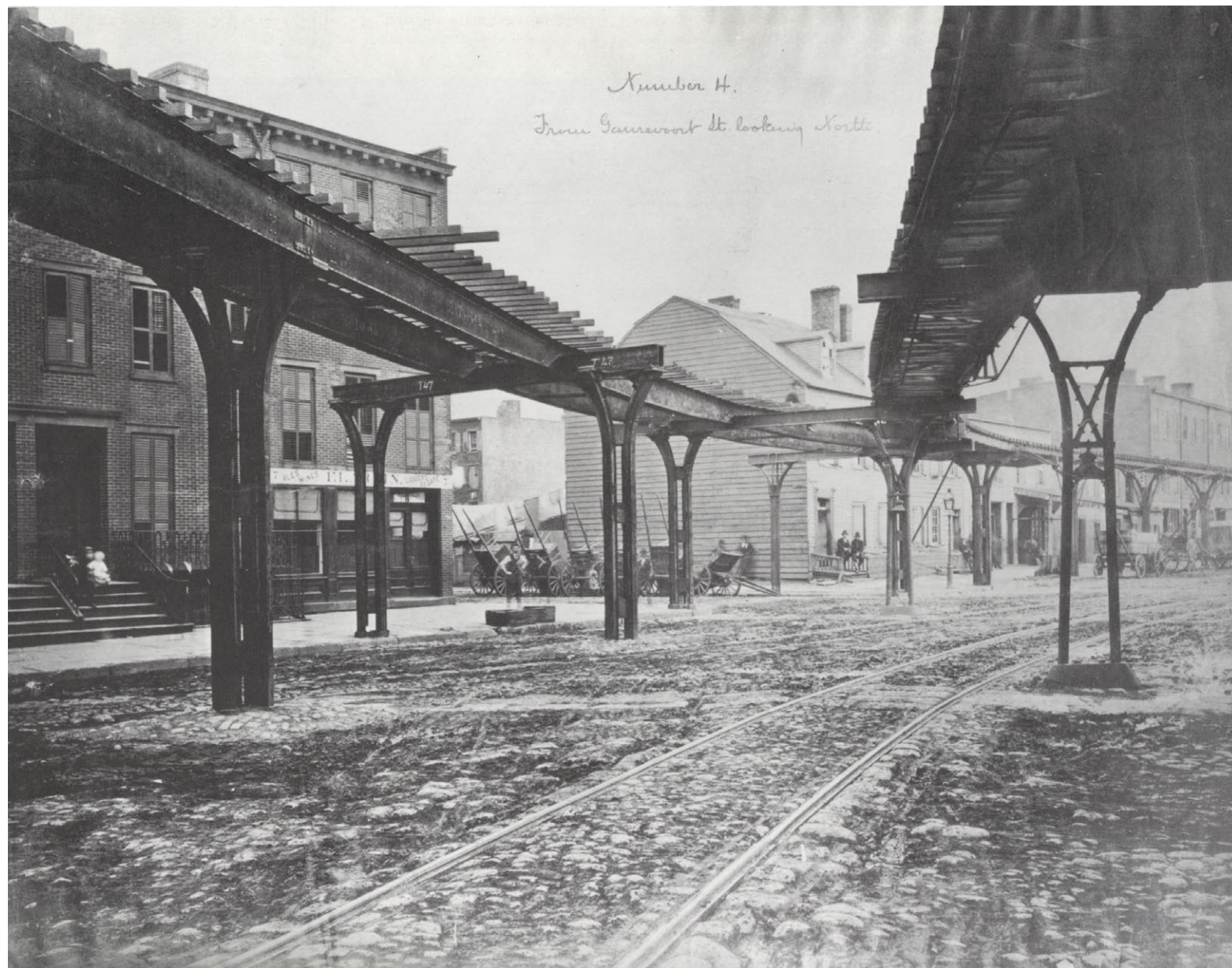
VIEW NORTH UP NINTH AVE FROM GANSEVOORT STREET ca 1876 (NYHS)
