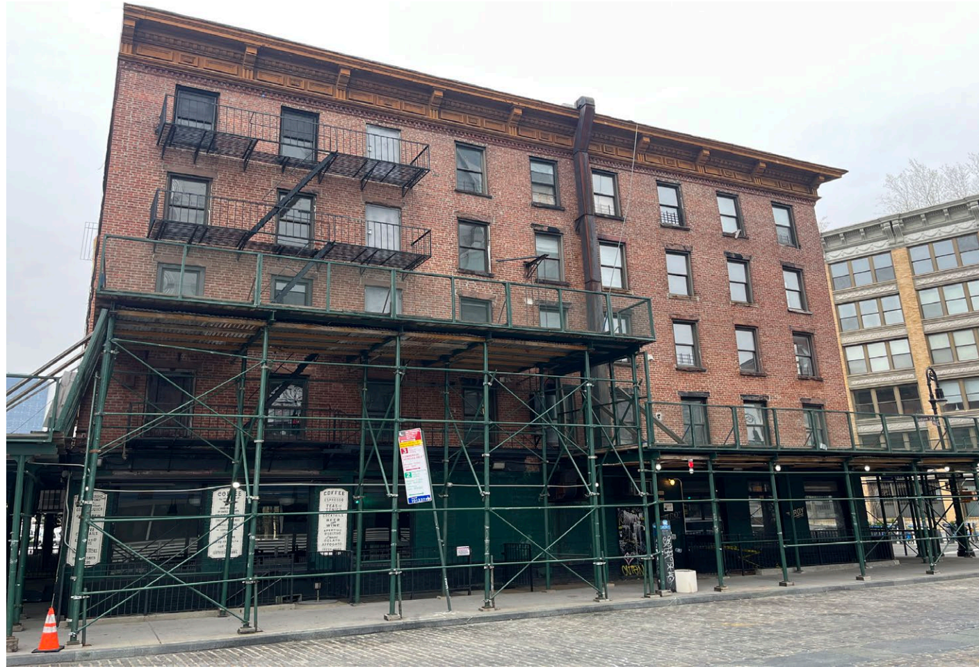
VIEW ON WEST 13TH STREET
