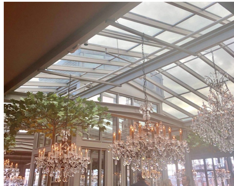
ROOFTOP OF 9-19 9TH AVENUE
