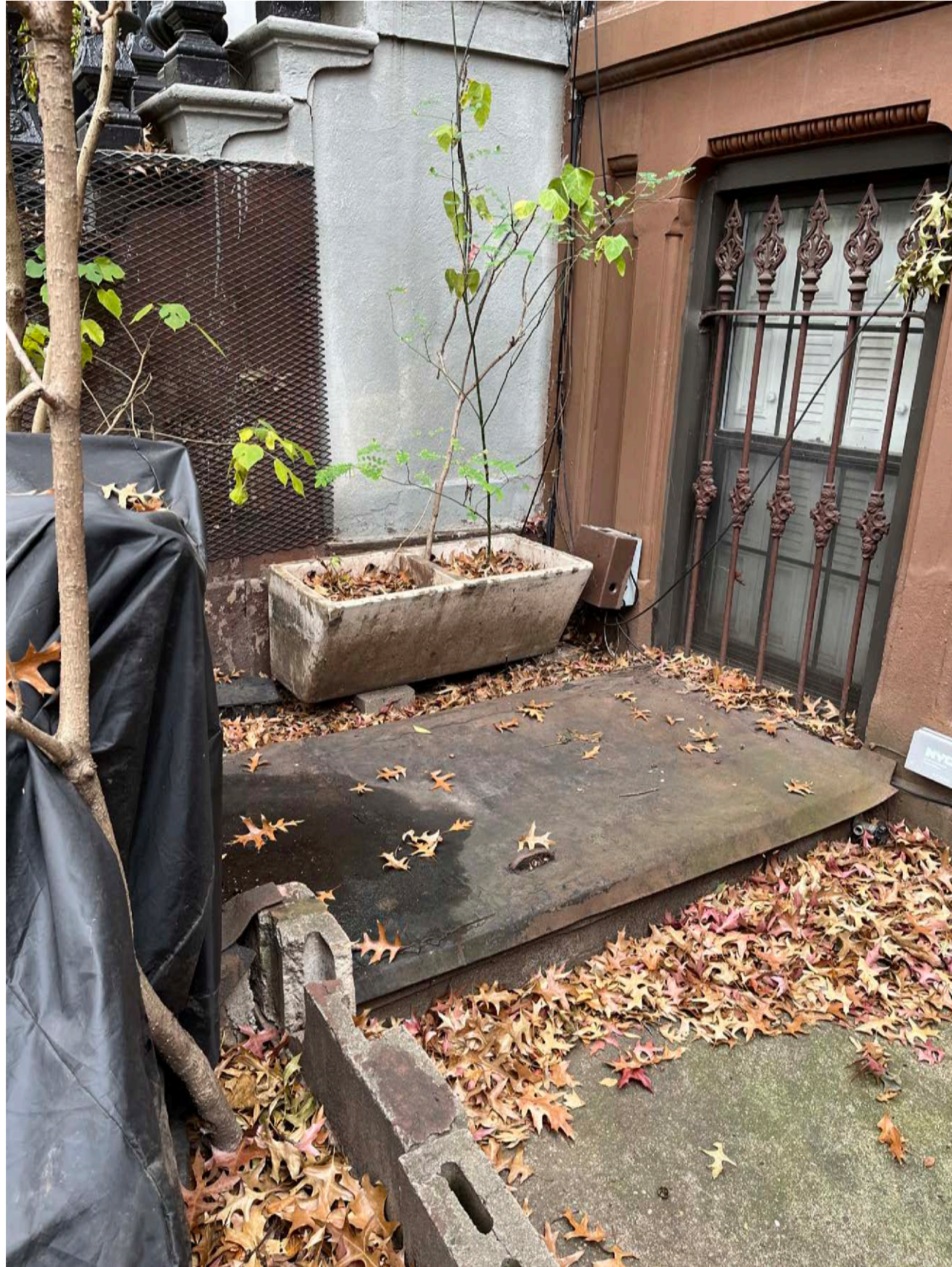
Basement windows and covered cellar hatch
