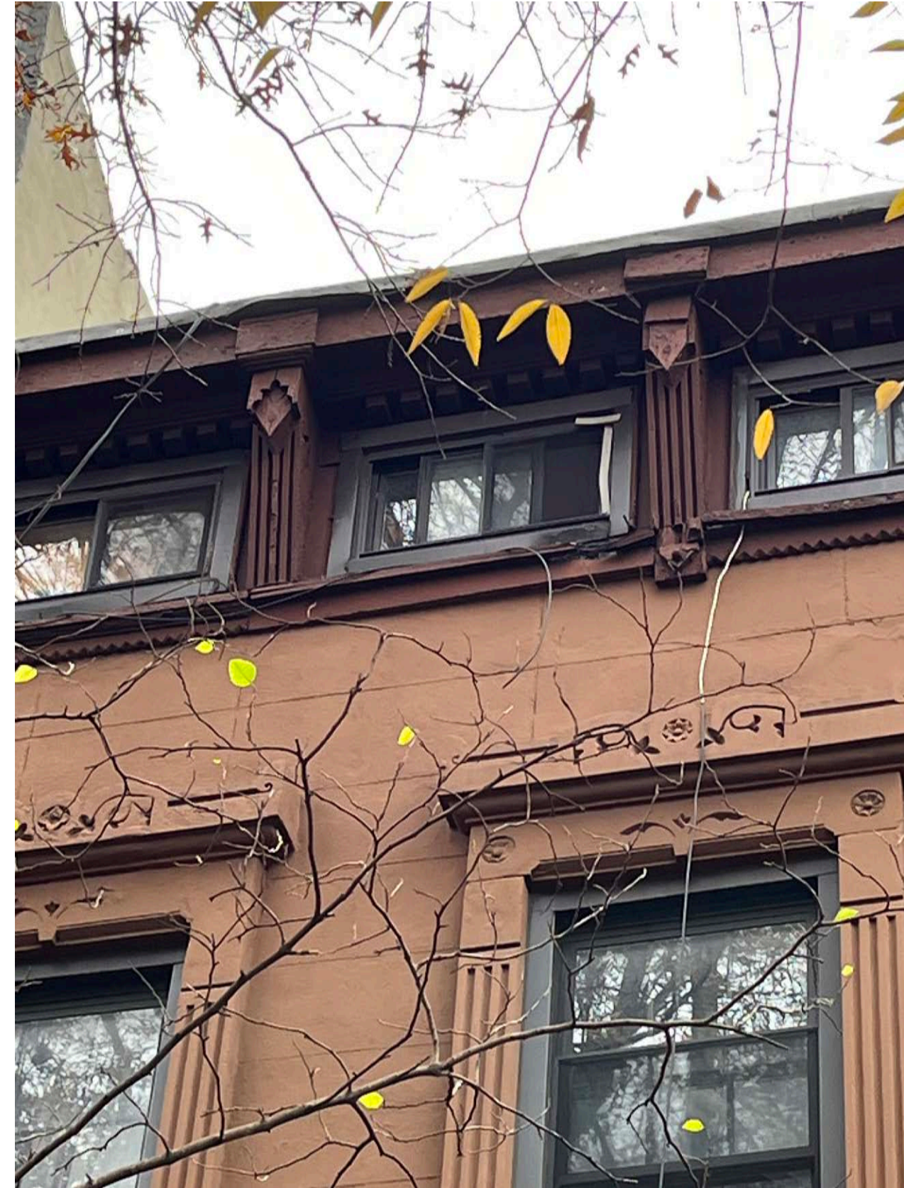
Non-historic windows in cornice
