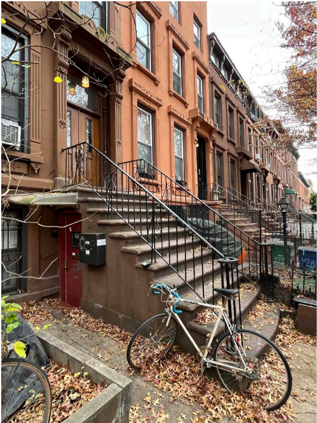
Stoop and basement entry
