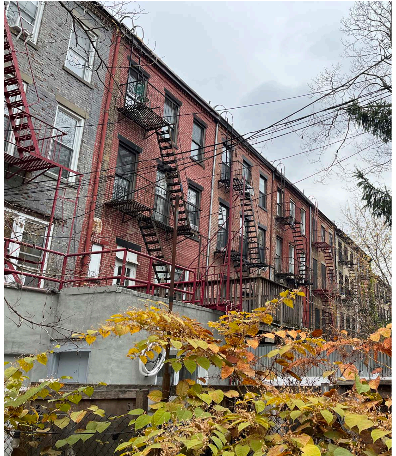
Adjacent rears, facing east
