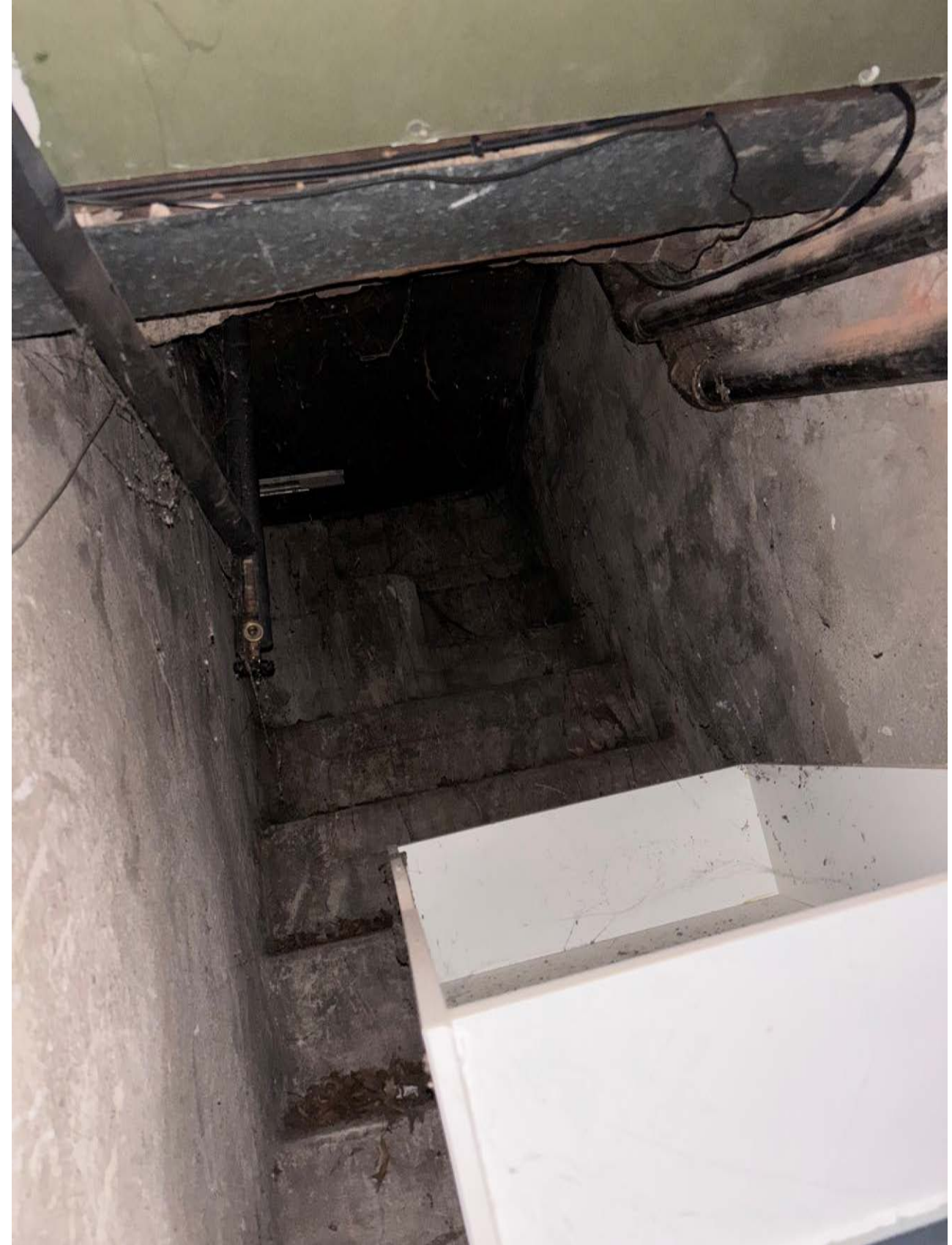
View from cellar of existing steep and shallow hatch
