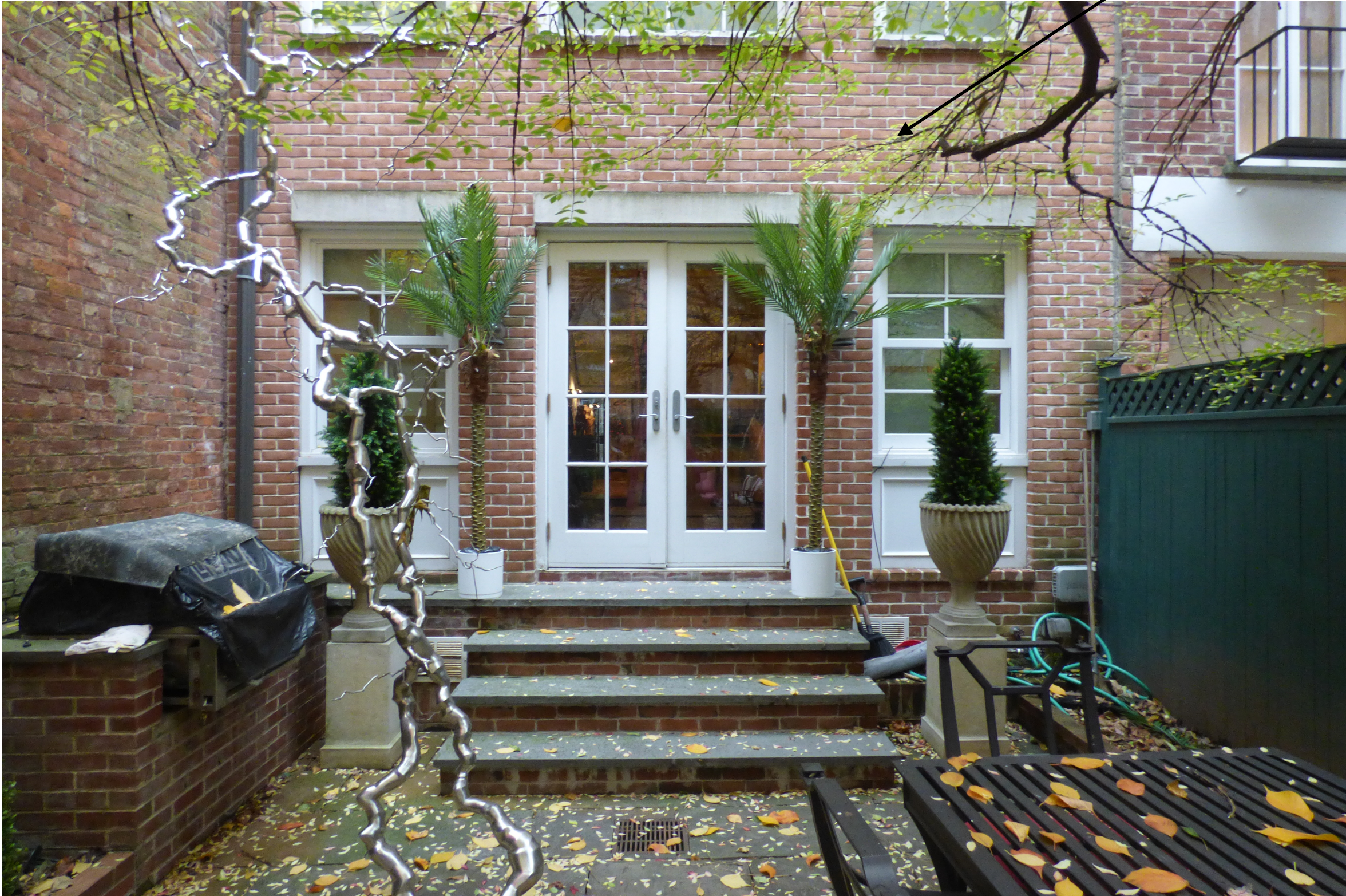
Rear Facade - Existing Conditions
