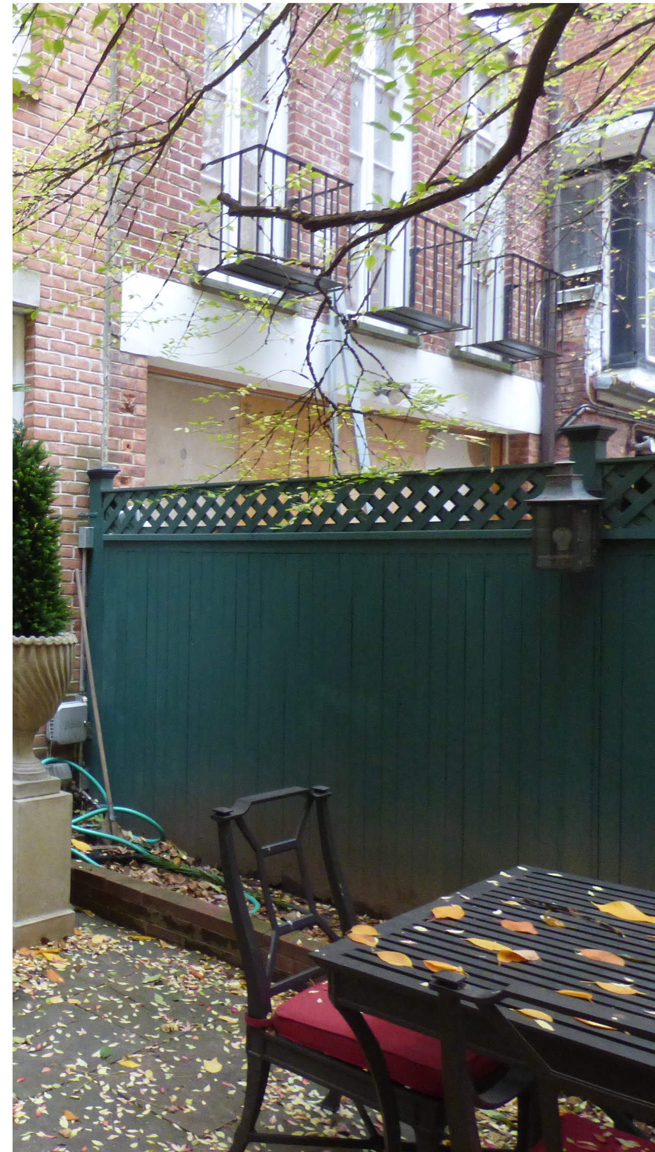
Rear Facade - Existing Conditions, View from the east
