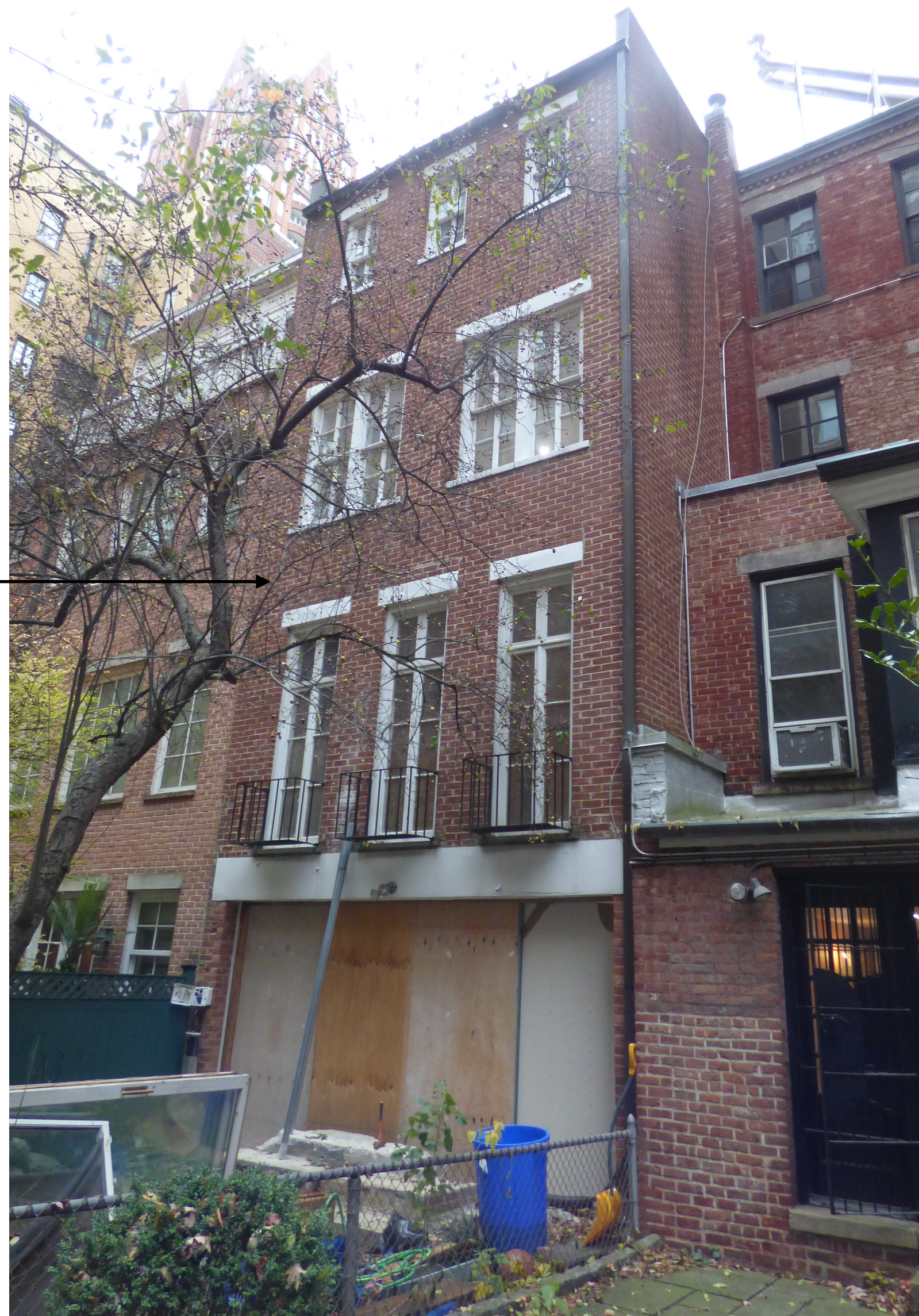
Rear Facade - Existing Conditions, View from the west
