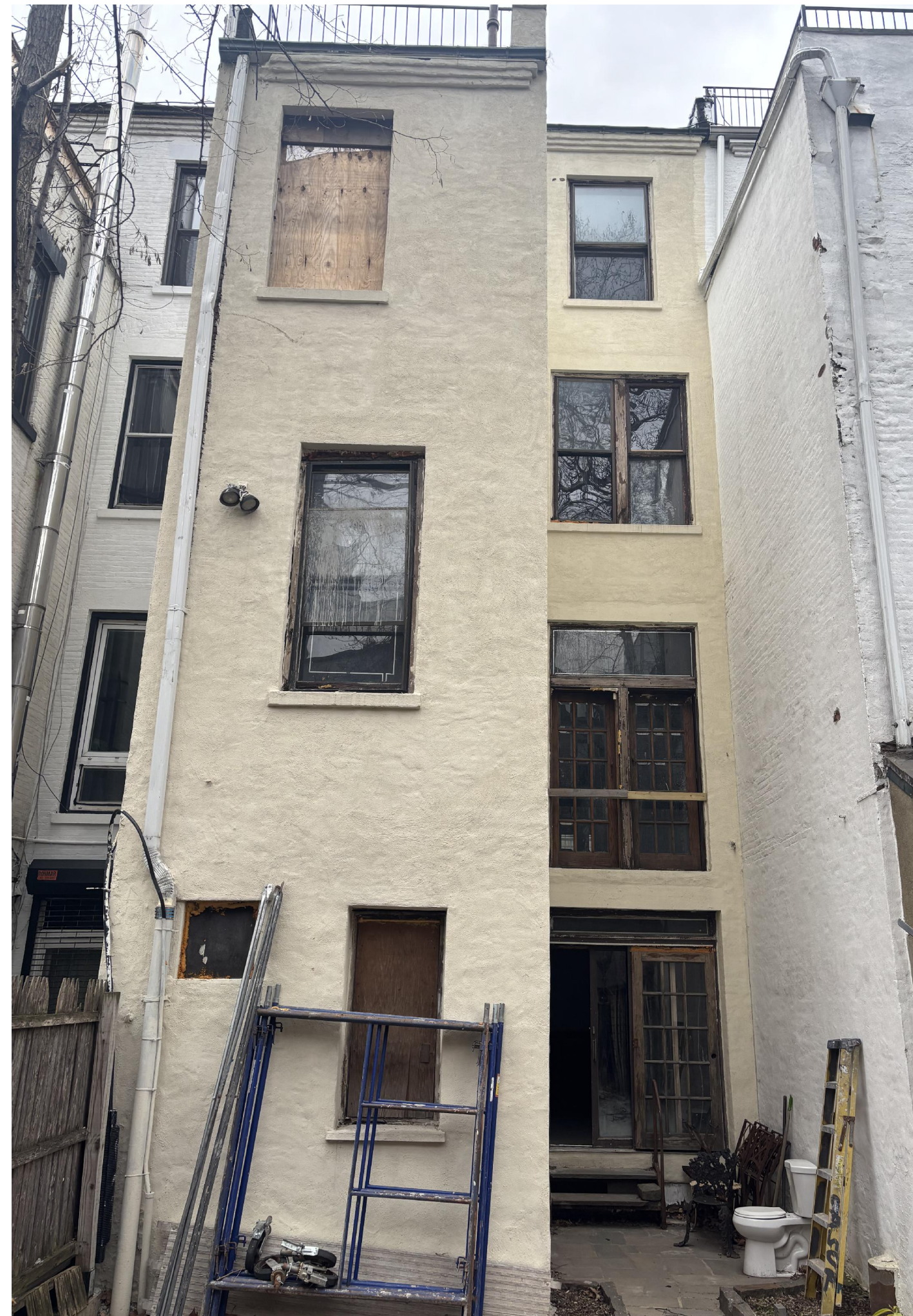
01 140W 88TH STREET - EXISTING REAR FACADE
