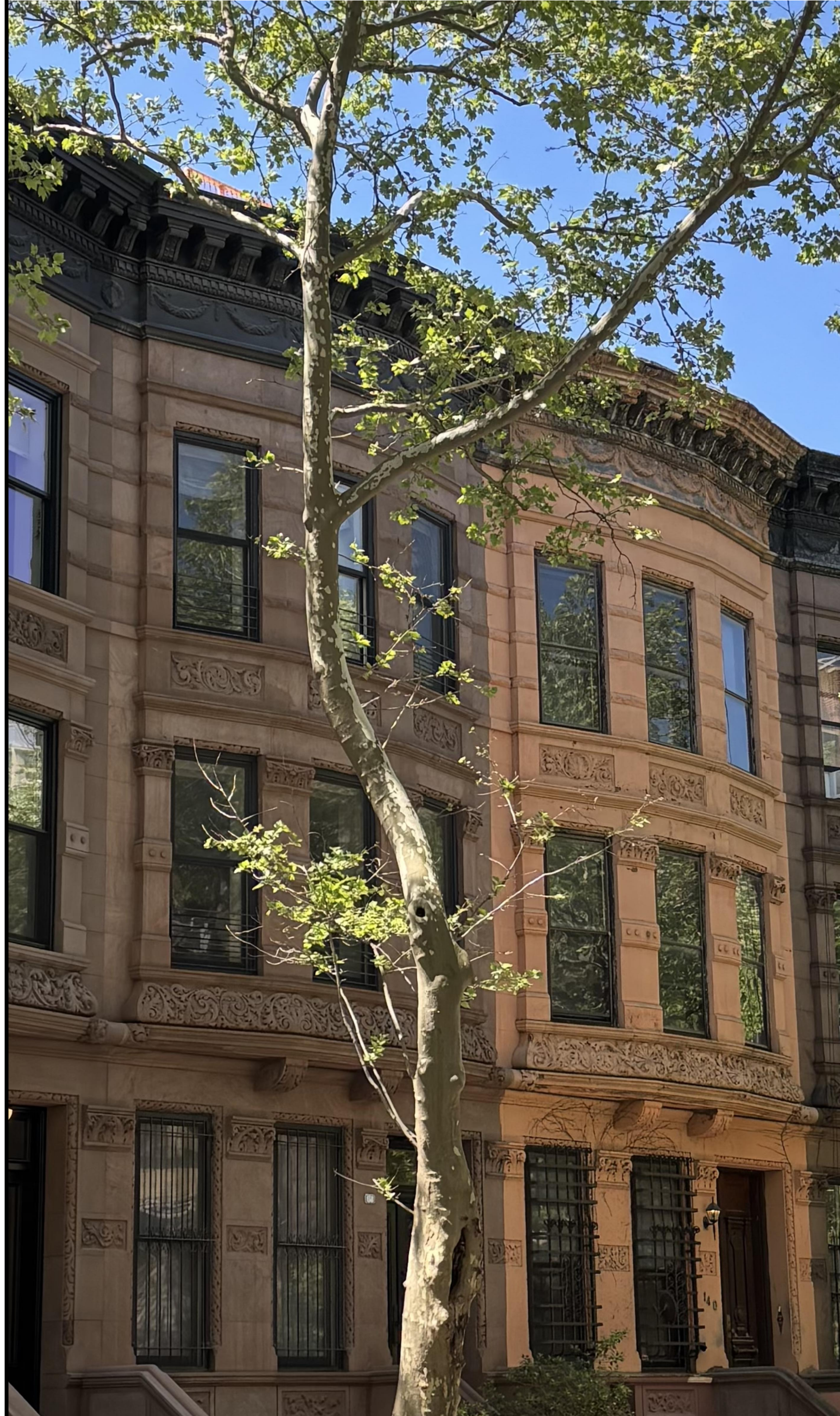
01 PICTURE 1 - MINOR VISIBILITY FROM THE STREET
