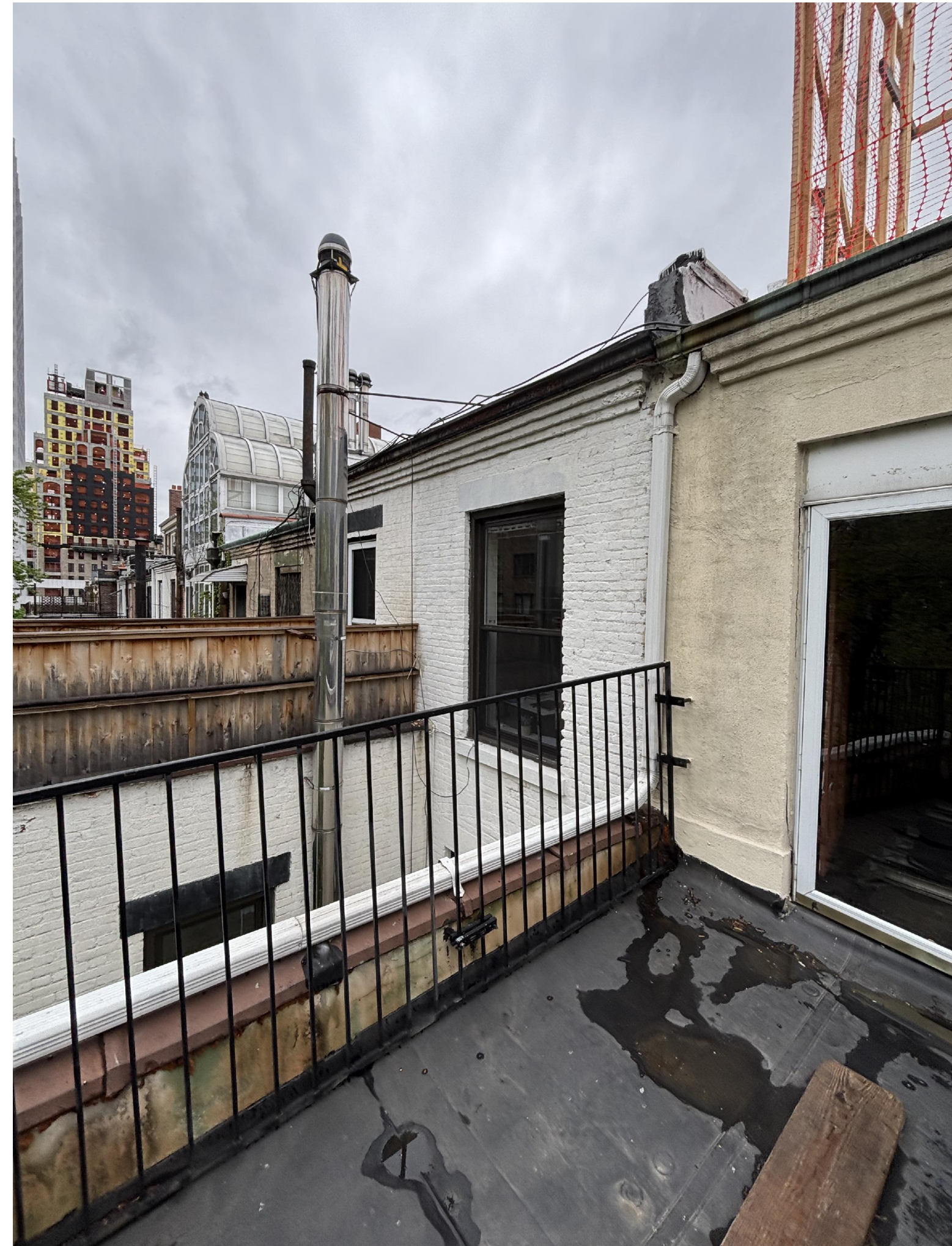
02 140W 88TH STREET - EXISTING 3RD FLOOR REAR FACADE NEIGHBORS SCALE: N.T.S.
