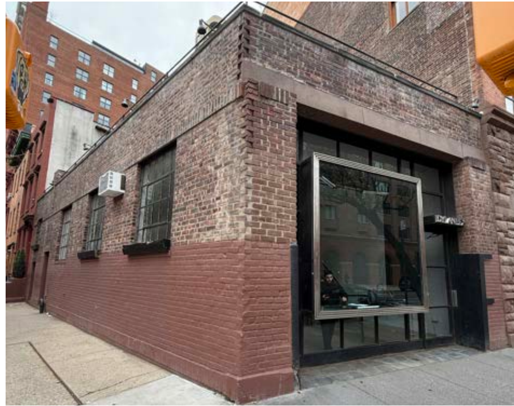
CURRENT BUILDING PHOTO - 2025
