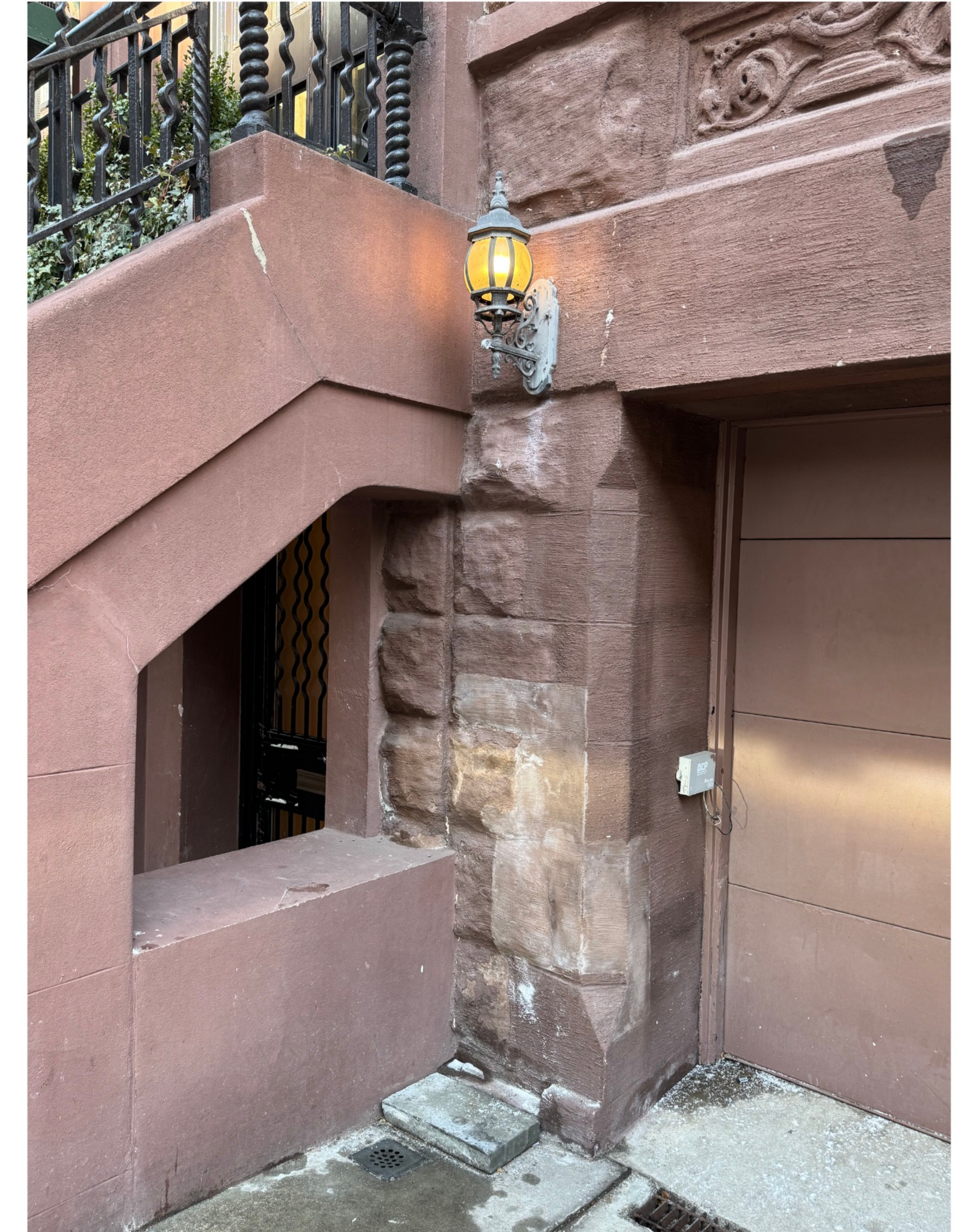
ALL SURFACES ARE STUCCO (NO ORIGINAL BROWNSTONE)
