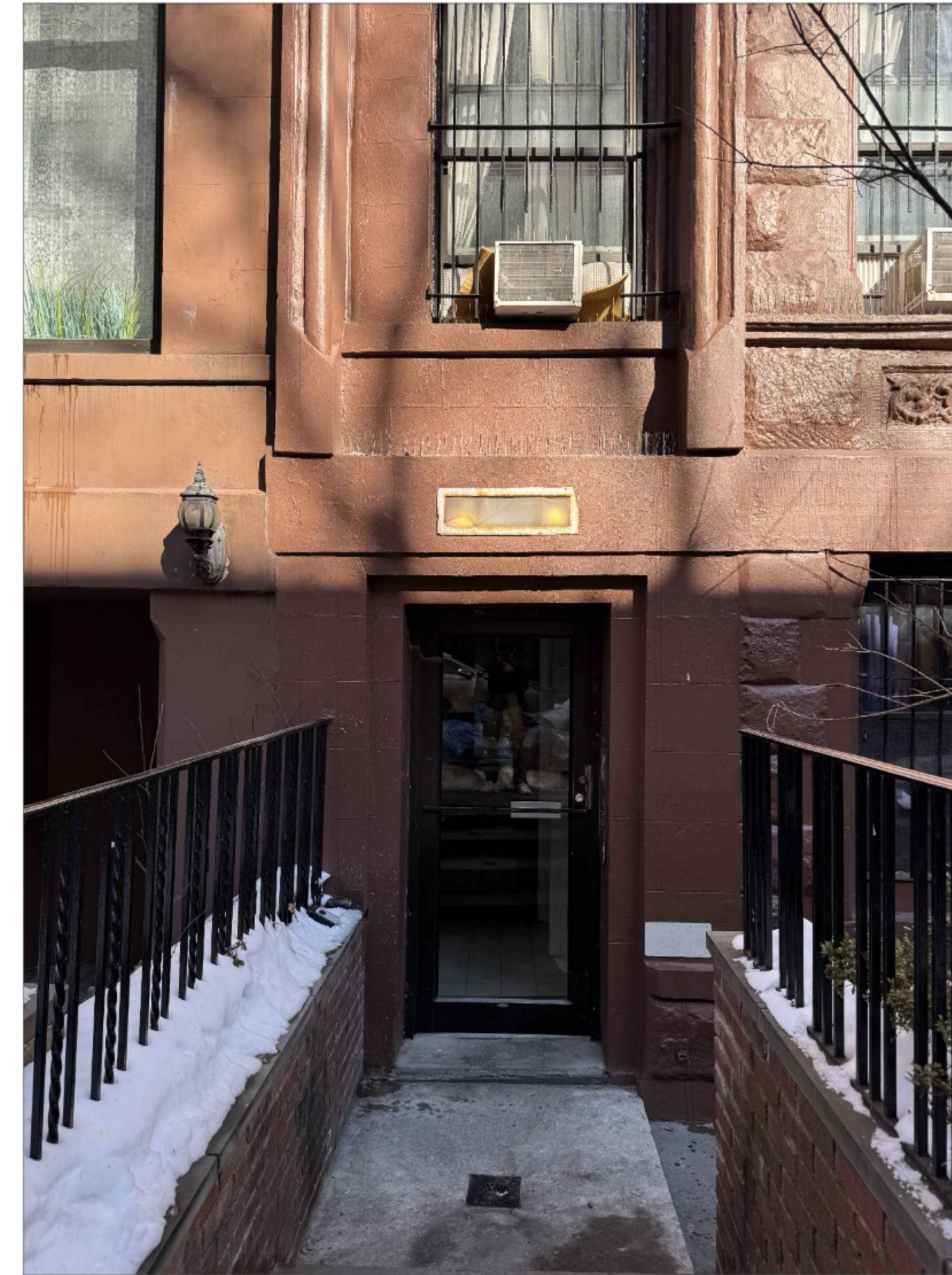
EXISTING CONCRETE RETAINING WALL & RAILING RETURN @ 57 W 90TH ST MKCA RECORDS 40
