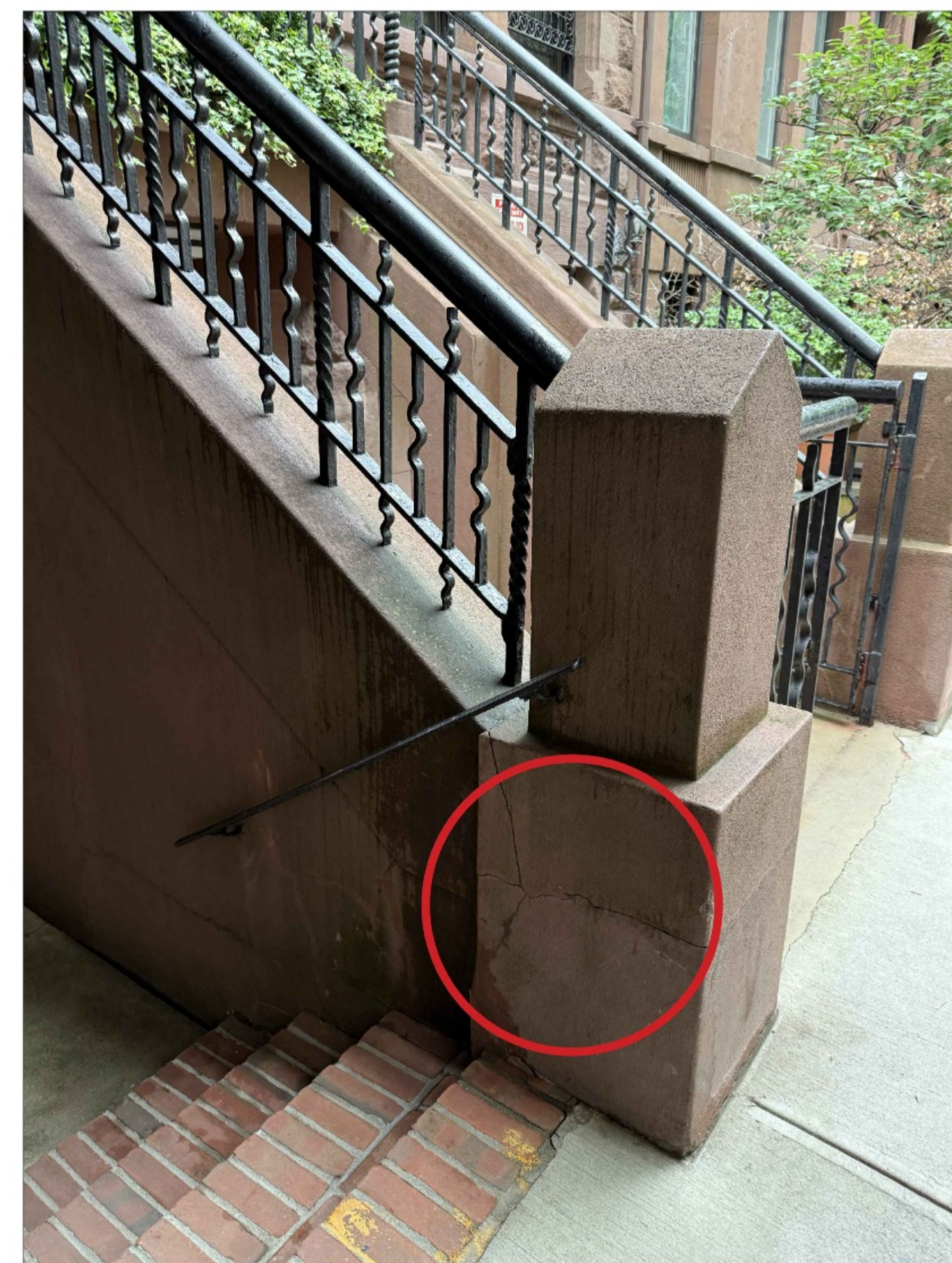
CRACKS & DISCOLORATION ON NEWELS MKCA RECORDS 20
