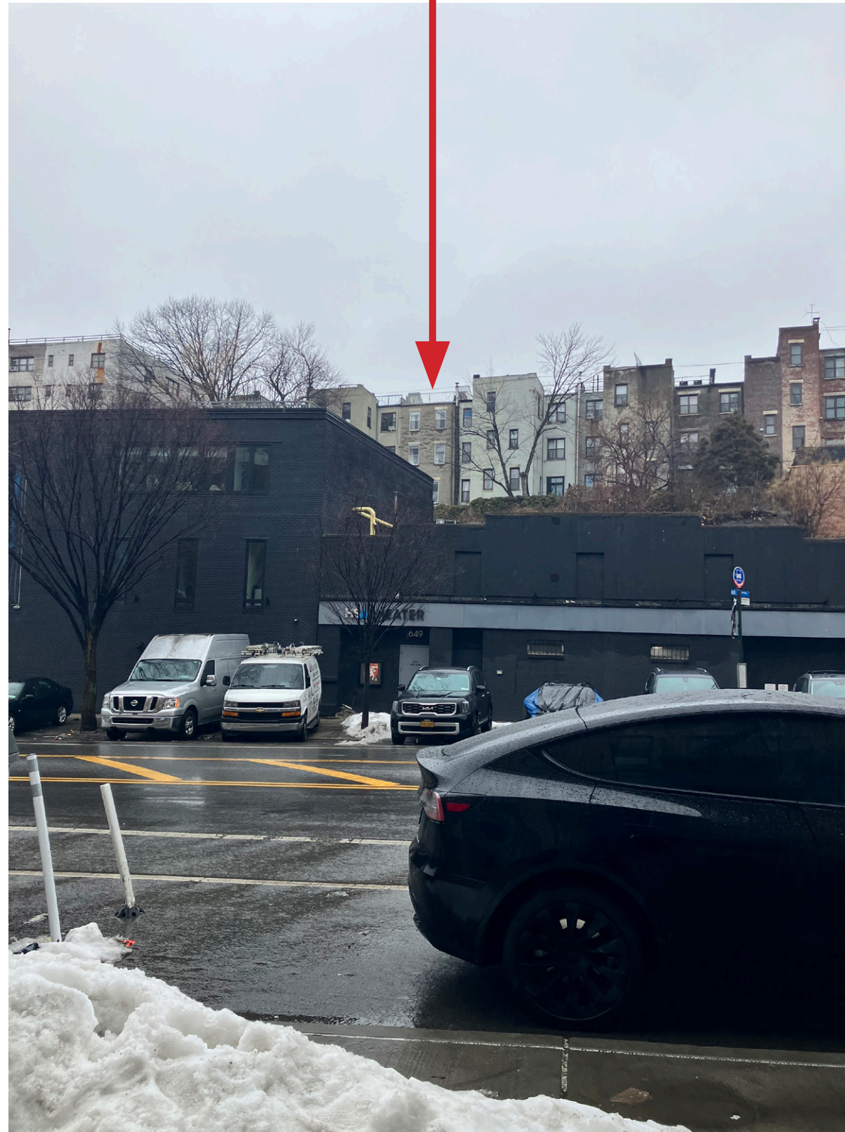
EXISTING REAR FACADE
