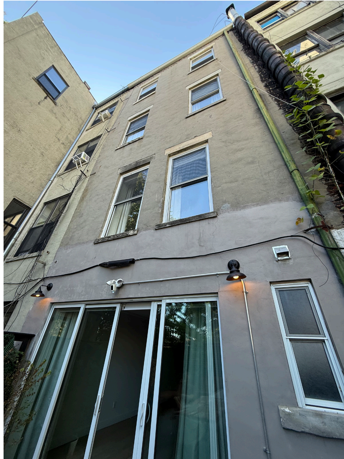
EXISTING REAR FACADE
