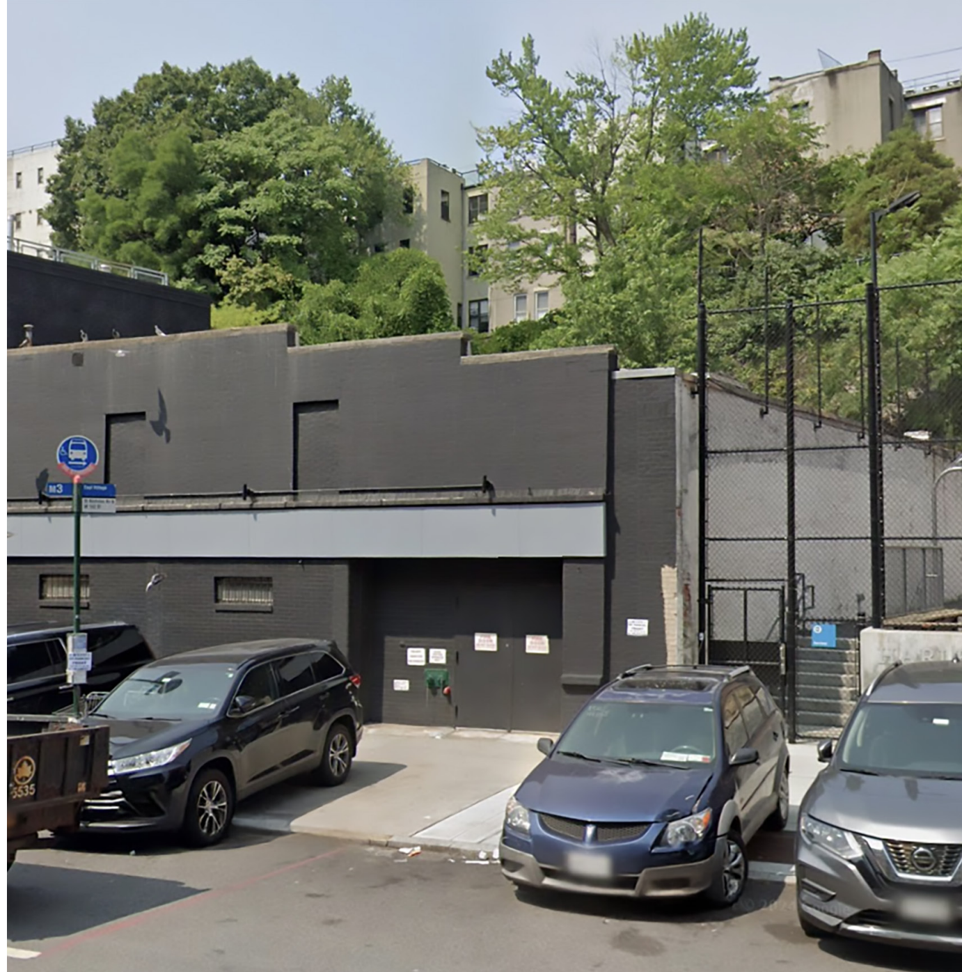
EXISTING REAR FACADE
