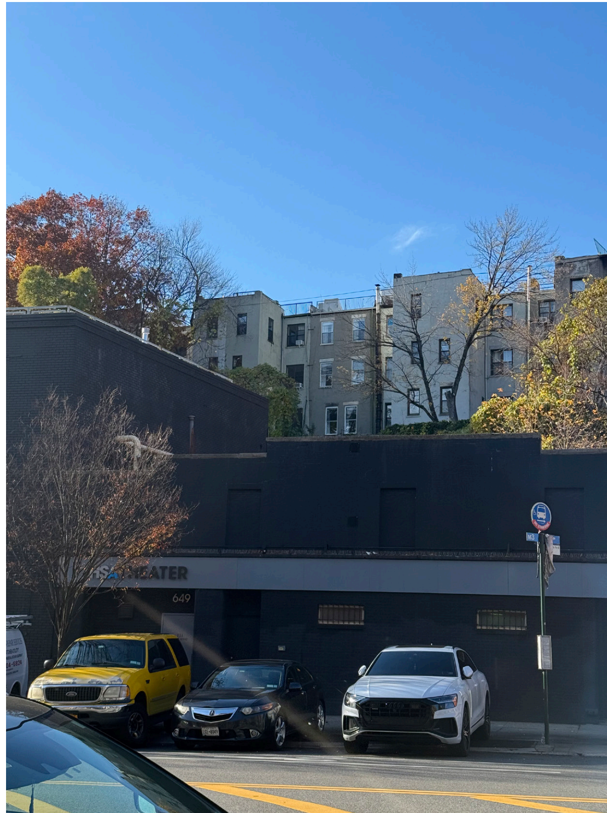
EXISTING REAR FACADE
