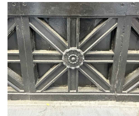
EXISTING METAL GRILLE
