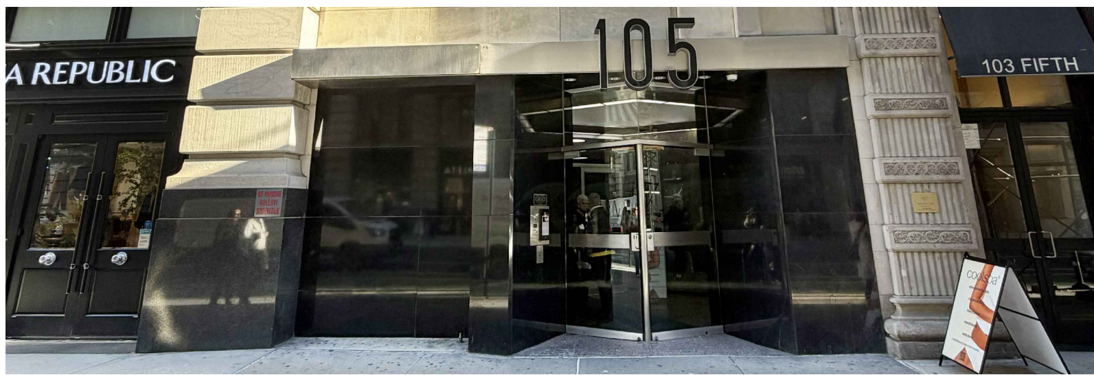
CURRENT FACADE - 5TH AVENUE
