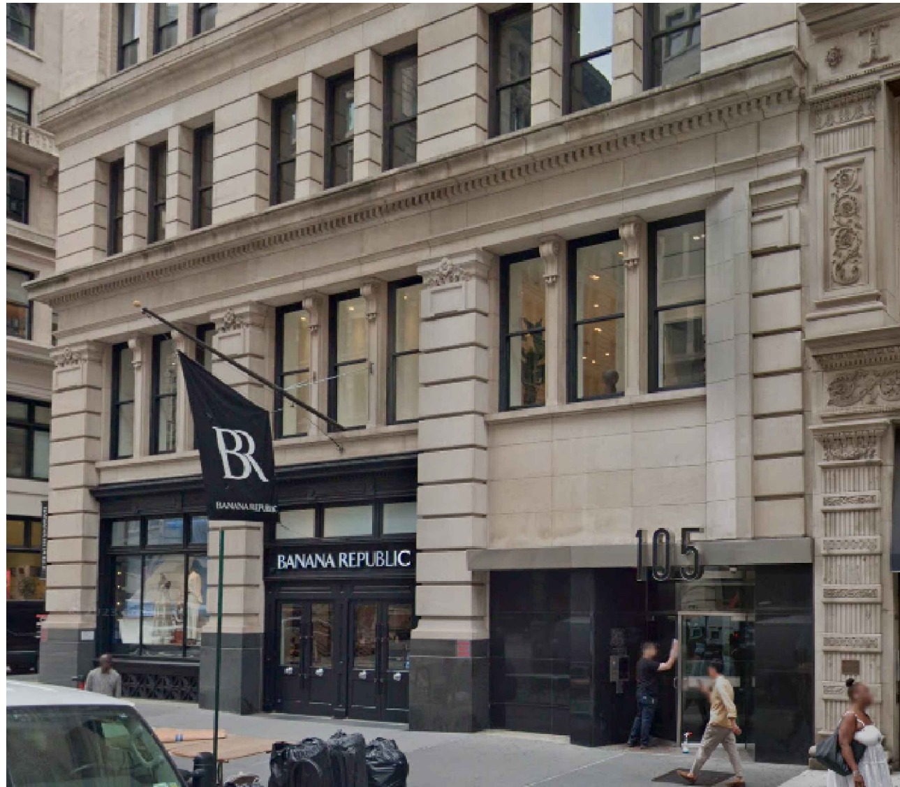
CURRENT FACADE - 5TH AVENUE
