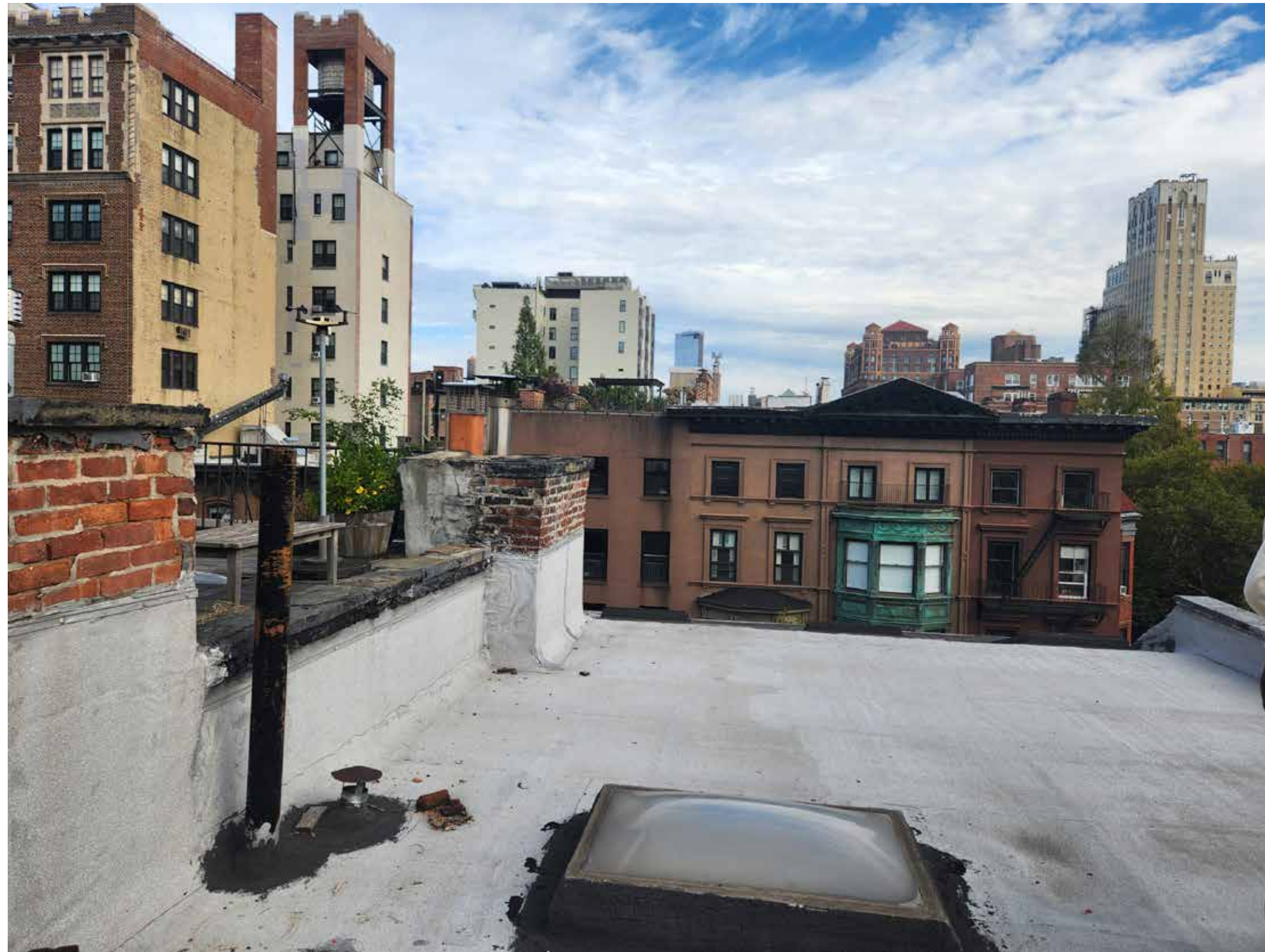
VIEW FROM ROOF LOOKING NORTH
