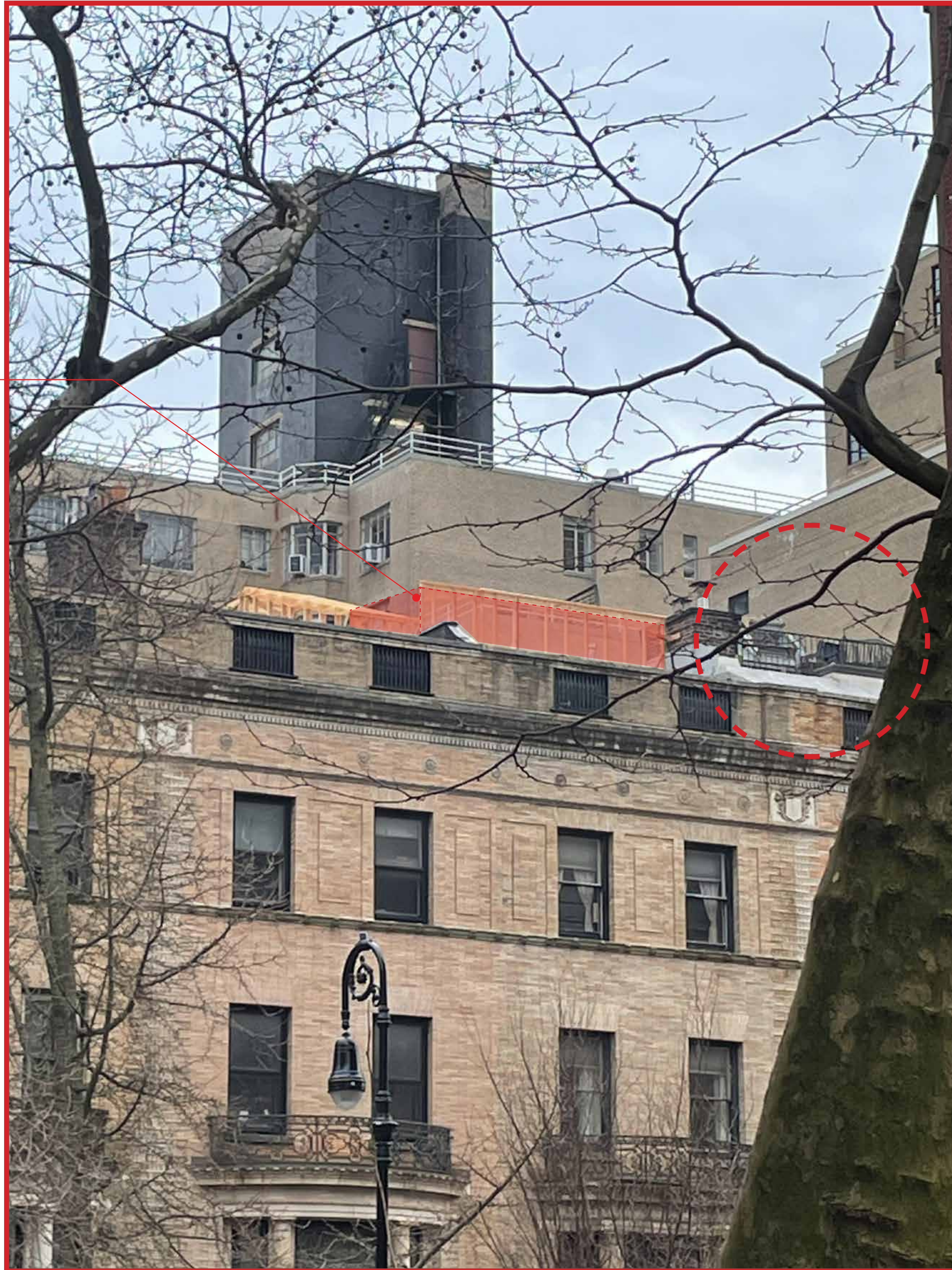
CLOSE-UP VIEW OF 8 PIERREPONT ST'S ROOF BULKHEAD FROM WILLOW STREET
