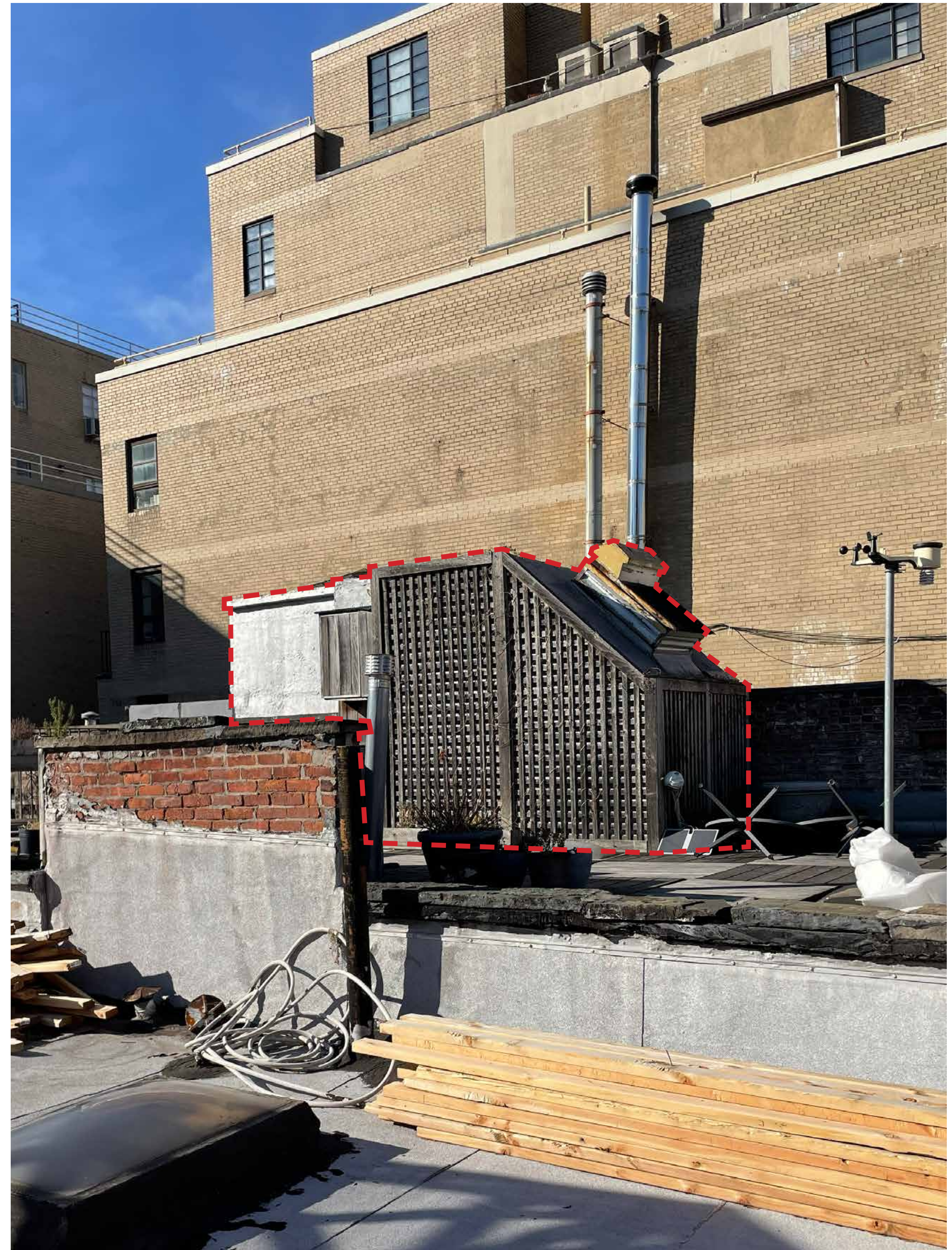
VIEW OF 8 PIERREPONT ST'S BULKHEAD FROM 10 PIERREPONT ST'S ROOF
