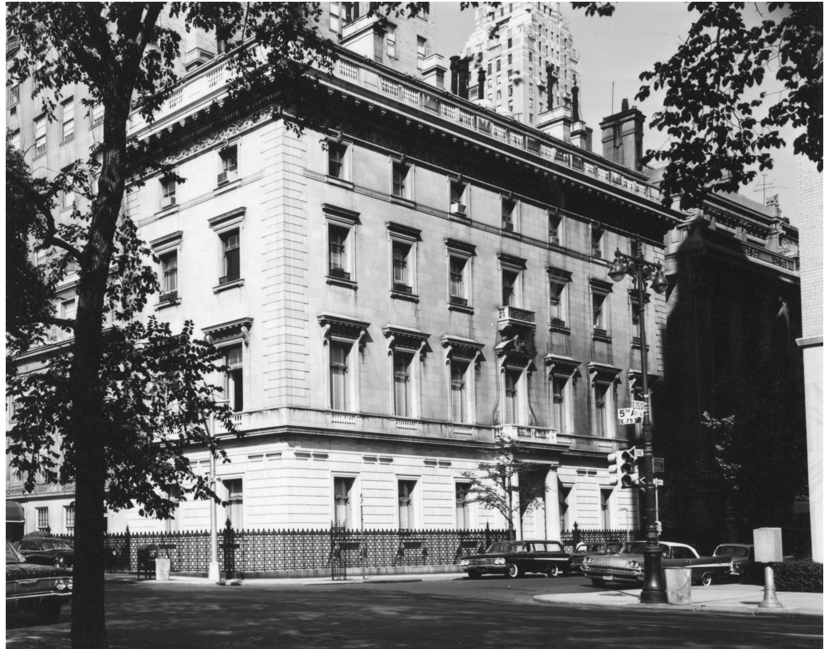
CORNER OF 5TH AVE AND 75TH STREET ca 1967 (LPC DESIGNATION PHOTO)
