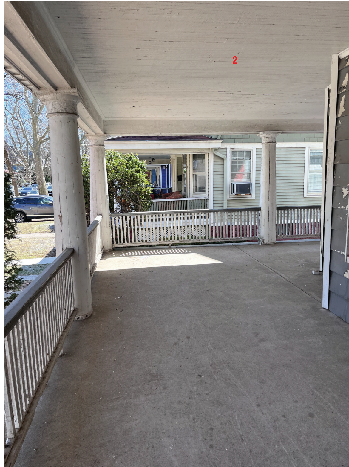
Existing porch ceiling: dropped beadboard
