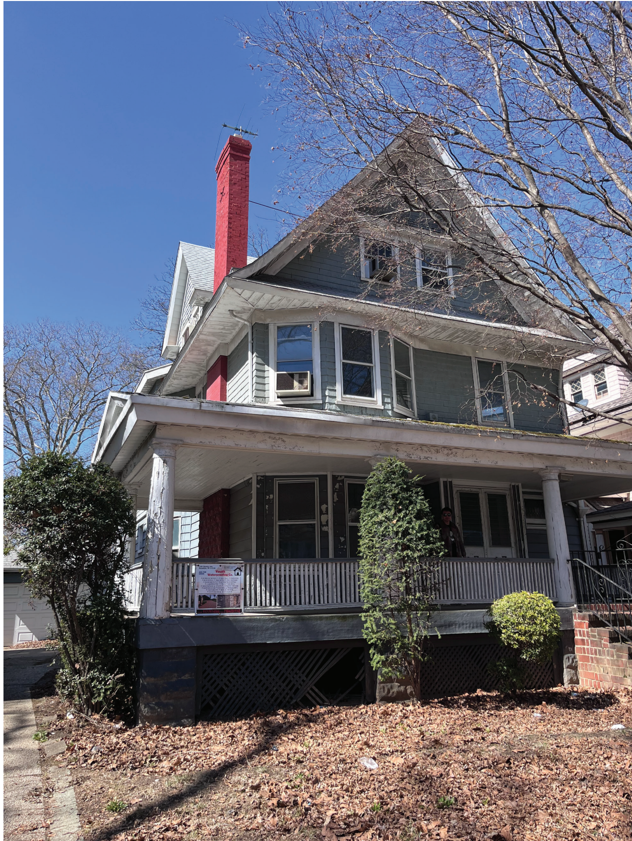
Existing Facade color: Dark Blue Gray 1st floor (lap siding) Light Blue Gray 2nd and 3rd floor (Shingle siding)
