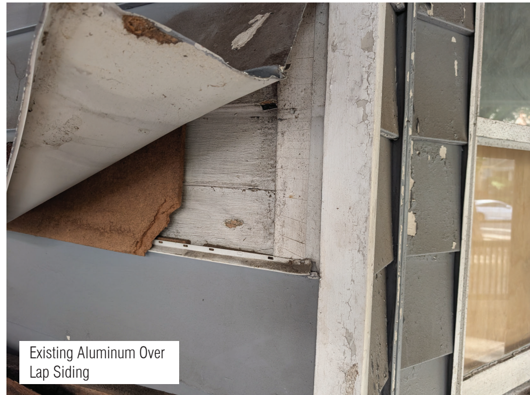
Existing Lap Siding and Wood Trim
