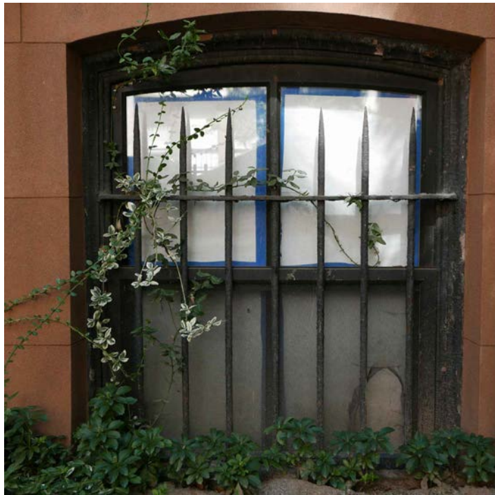
3 EXISTING FRONT FACADE BASEMENT WINDOW WITH EXISTING GRILLE AND BRICKMOLD
