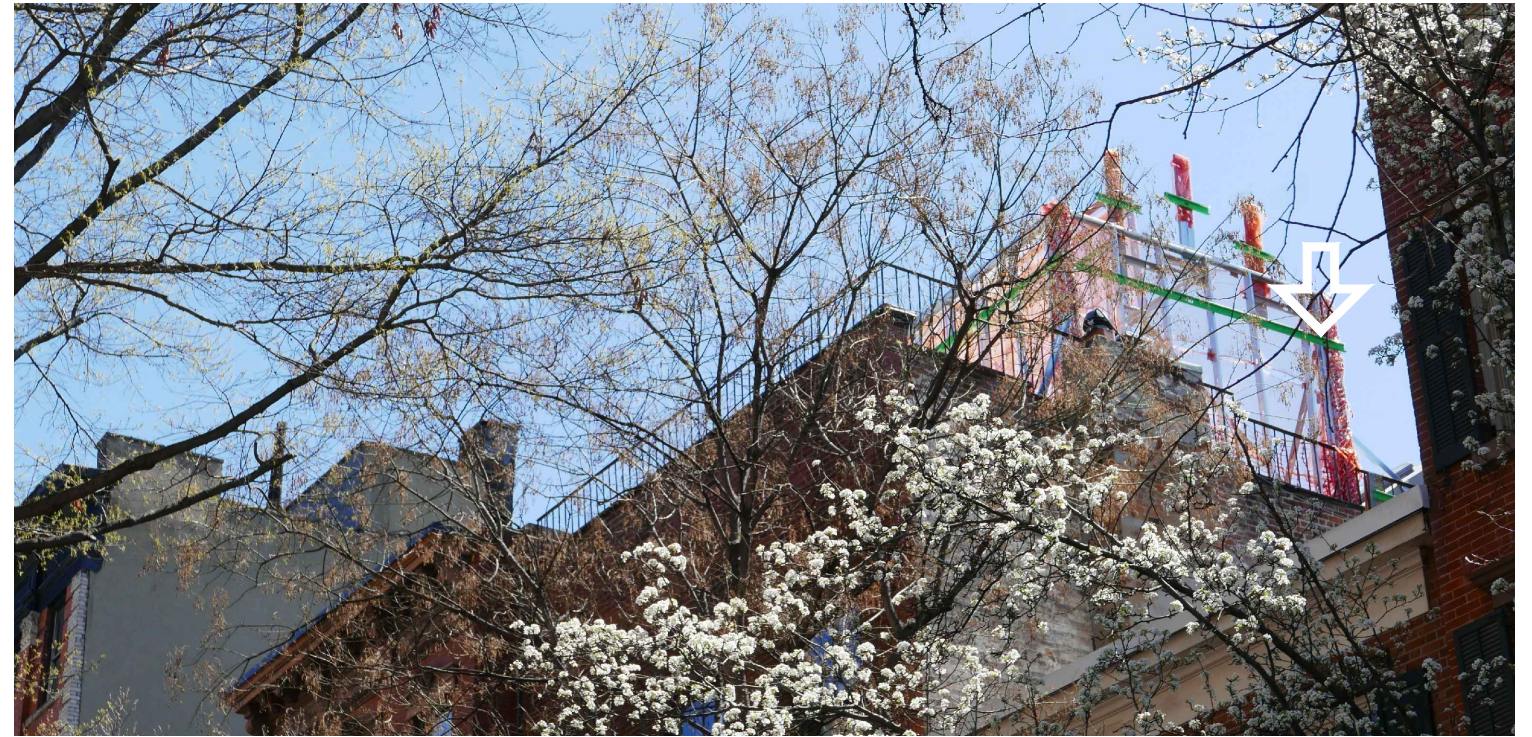
(C1) ENLARGED VIEW OVER 62 BANK ST OF 60 BANK ST ROOF ADDITION MOCK-UP, EXISTING NORTH RAILING REMOVED N/A
