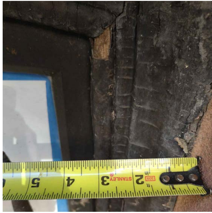
2 EXISTING BRICK MOLD DETAIL
