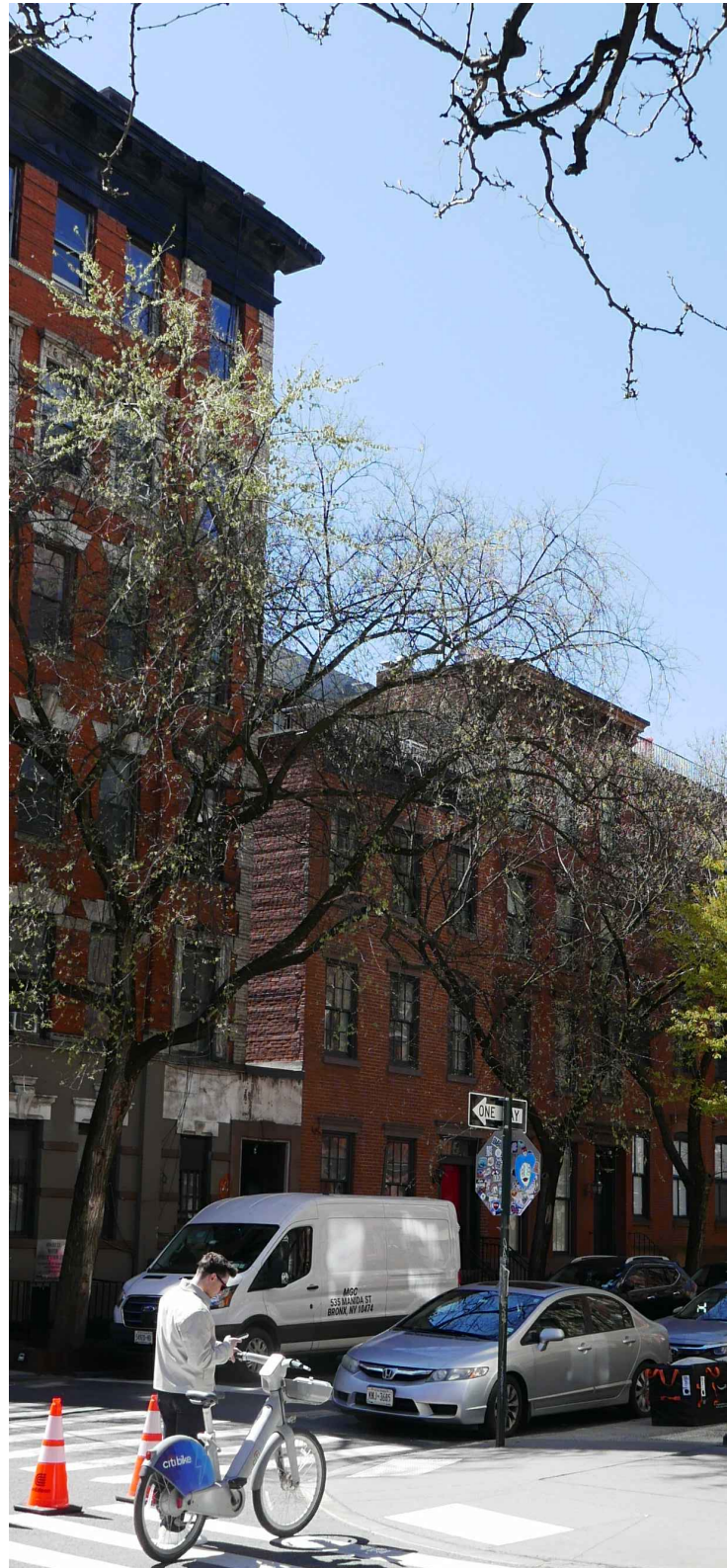
F VIEW SOUTHWEST TOWARD 60 BANK STREET OF ROOF ADDITION MOCK-UP TAKEN FROM BANK ST. AND W 4TH ST. N/A
