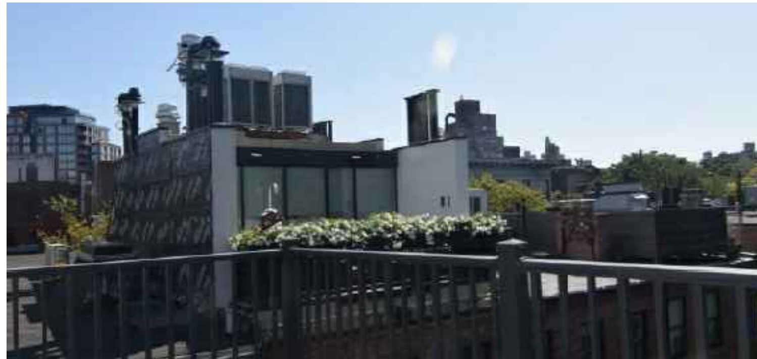
③ 292 W 4TH ST ROOF ADDITION IMAGE C/O 58 BANK ST LPC FILING
