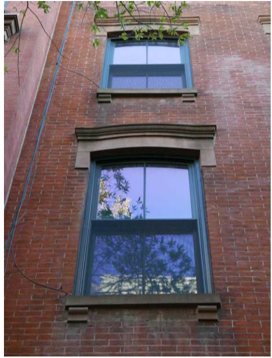
4 EXISTING 2ND AND 3RD FLOOR BRICKMOLD, TYPICAL
