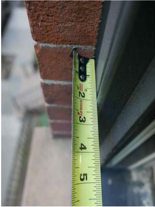
6 EXISTING 2ND AND 3RD FLOOR BRICKMOLD DEPTH
