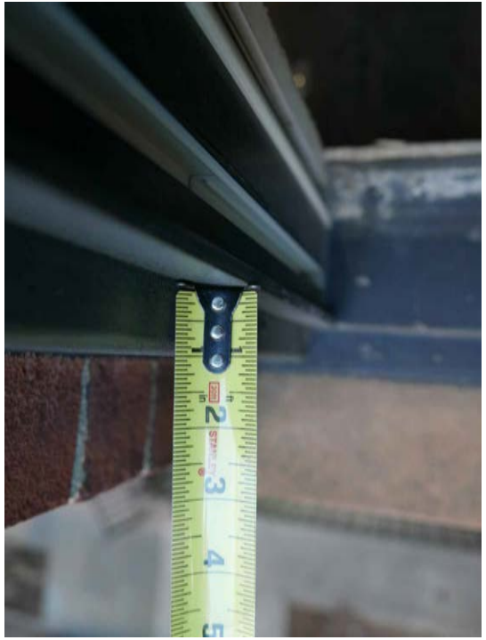
5 EXISTING 2ND AND 3RD FLOOR BRICKMOLD WIDTH
