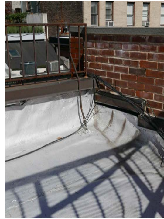
3 NORTHERN FACADE METAL COPING MEETING 58 BANK STREET
