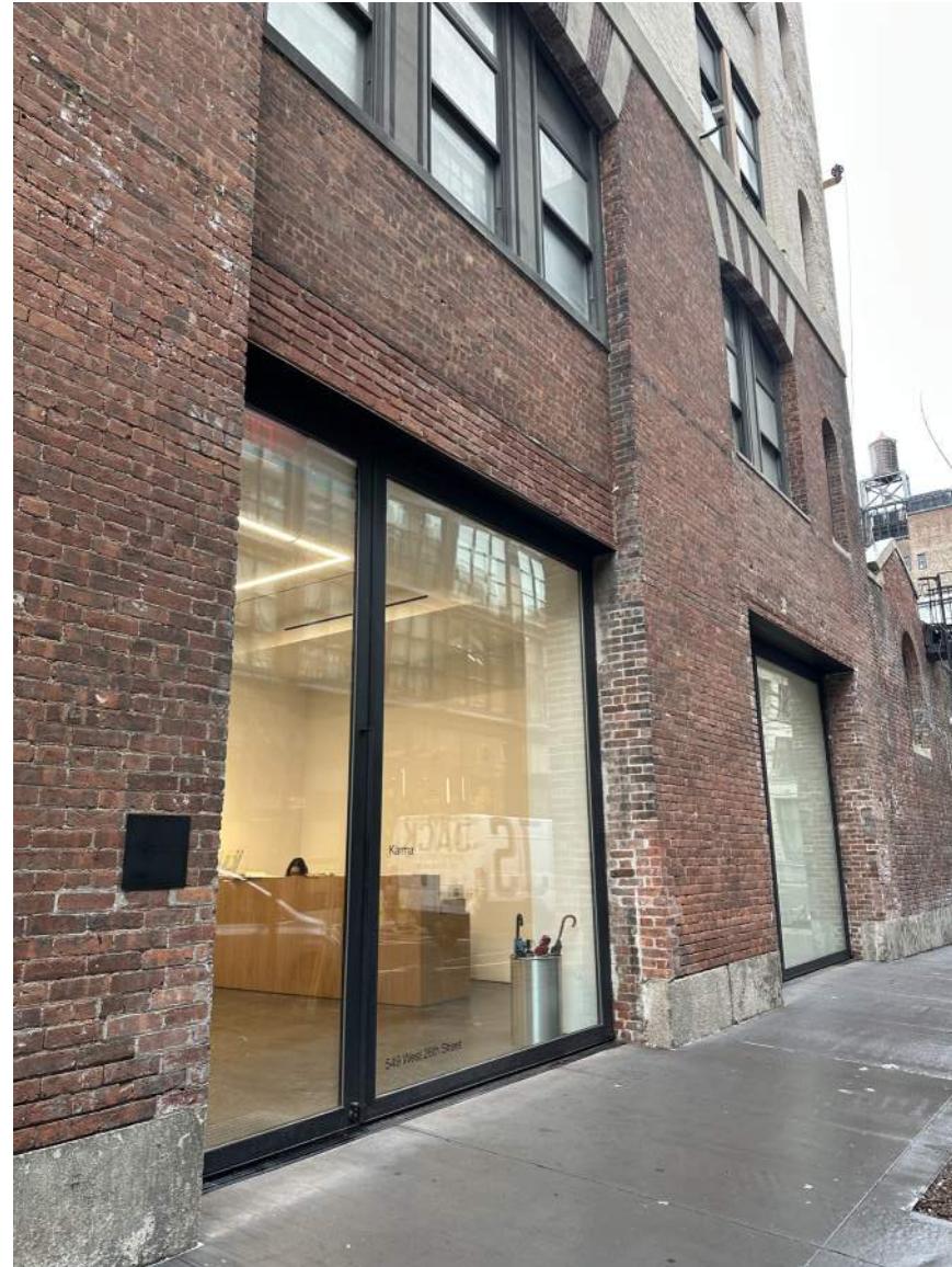
CURRENT CENTER DOOR AT SOUTH FACADE
