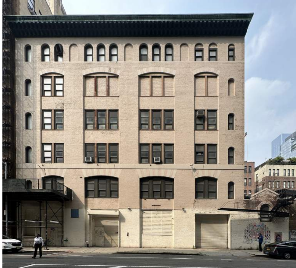
EXISTING SOUTH FACADE
