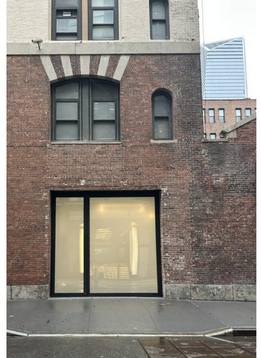
CURRENT EASTERN DOOR AT SOUTH FACADE
