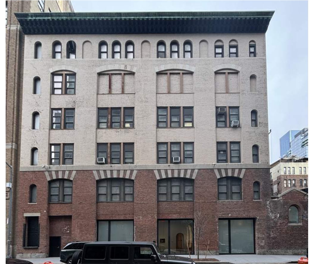
CURRENT SOUTH FACADE
