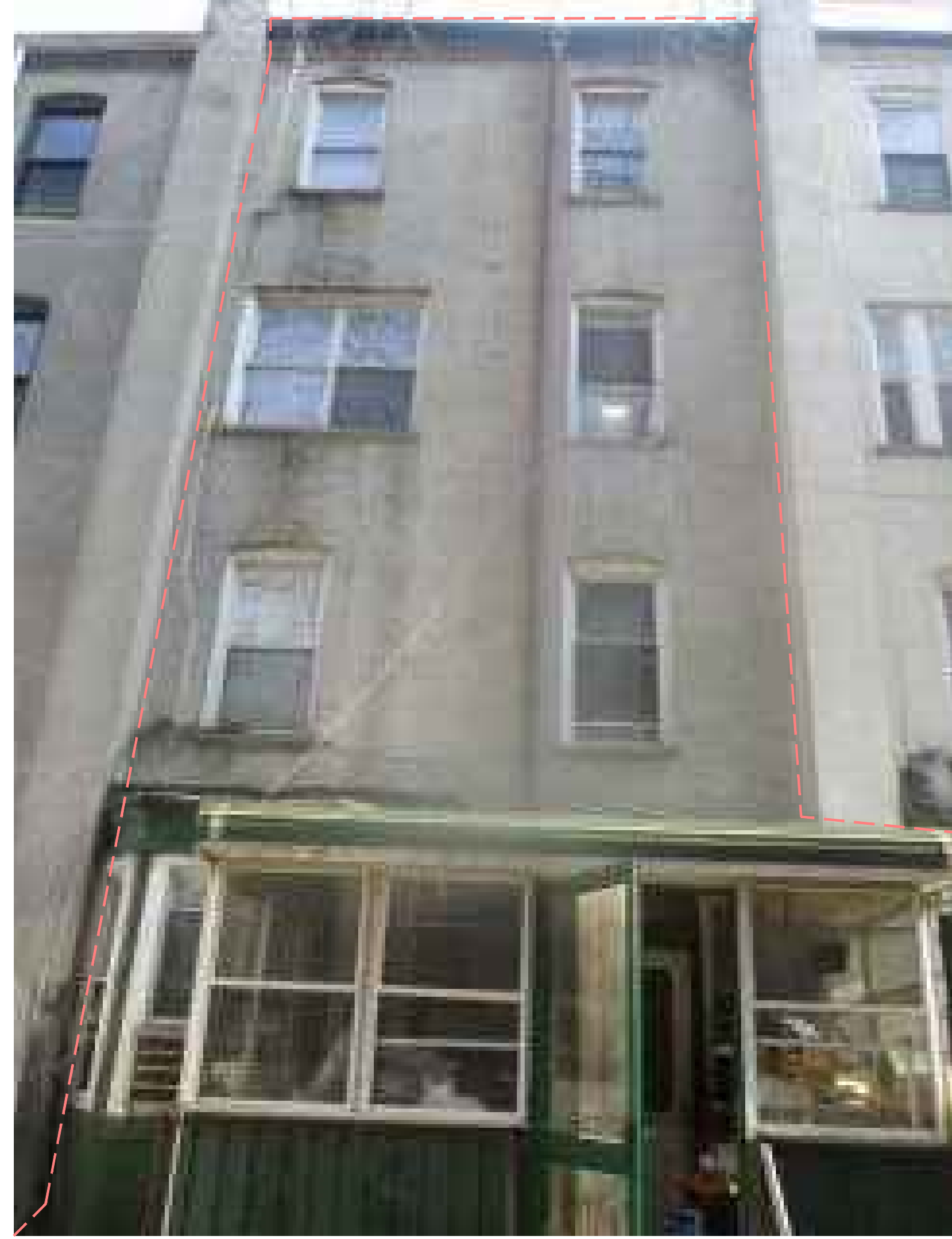
2 REAR VIEW PRIOR TO DEMOLITION
