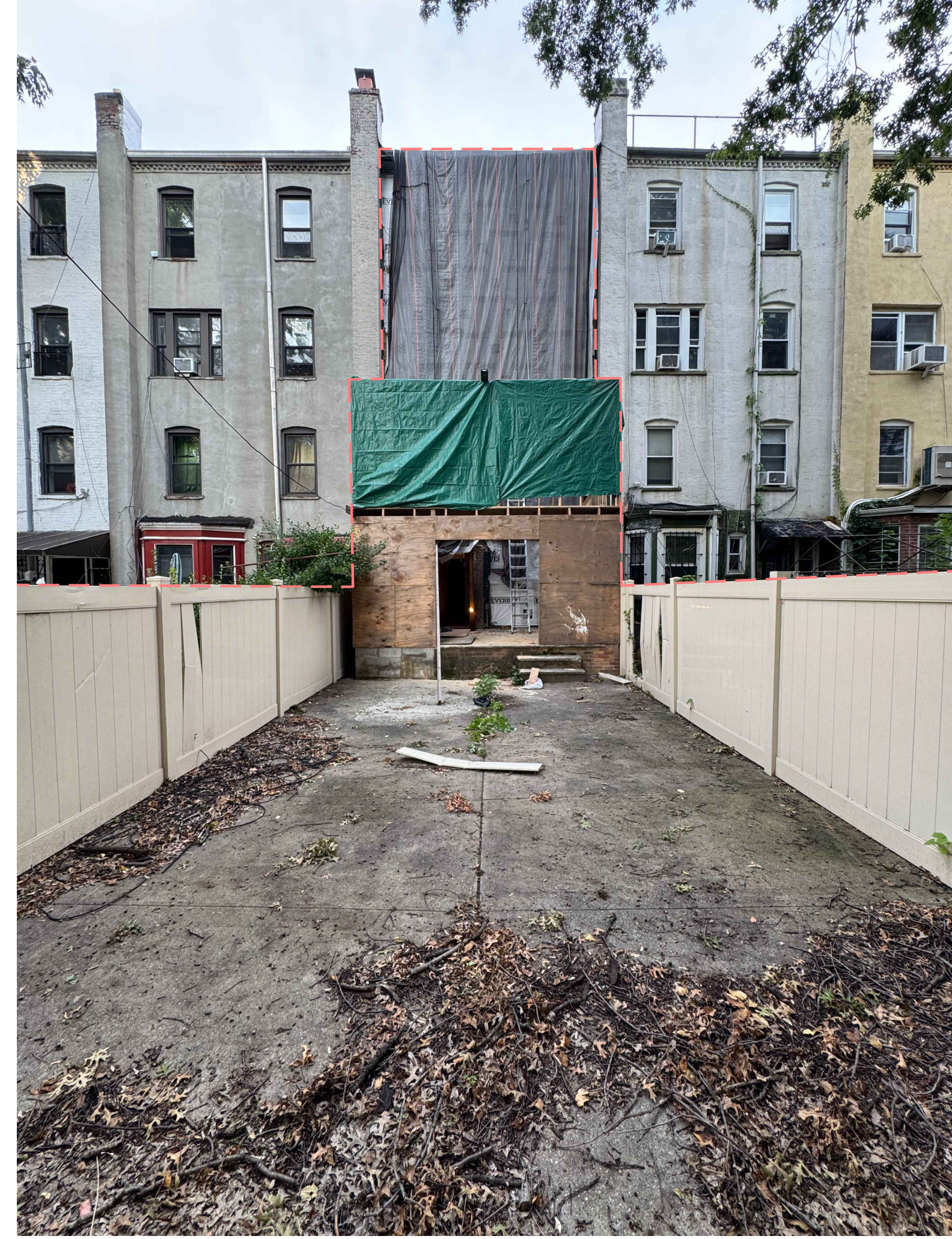
3 REAR VIEW WITHIN REAR YARD
