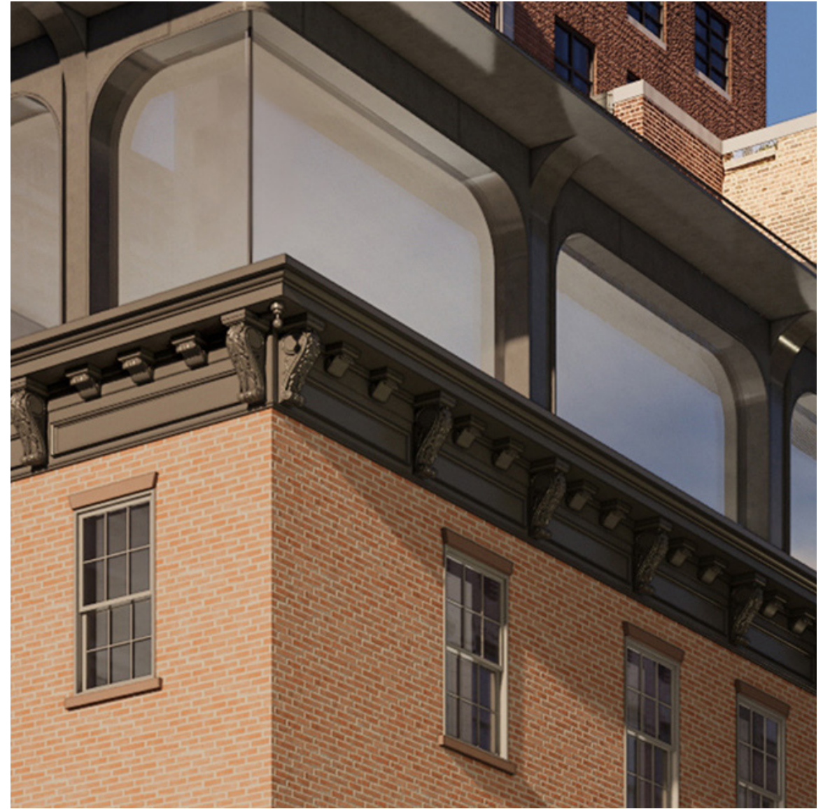
PROPOSED CORNICE RESTORATION AT 385 GREENWICH
