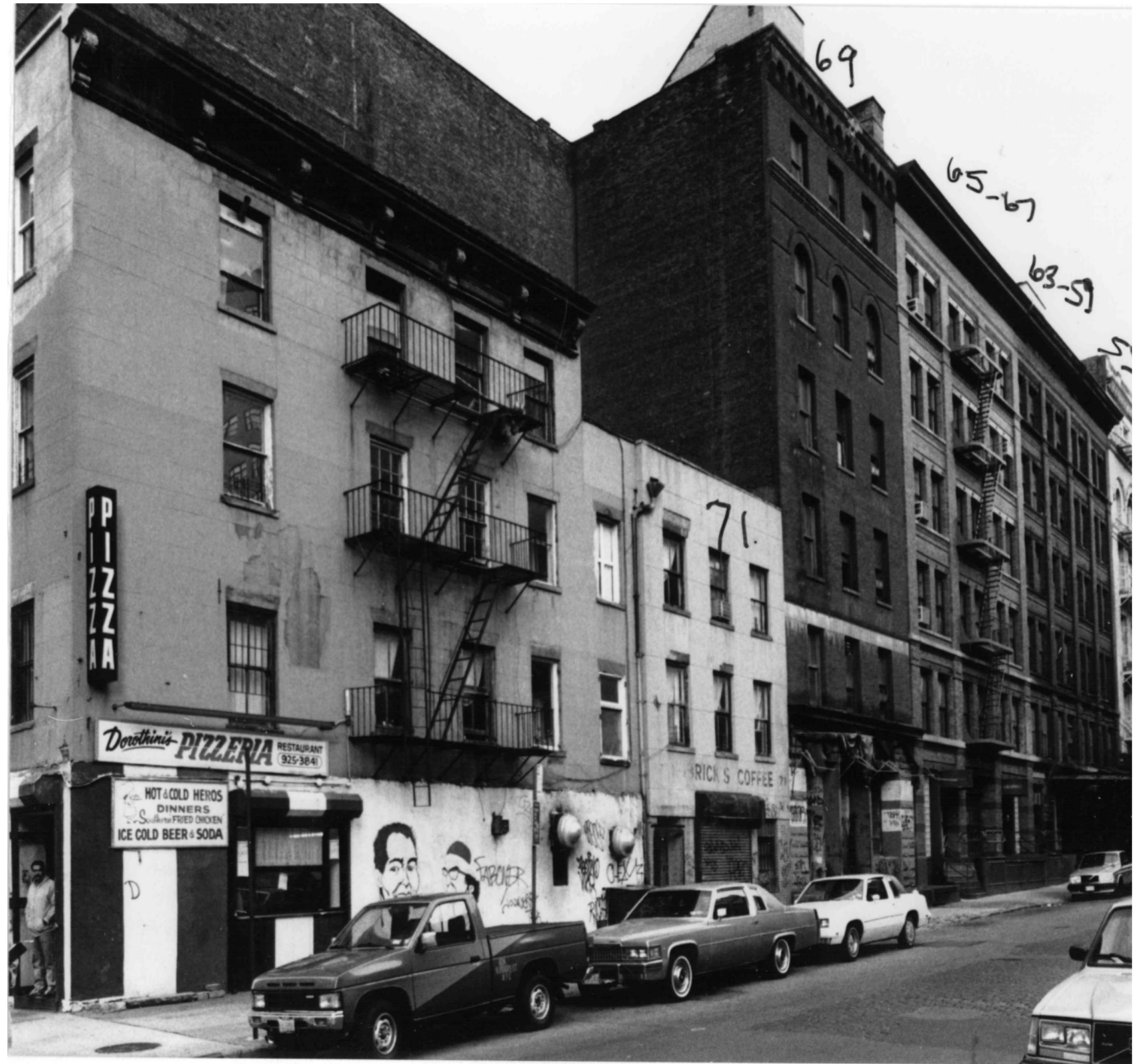
1991 (LPC Designation Photo)
