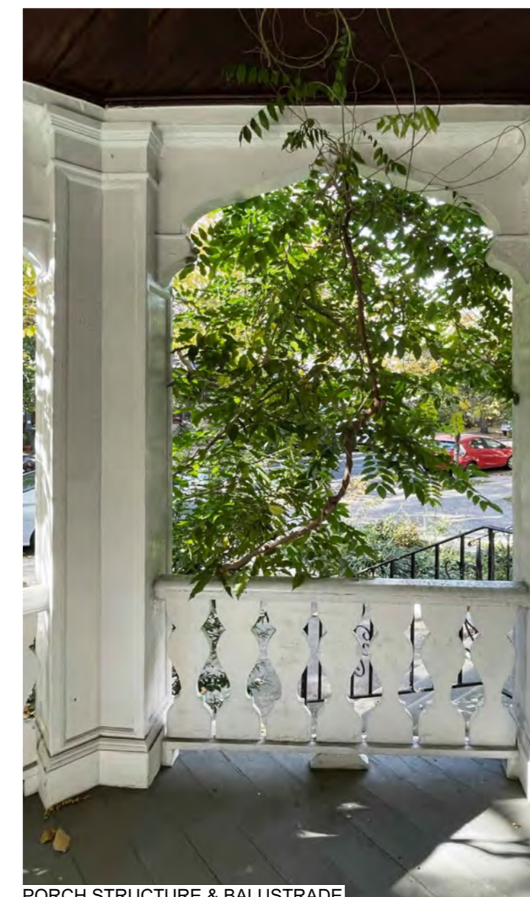
PORCH STRUCTURE & BALUSTRADE
