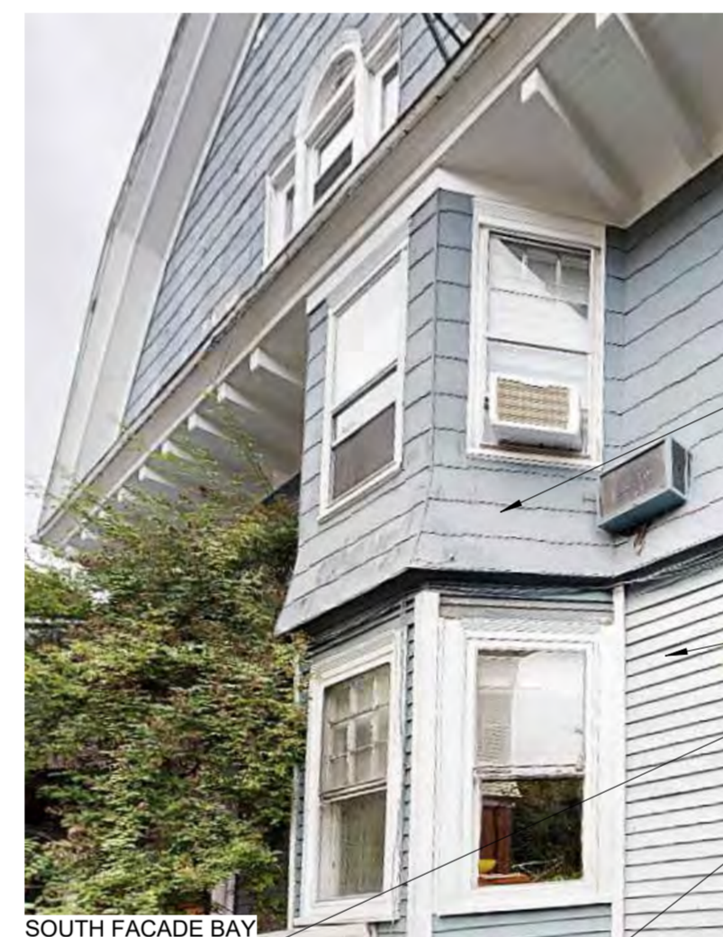
SOUTH FACADE BAY
