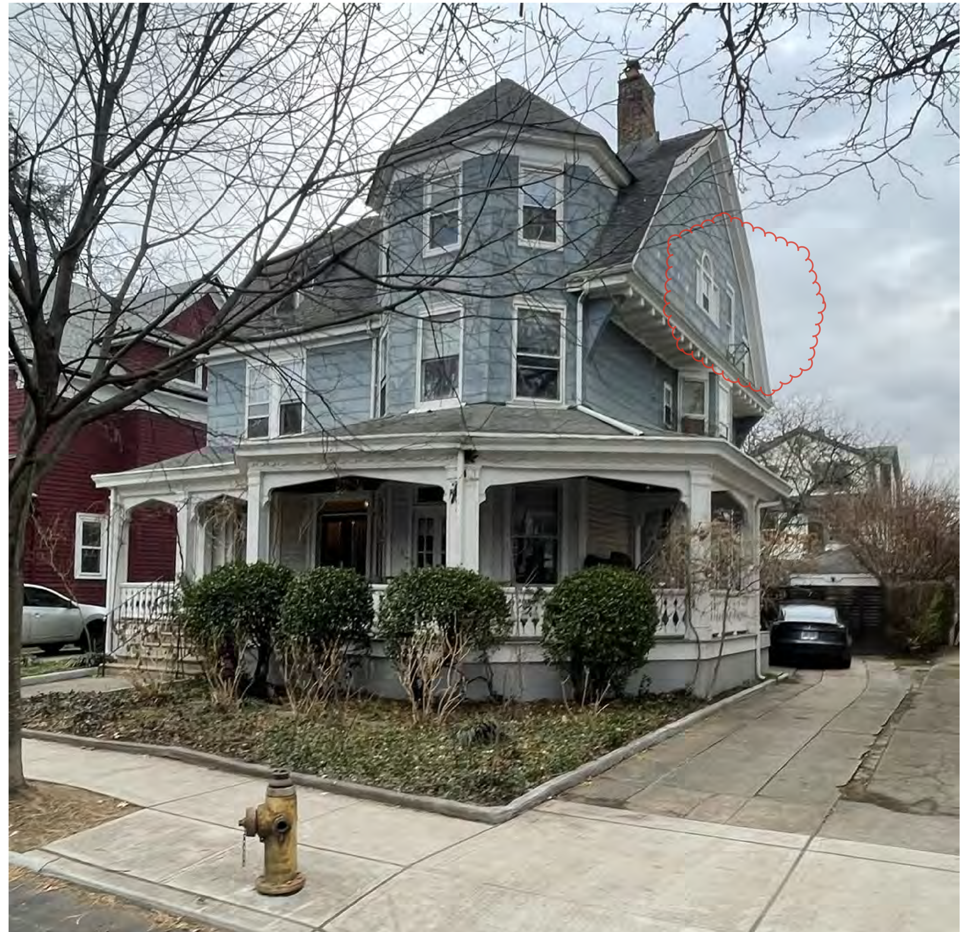
SIDE VIEW - SOUTH FACADE
