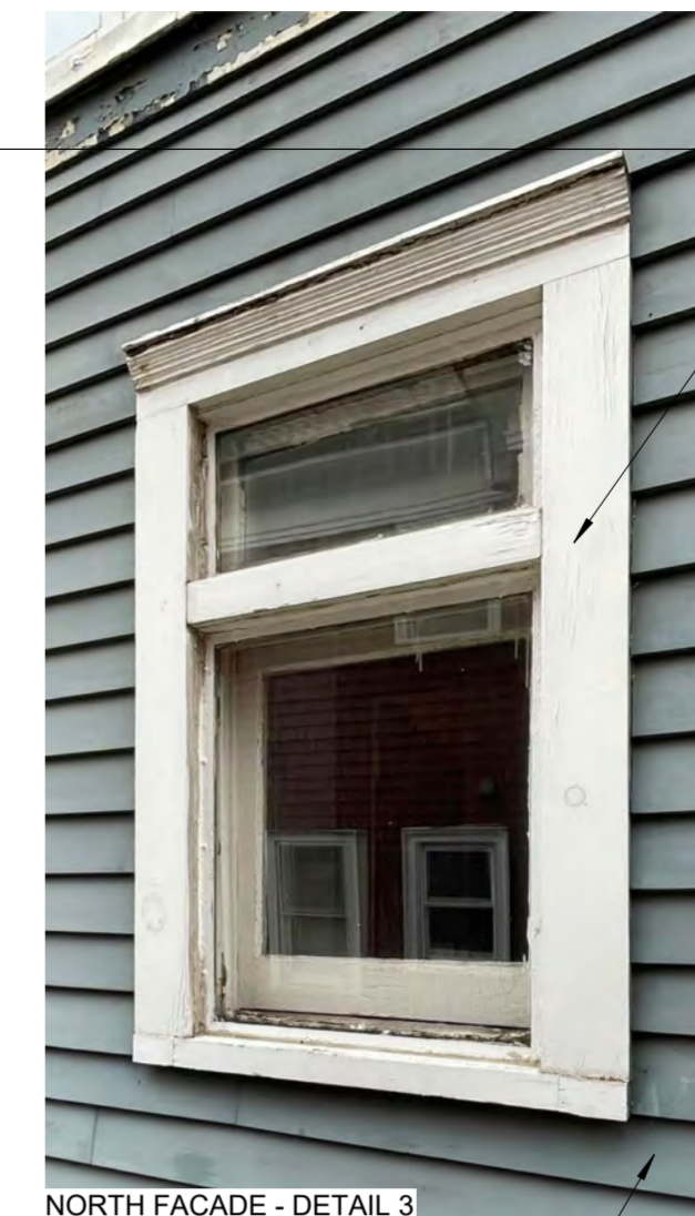
NORTH FACADE - DETAIL 3
