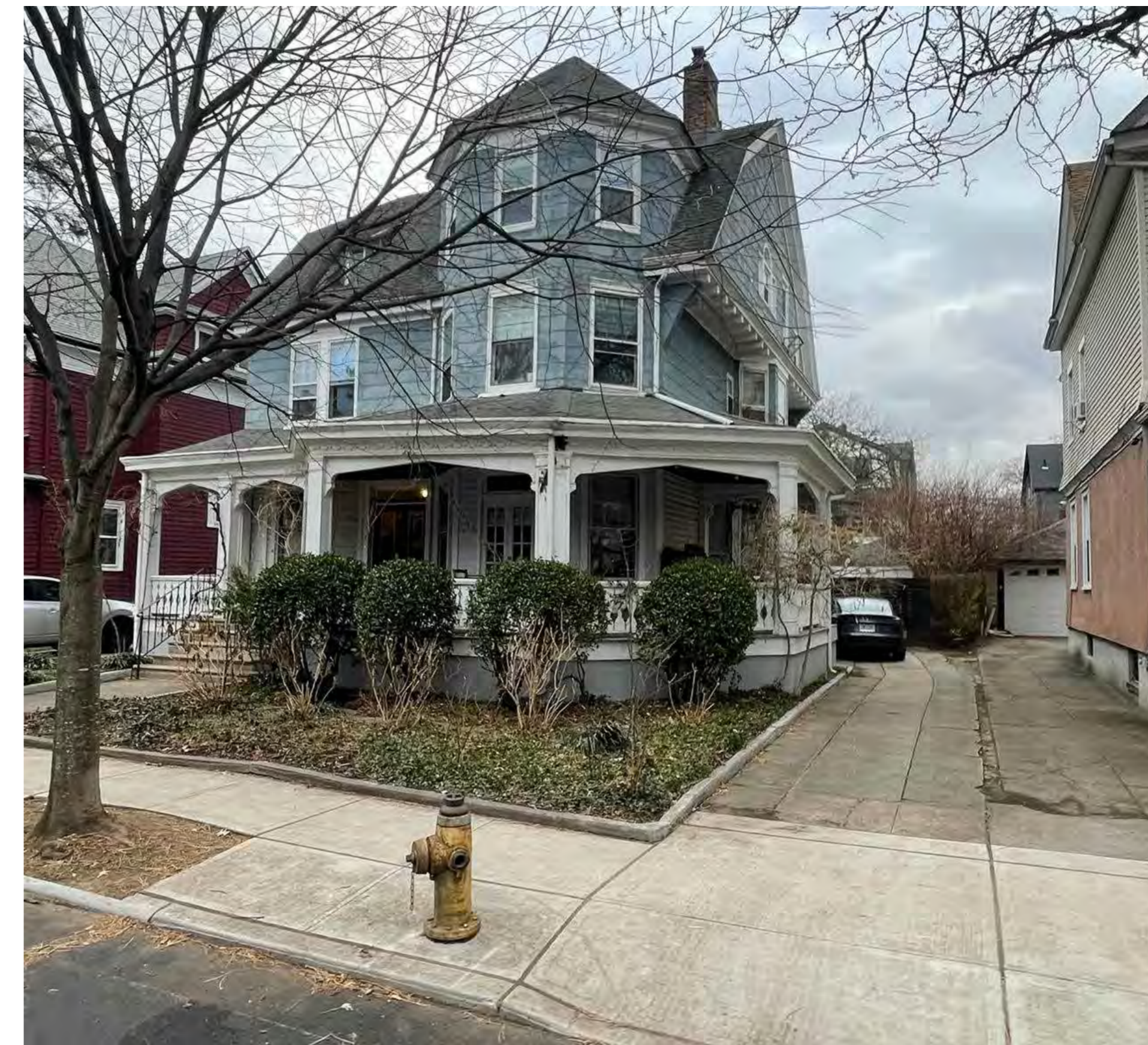
DRIVEWAY AND GARAGE: EXISTING CONDITIONS
