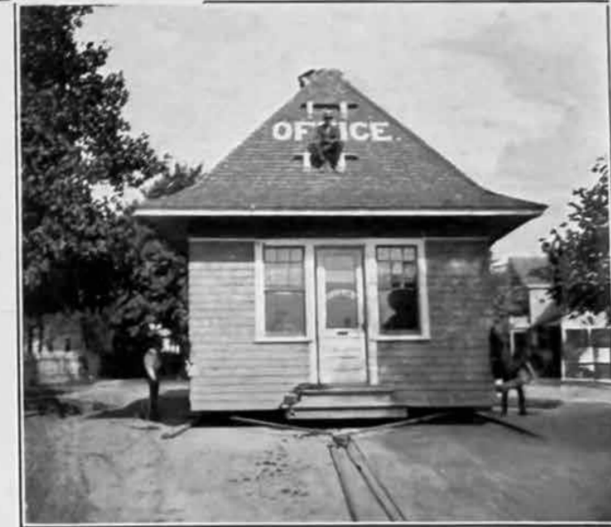
East 19th Street and Avenue C looking North. This picture was also taken in 1899. The little office to the right was made twice the size in 1900, and in 1901 moved from 19th Street to 15th Street in Beverley Square West.
