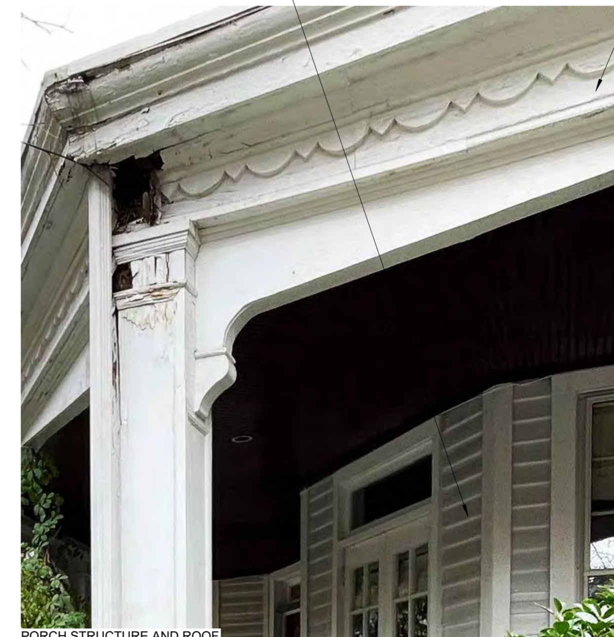
PORCH STRUCTURE AND ROOF
