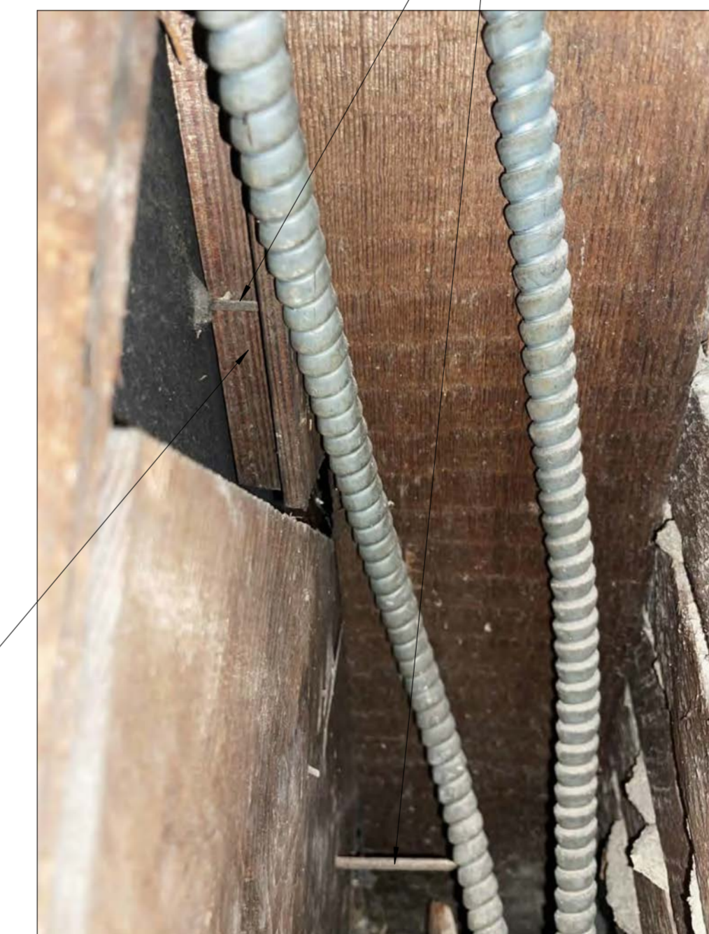
FLAT CUT NAIL FROM ORIGINAL CONSTRUCTION VS NEWER STYLE NAIL USED DURING ALTERATION
