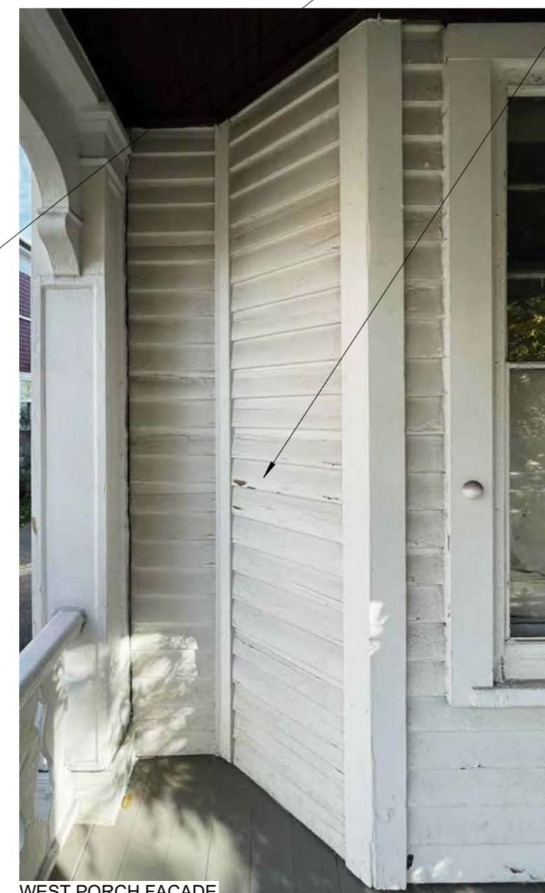
WEST PORCH FACADE
