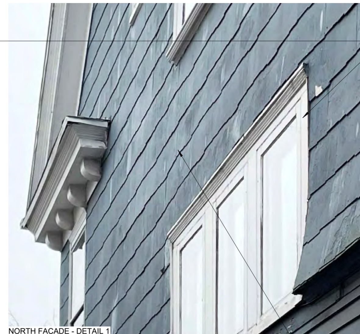
NORTH FACADE - DETAIL 1
