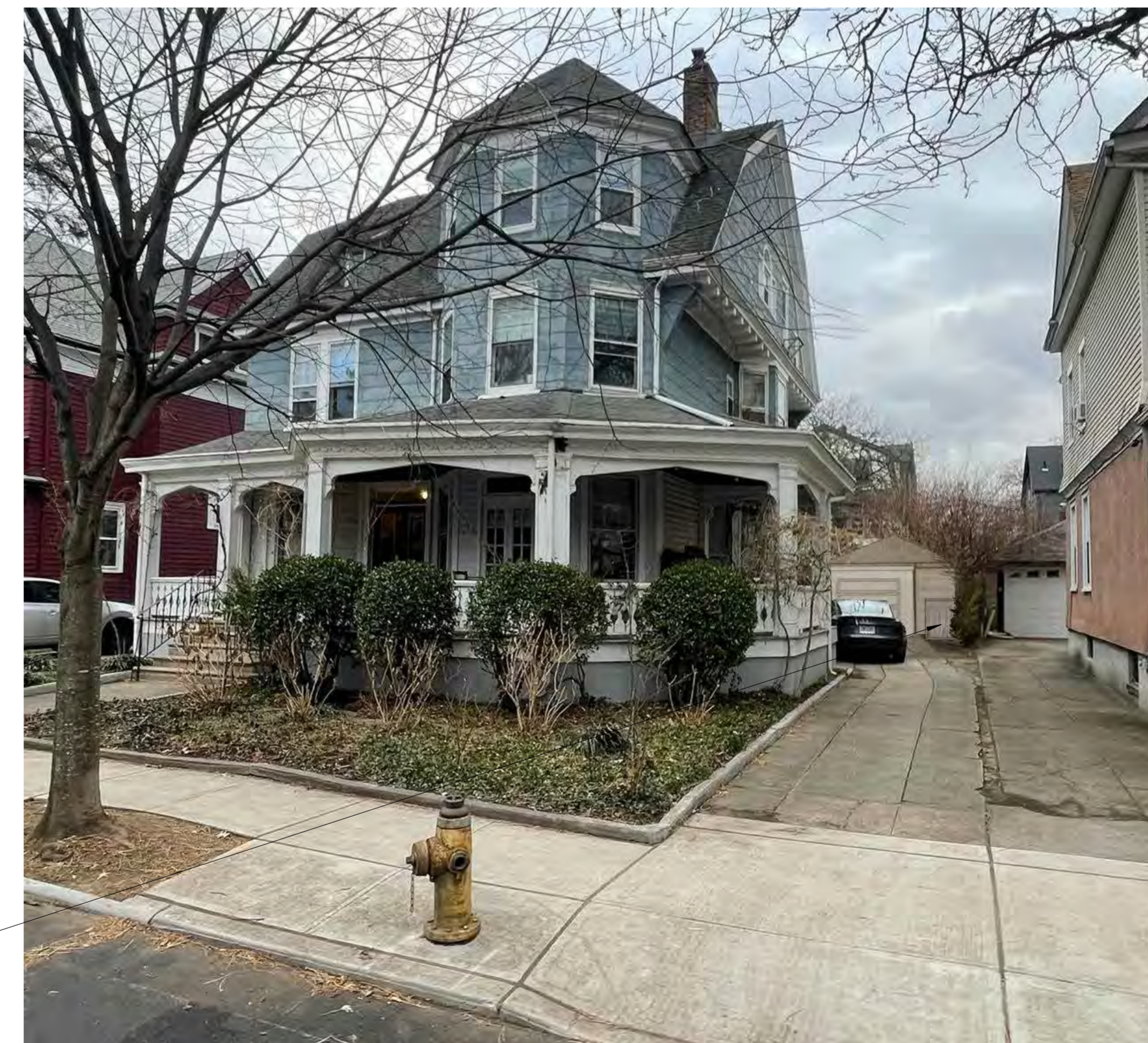
DRIVEWAY AND GARAGE: PROPOSED CONDITIONS (NO PROPOSED CHANGES TO GARAGE STRUCTURE OR FINISH)
