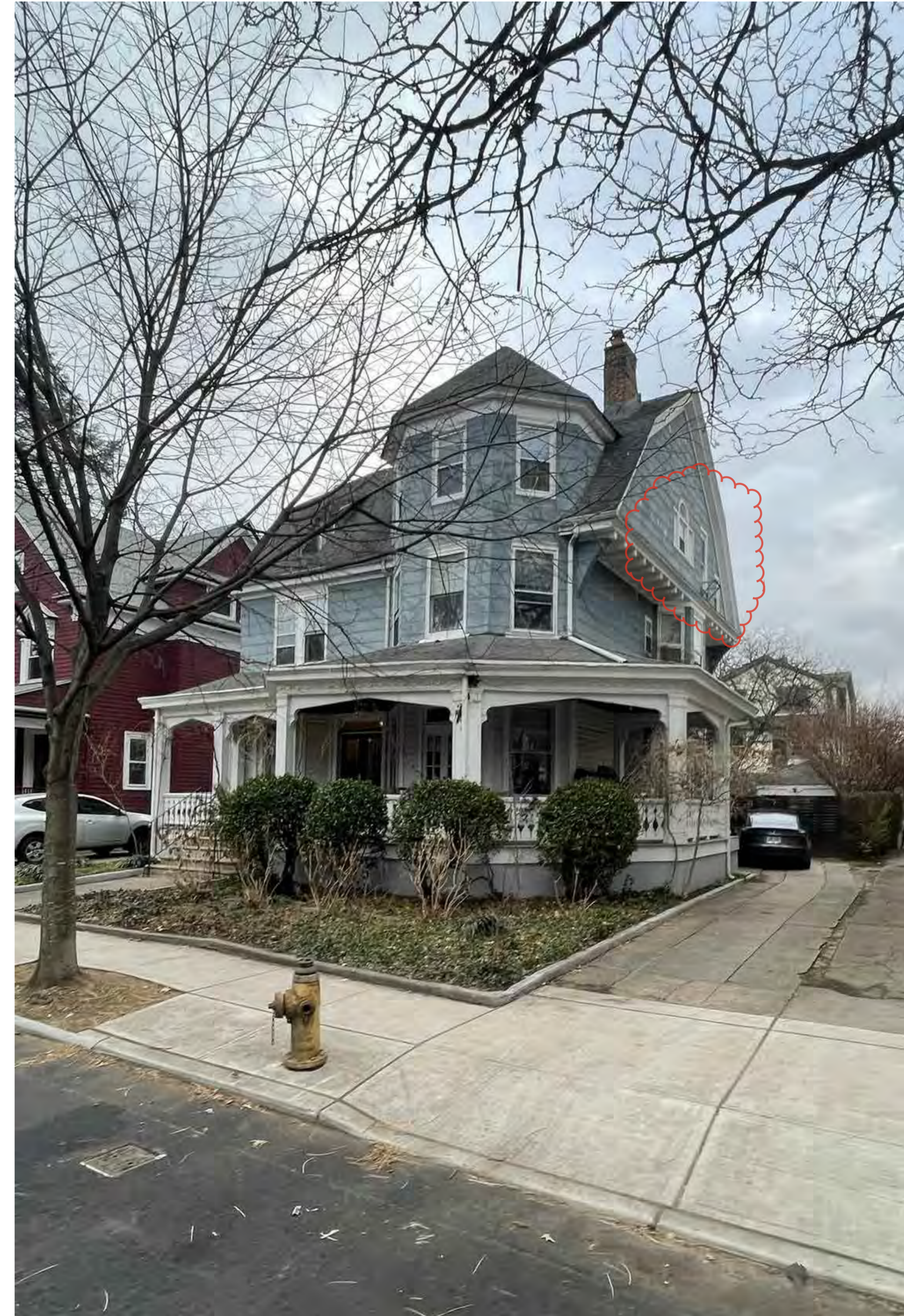
231 ARGYLE RD - SITE VISIT PHOTO SHOWING CURRENT CONDITION
