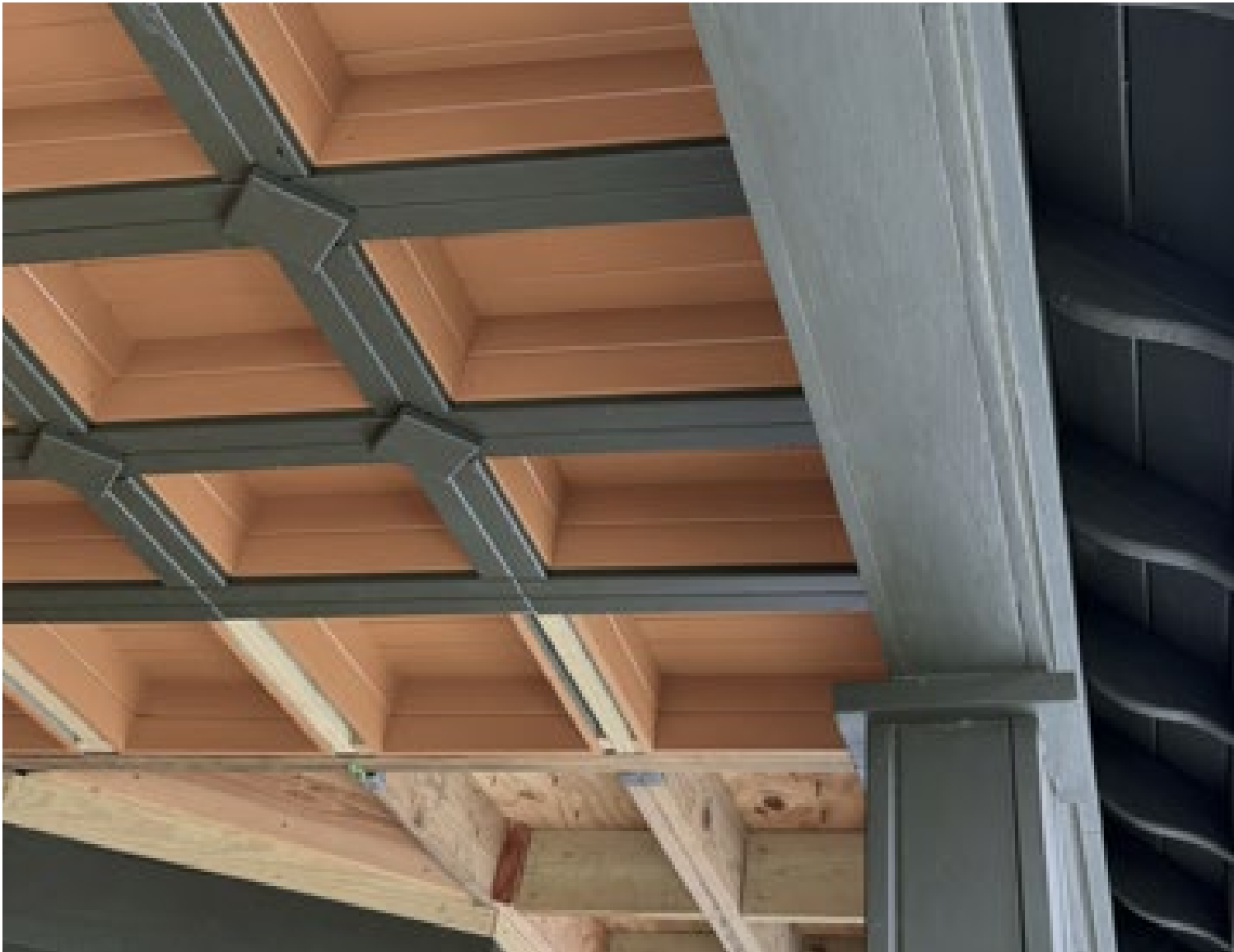
New porch soffit partially visible from the street
