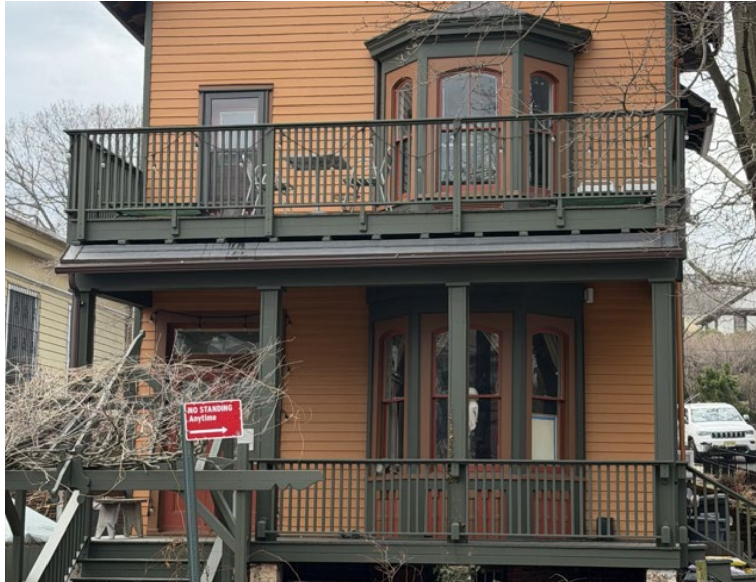
Porch gutter from the front
