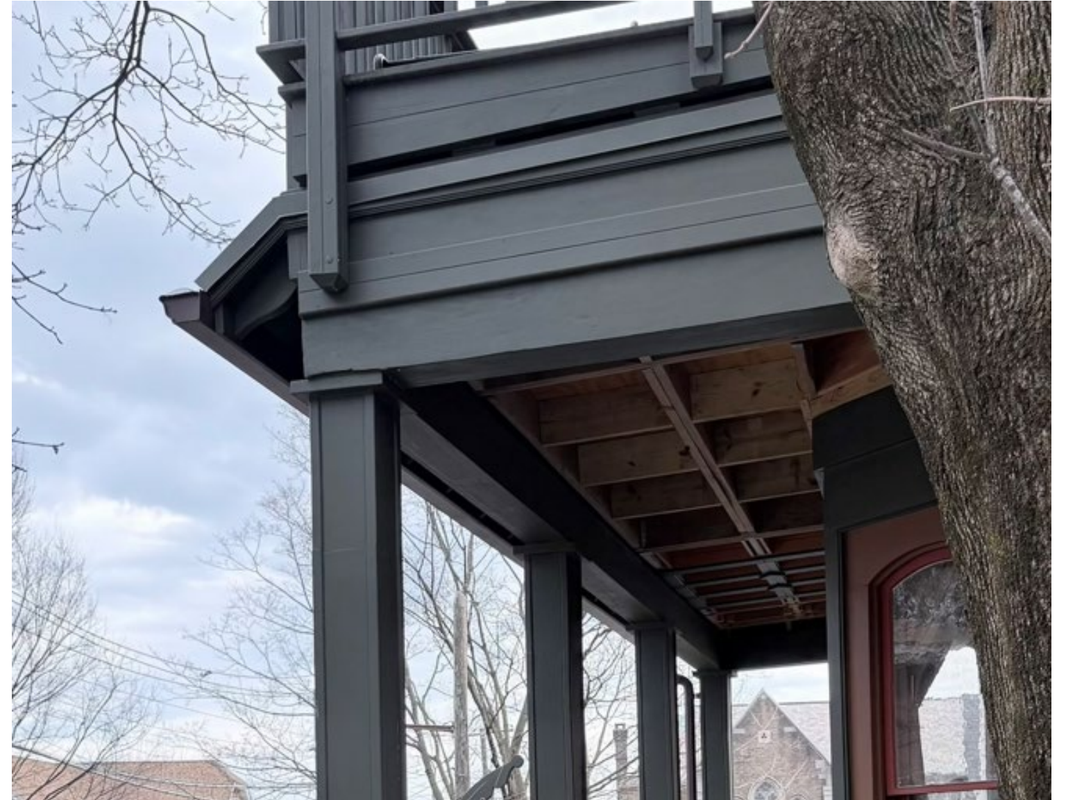
Porch gutter from the side
