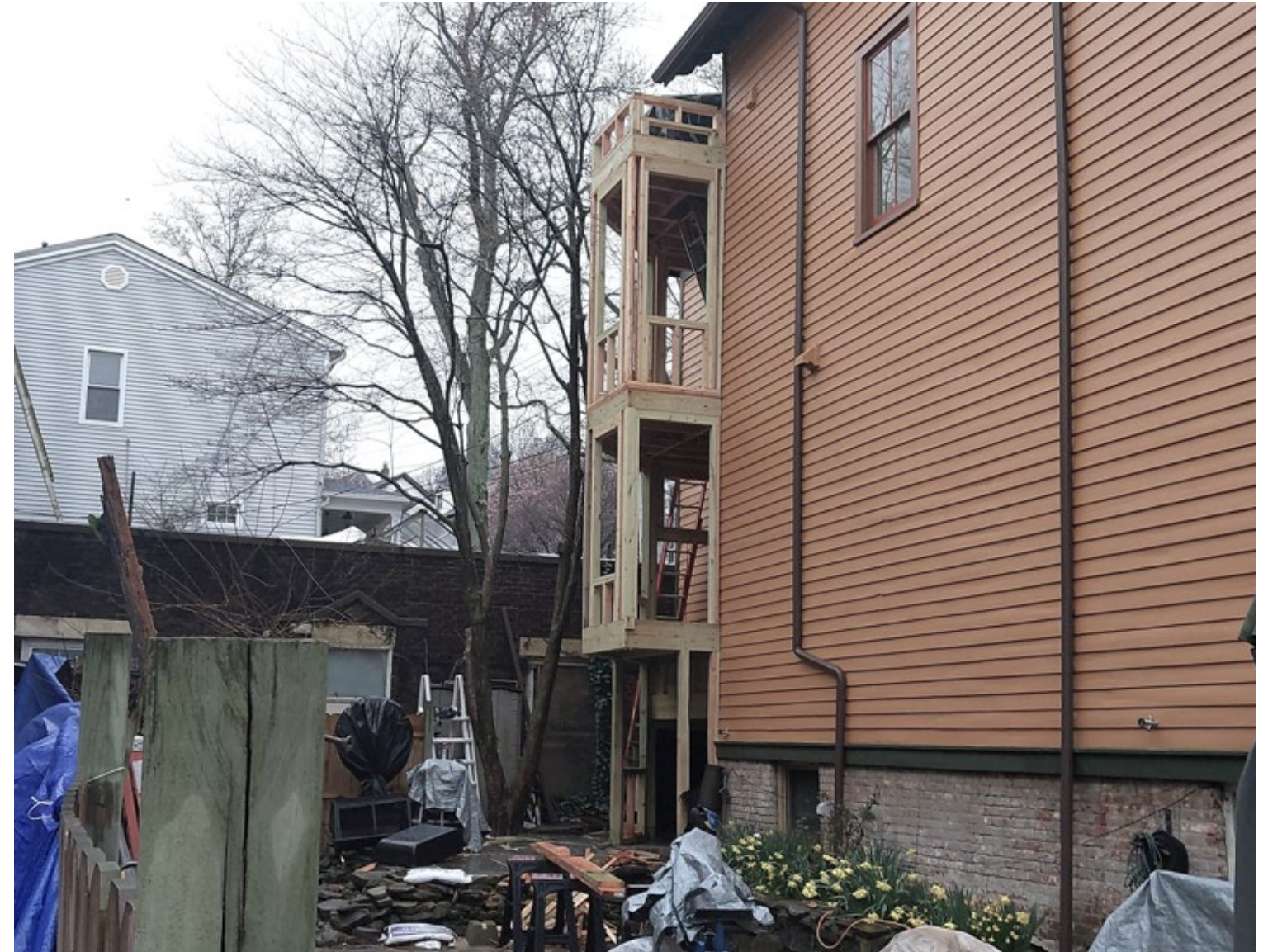
Visibility from Cebra Avenue (above fence)
