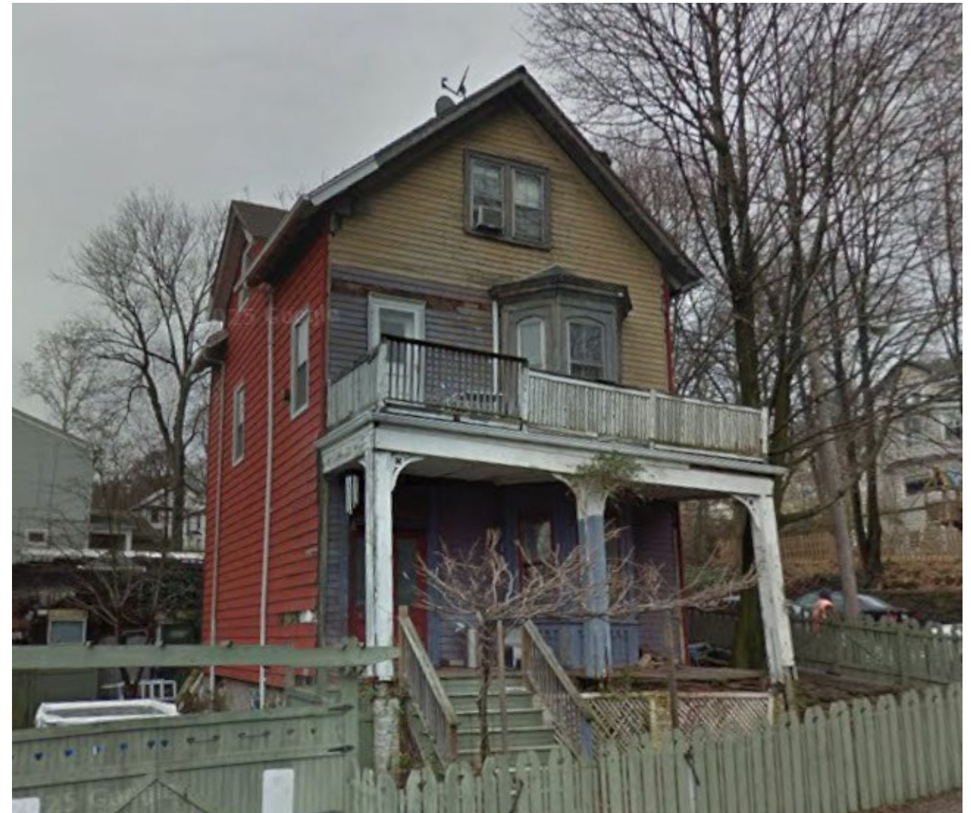
Conditions before work
