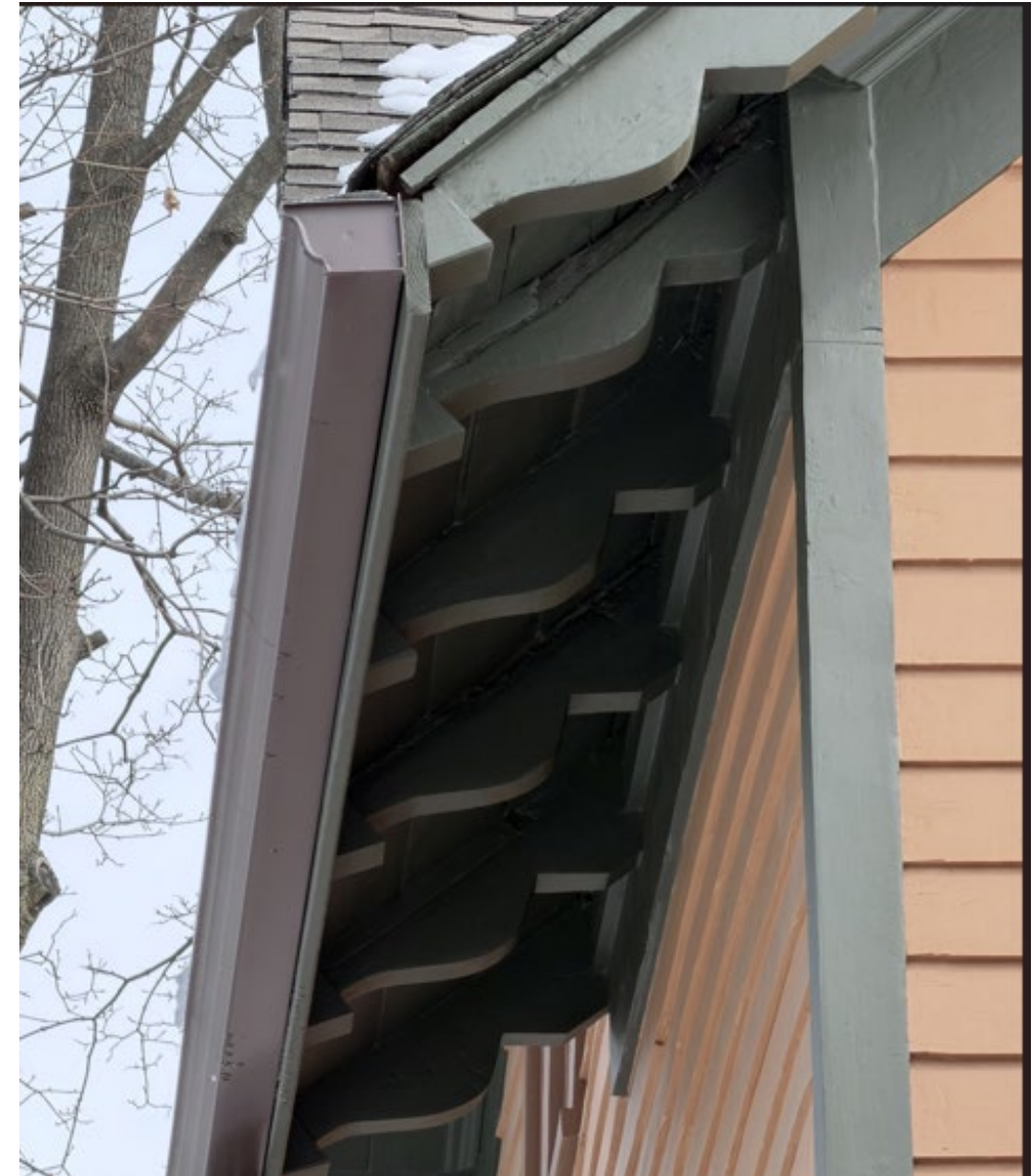
Gutters at side façade matching the new porch
