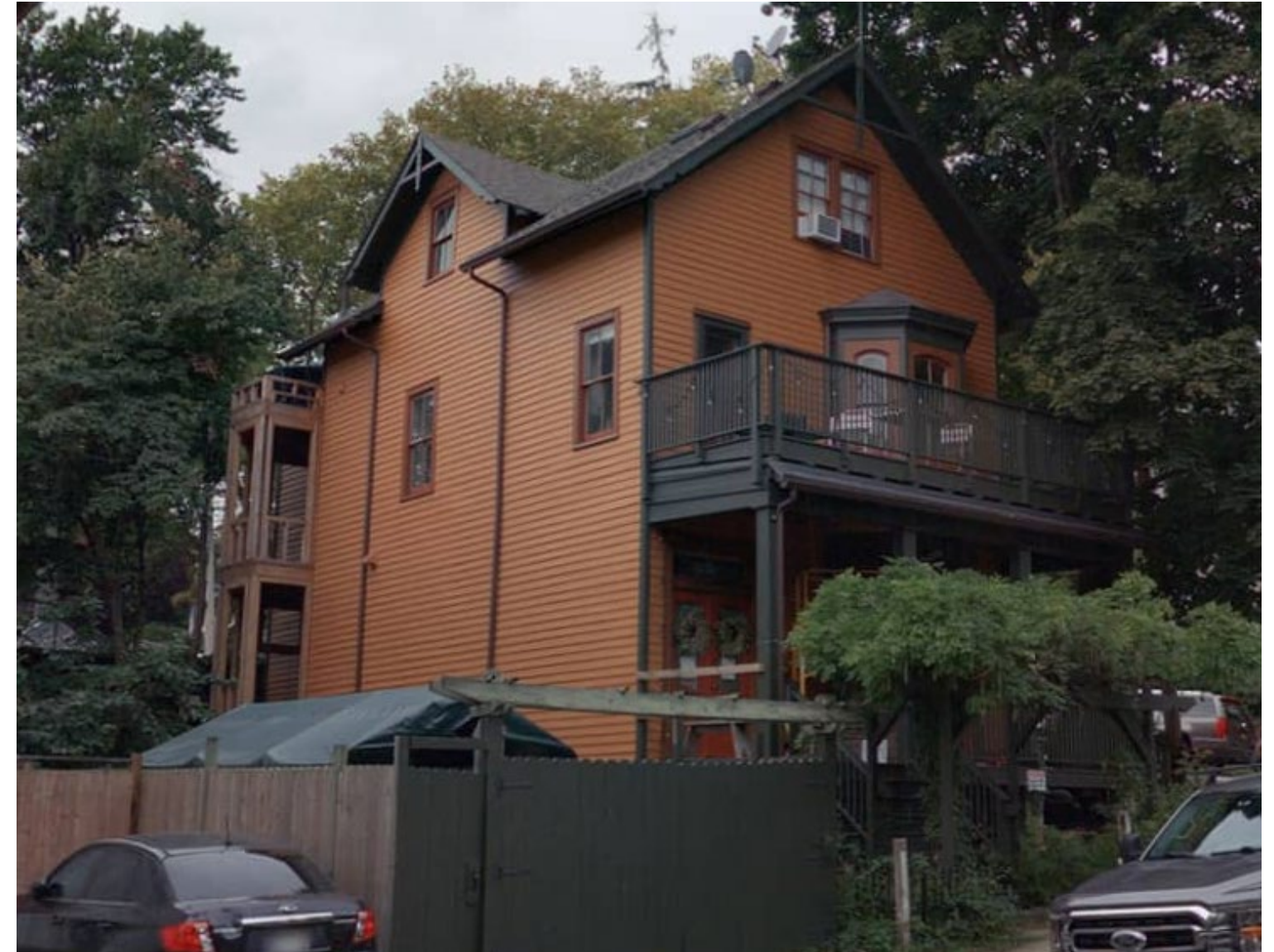
Side façade and extension
