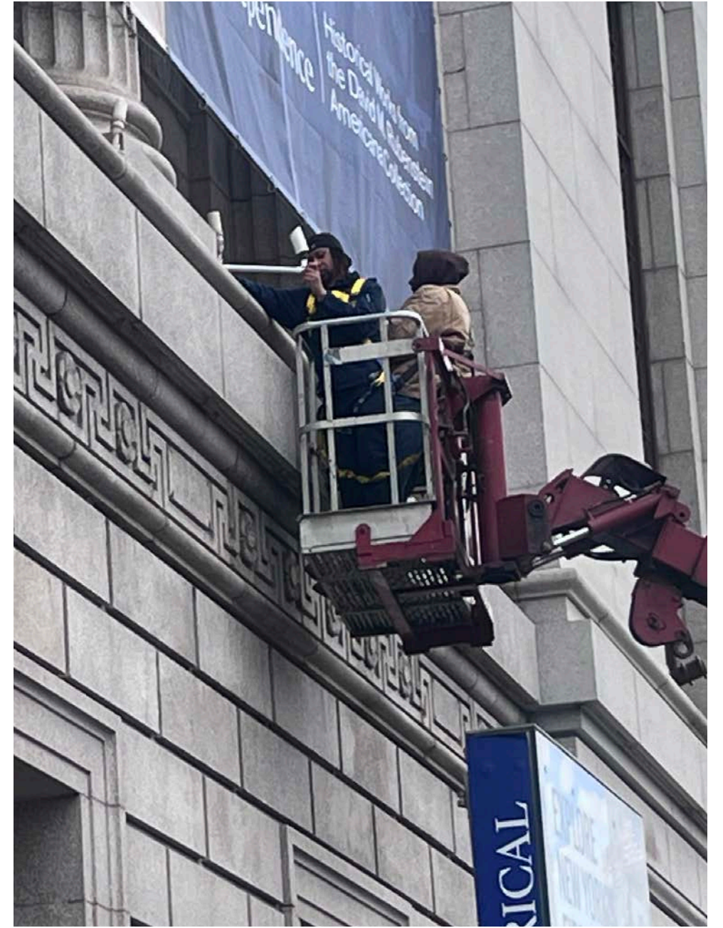
CLOSE-UP OF FIXTURE AT COLONNADE OF CENTRAL PARK WEST FACADE
