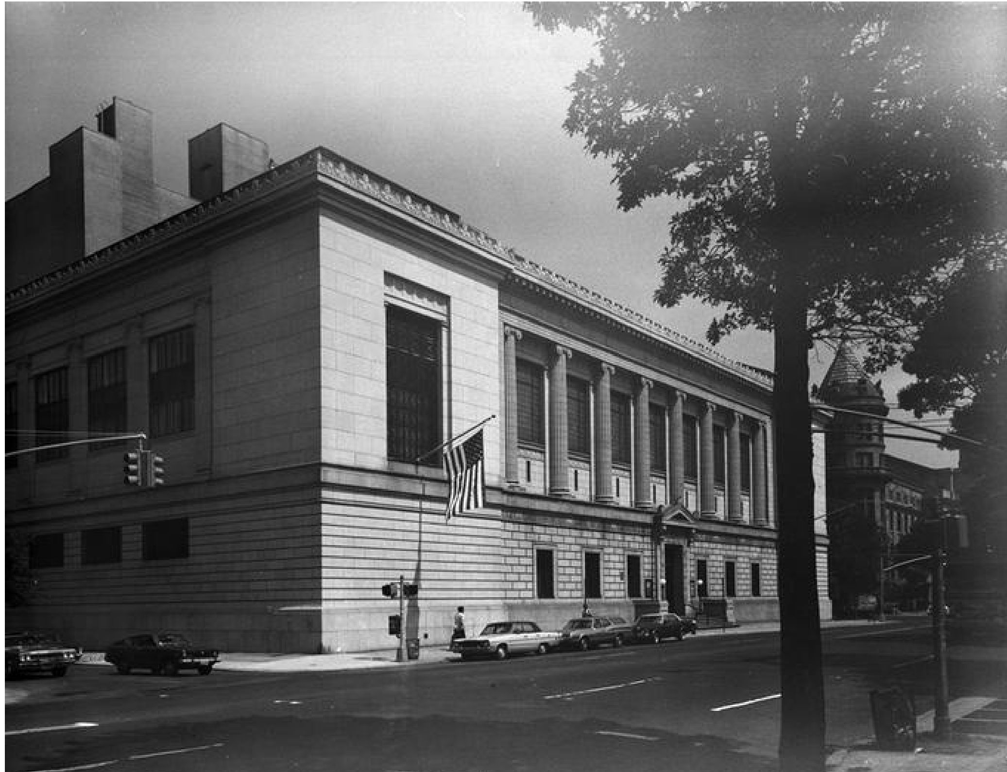
NYH CENTRAL PARK WEST - SOUTHEAST CORNER LOOKING NORTH, C. 1975. SOURCE: THE MUSEUM OF THE CITY OF NEW YORK COLLECTION
