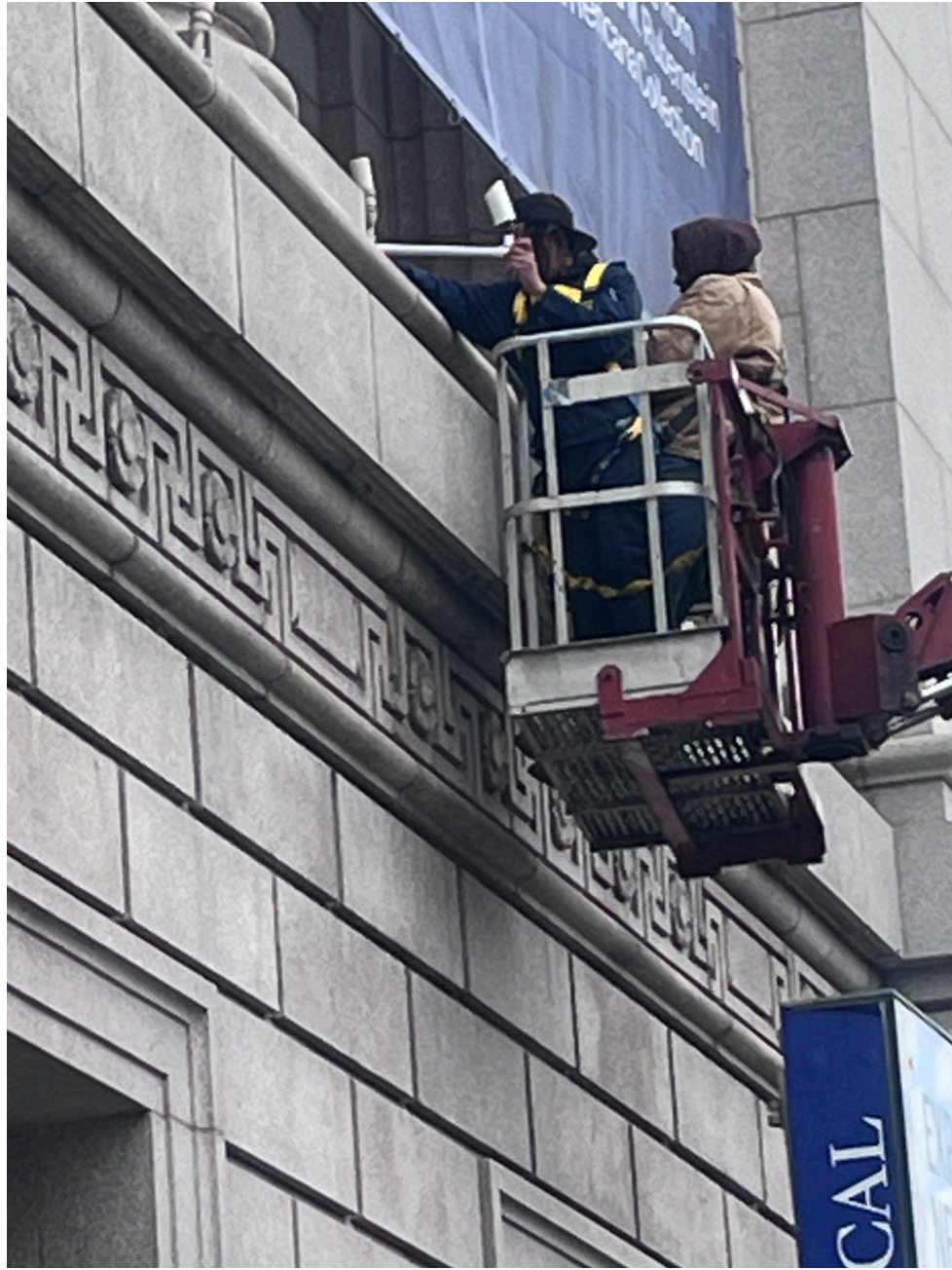
CLOSE-UP OF FIXTURE AT COLONNADE OF CENTRAL PARK WEST FACADE
