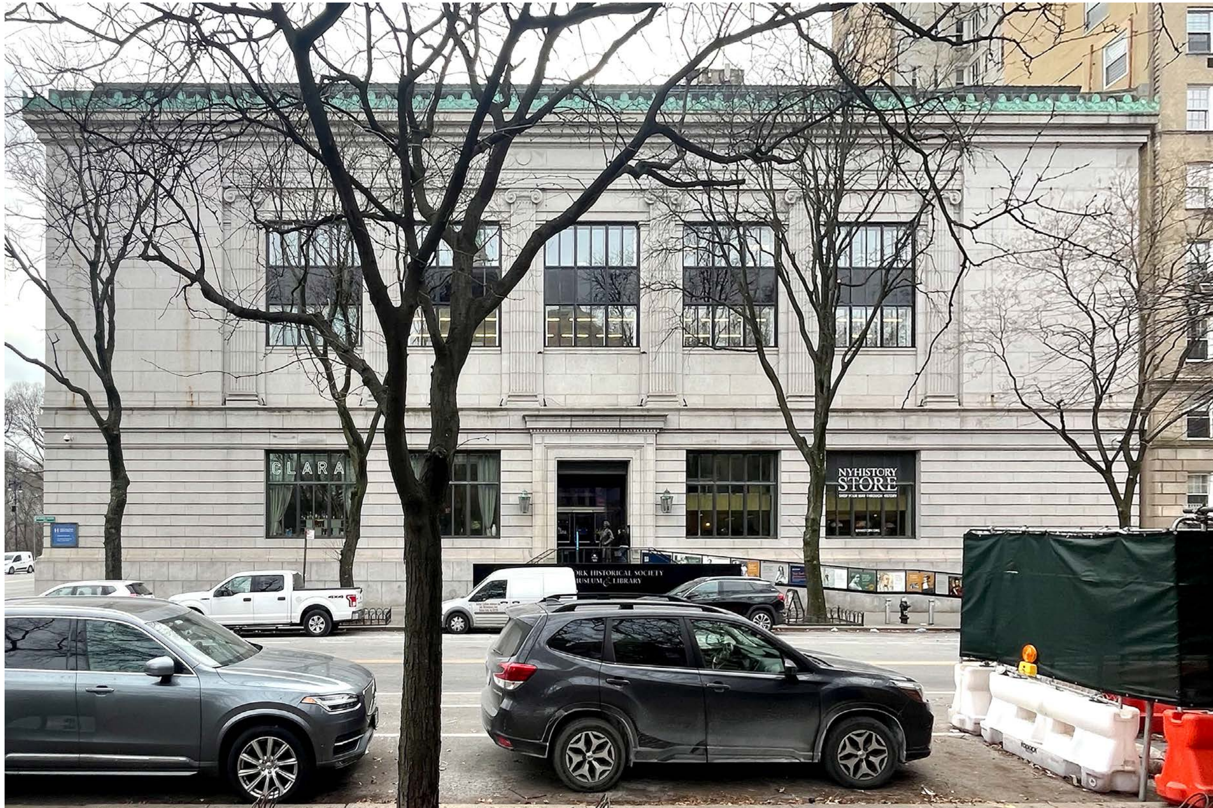
PHOTOGRAPH OF NORTH ELEVATION AT 77TH ST., JANUARY 2026
