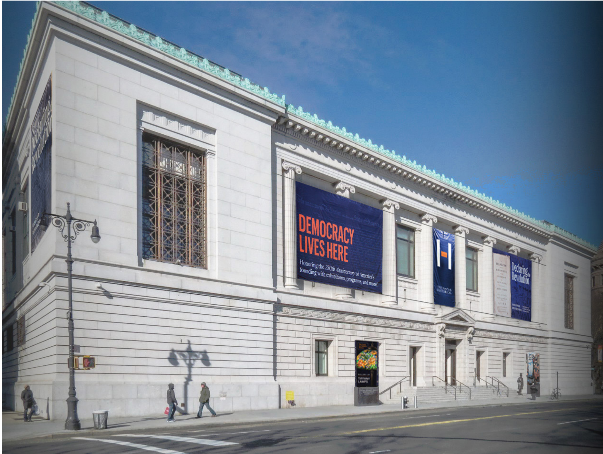
RENDERING OF EAST ELEVATION AT CENTRAL PARK WEST, SOUTHWEST CORNER VIEW, PROPOSED LAYOUT
