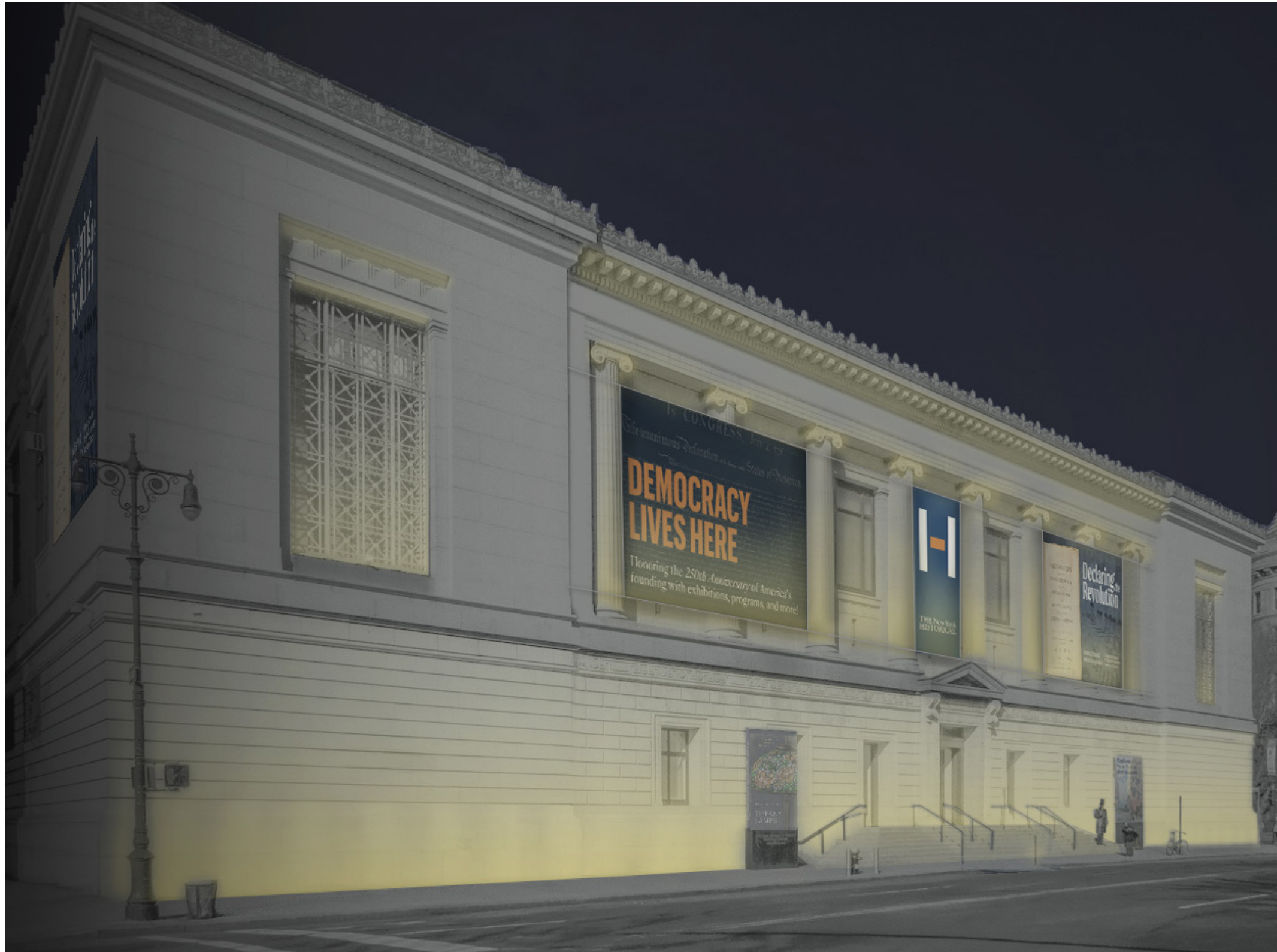
RENDERING OF EAST ELEVATION AT CENTRAL PARK WEST, SOUTHWEST CORNER VIEW, PROPOSED LIGHTING SCHEME
