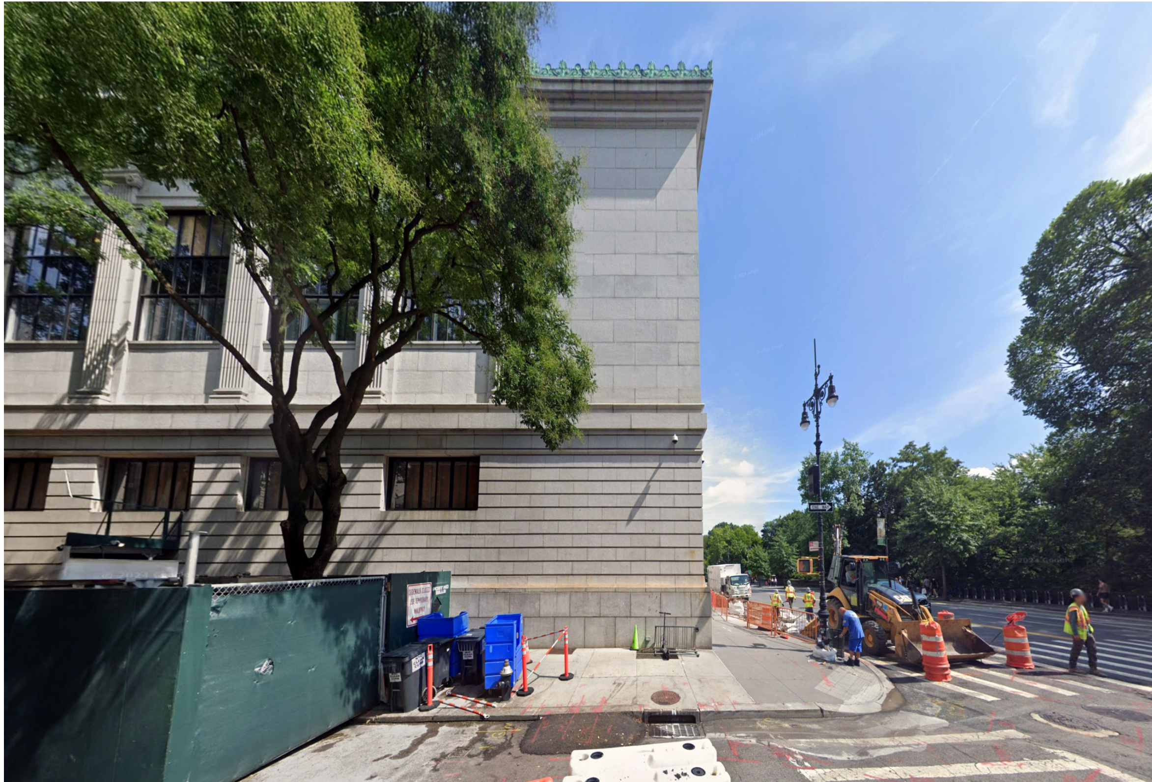
PHOTOGRAPH OF SOUTH ELEVATION AT 76TH ST., SEPTEMBER 2025
