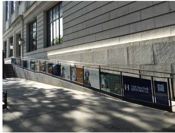
7 Ramp Handrail Signage at North Elevation
