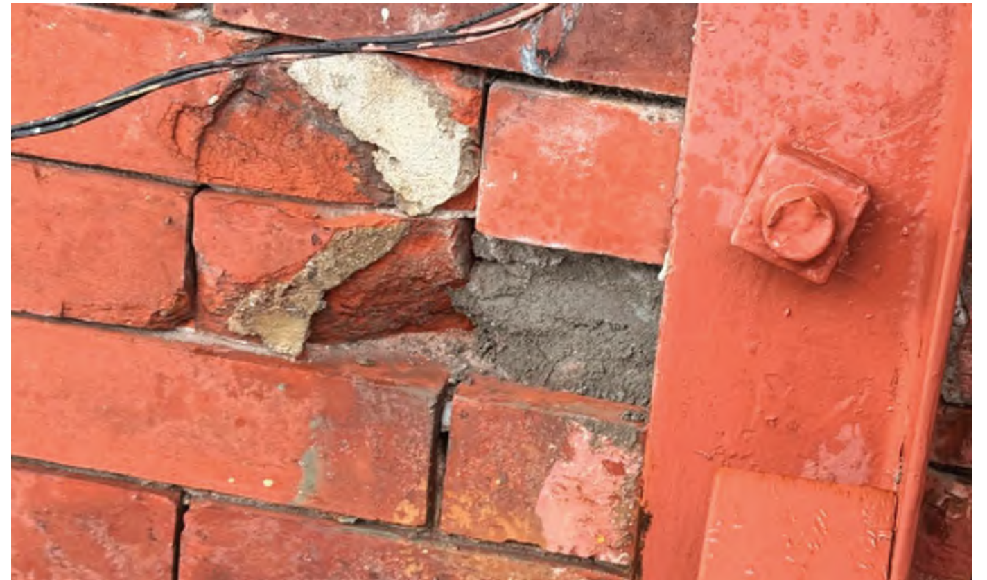
4 Missing/Damaged Brick
