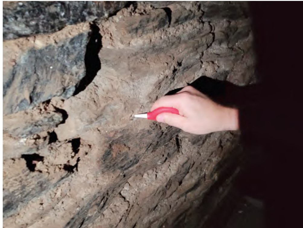
CLEARING DUST FROM TEST SITE
