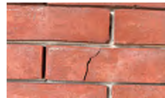
3. BRICK CRACK
