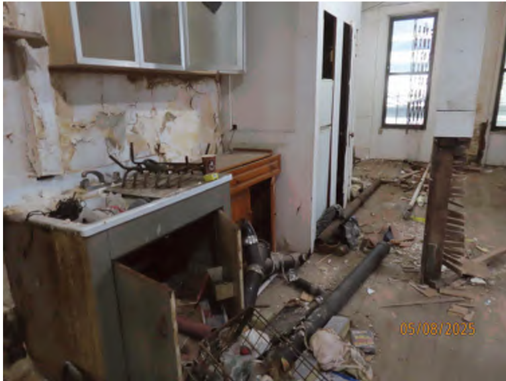
CURRENT CONDITION OF INTERIOR (TYPICAL)
