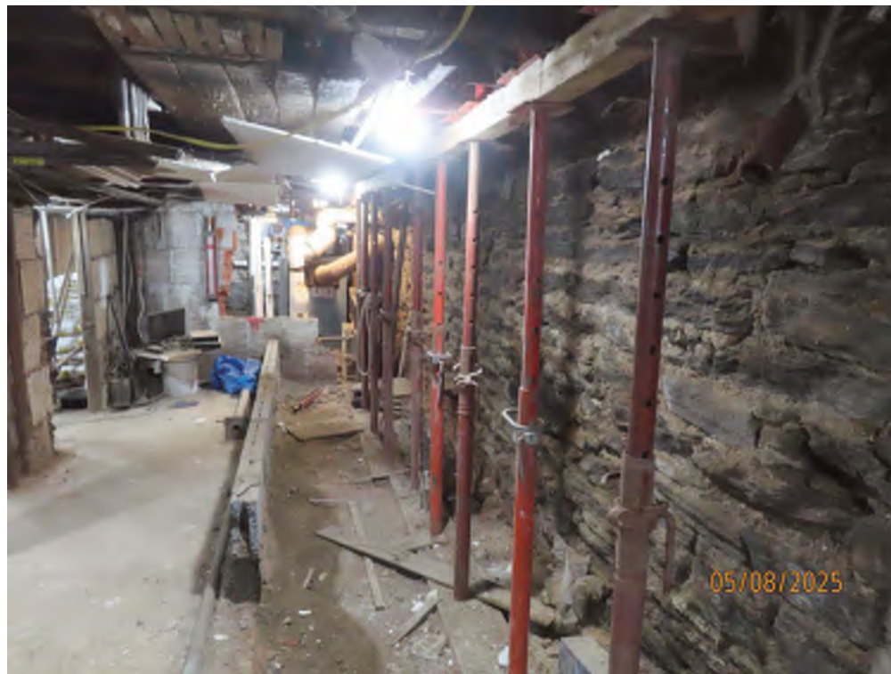
CURRENT CONDITION AT CELLAR
