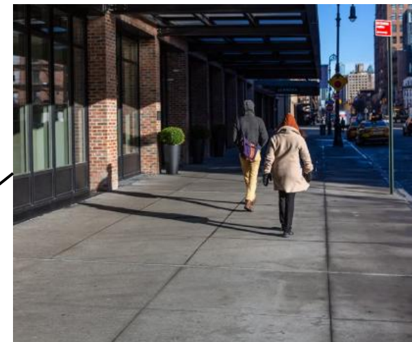
4"/7" PIGMENTED CONCRETE SIDEWALK
