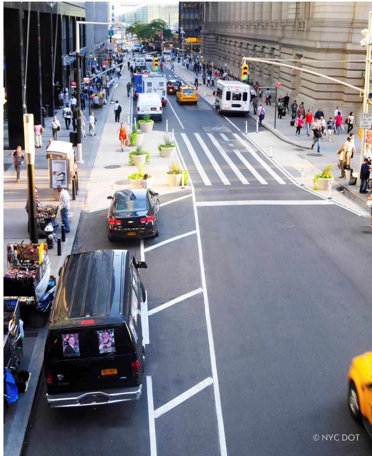
Adjacent to location No.3: Broadway and Bowling Green, looking South
