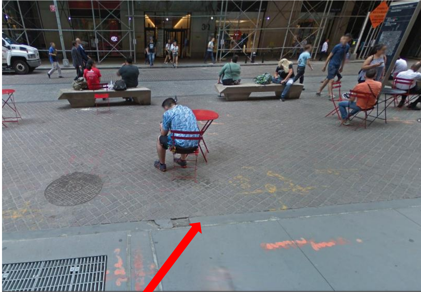
Existing curb preserved to maintain historic alignment
