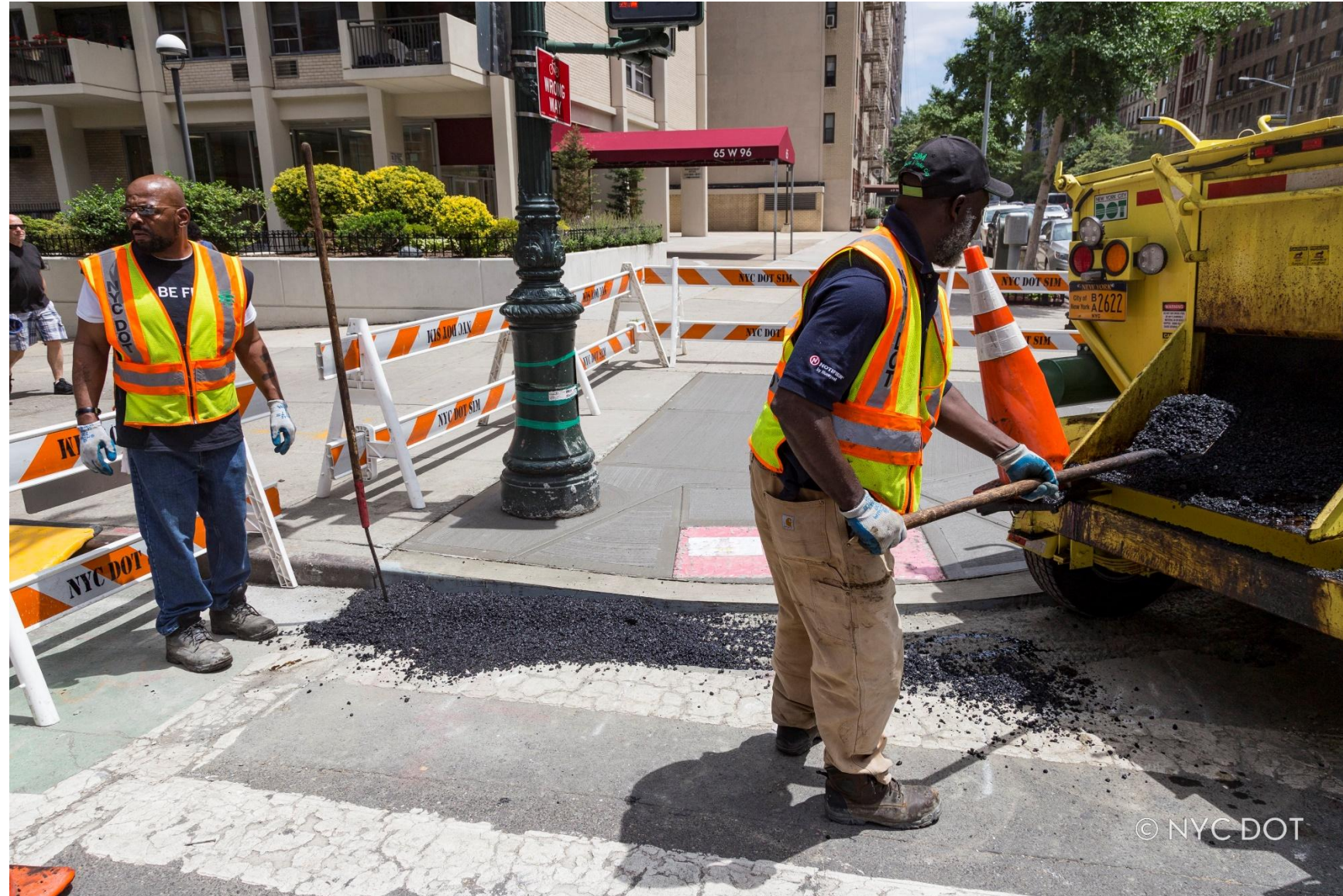
Pedestrian Ramp Installation
