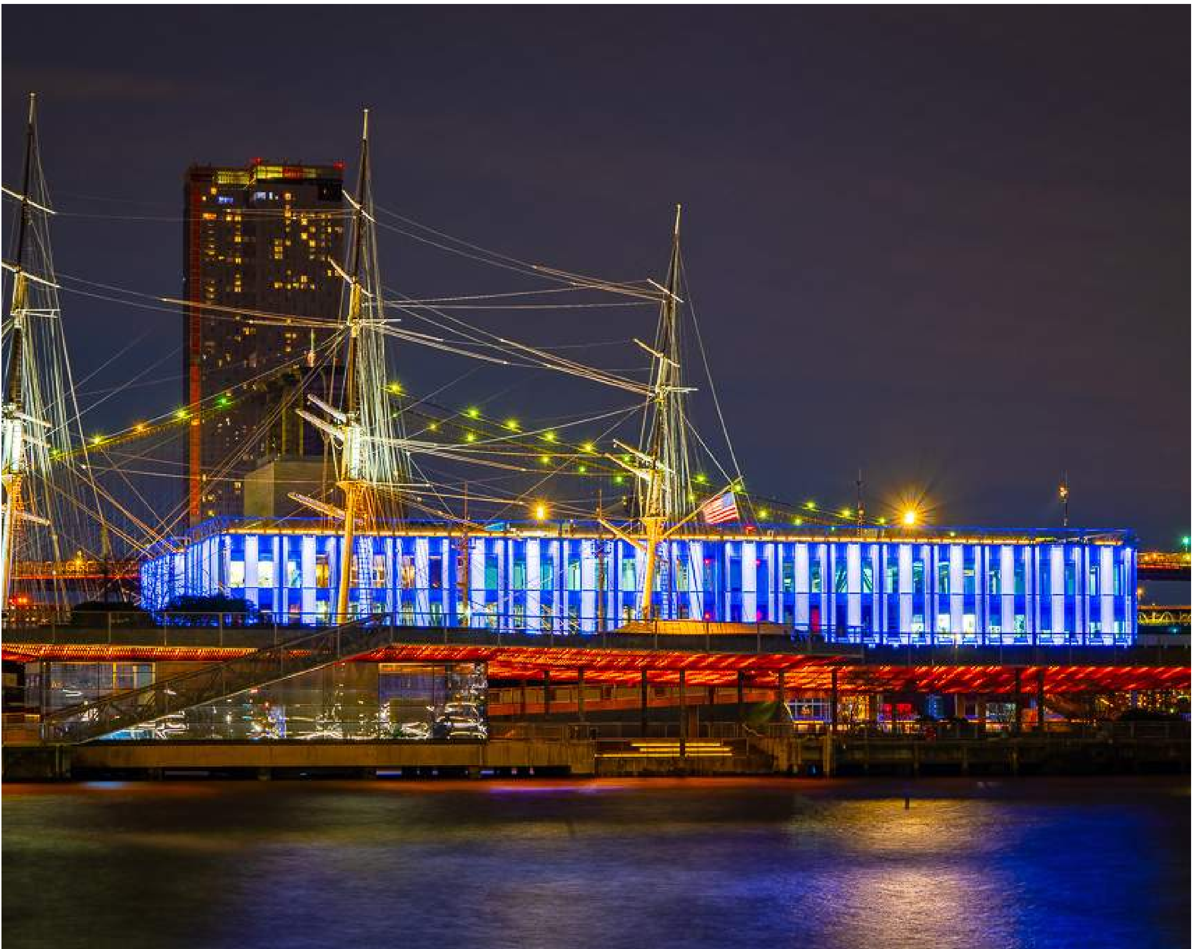
Exterior Views from South
