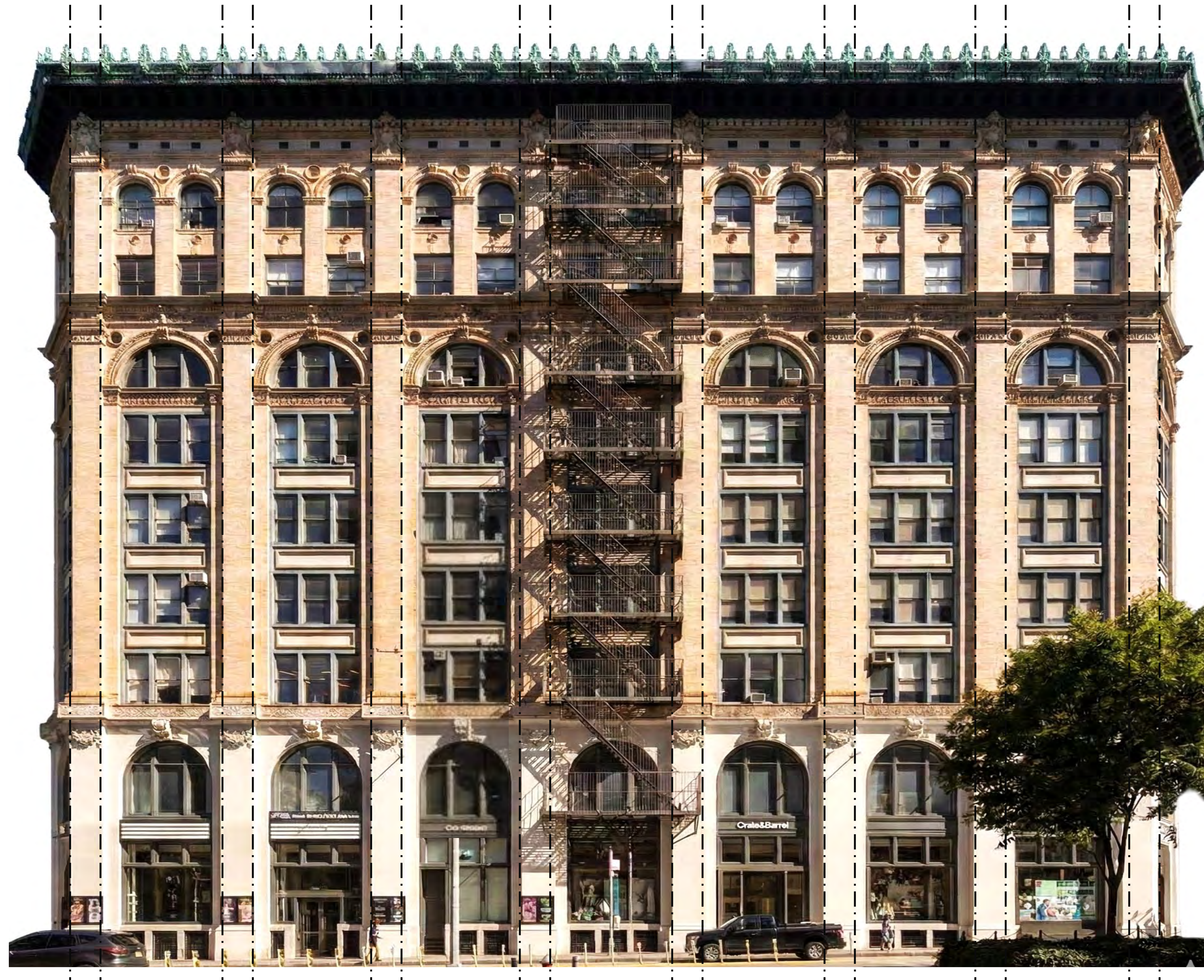
Cable Building , 611 Broadway at Houston St
