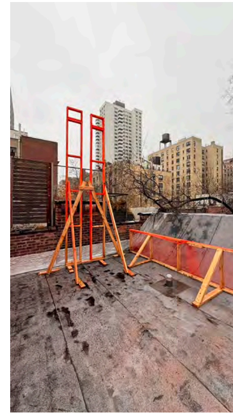
B. Front Chimney Flue and Railing
