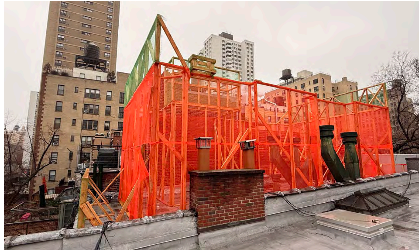
E. Rear of Mockup looking NW
