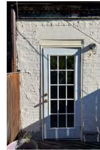
32 West 95th Street Top Floor Rear Facade
