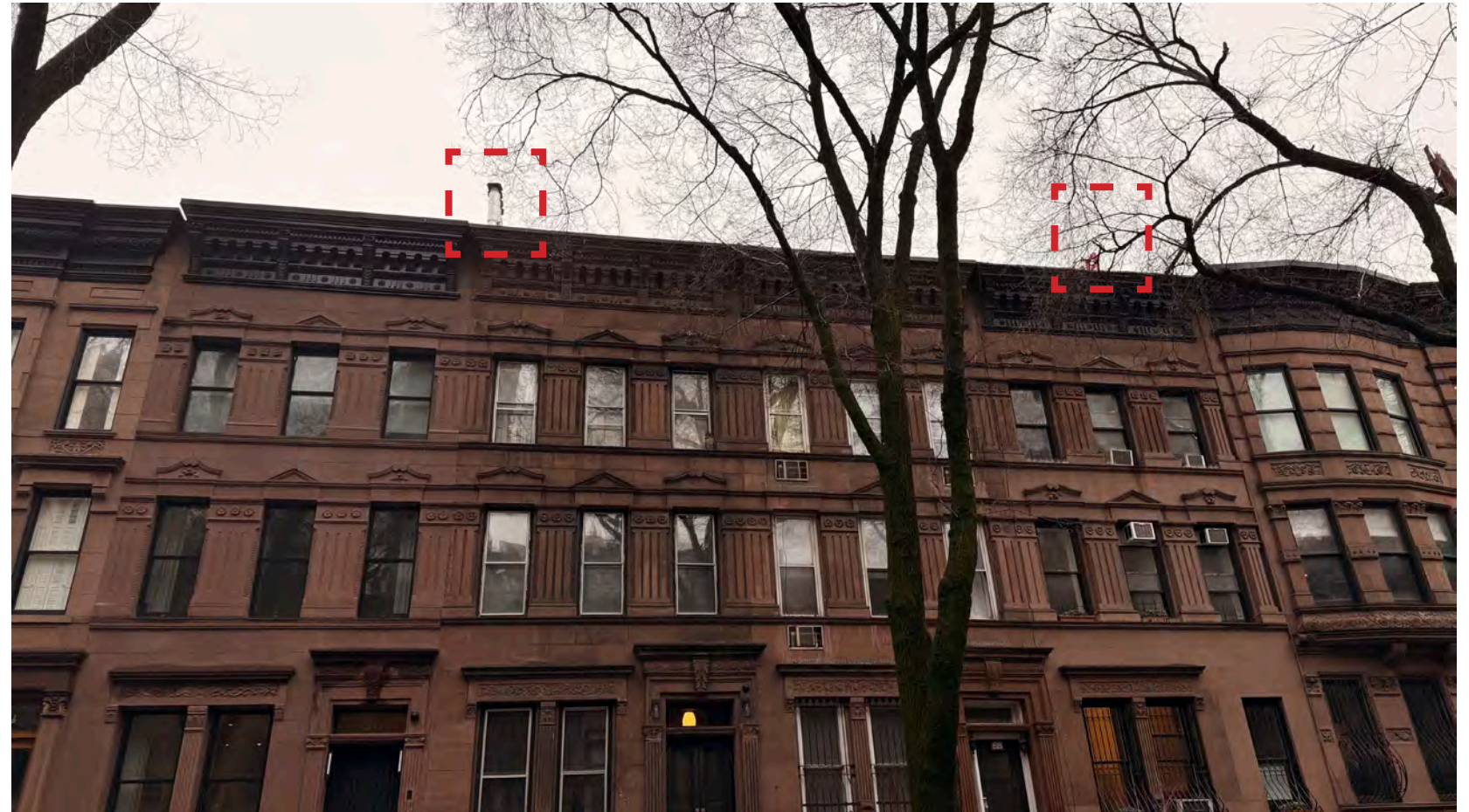
J - Wide angle View from 31 W 95th St. show flue mockup and neighboring flue
