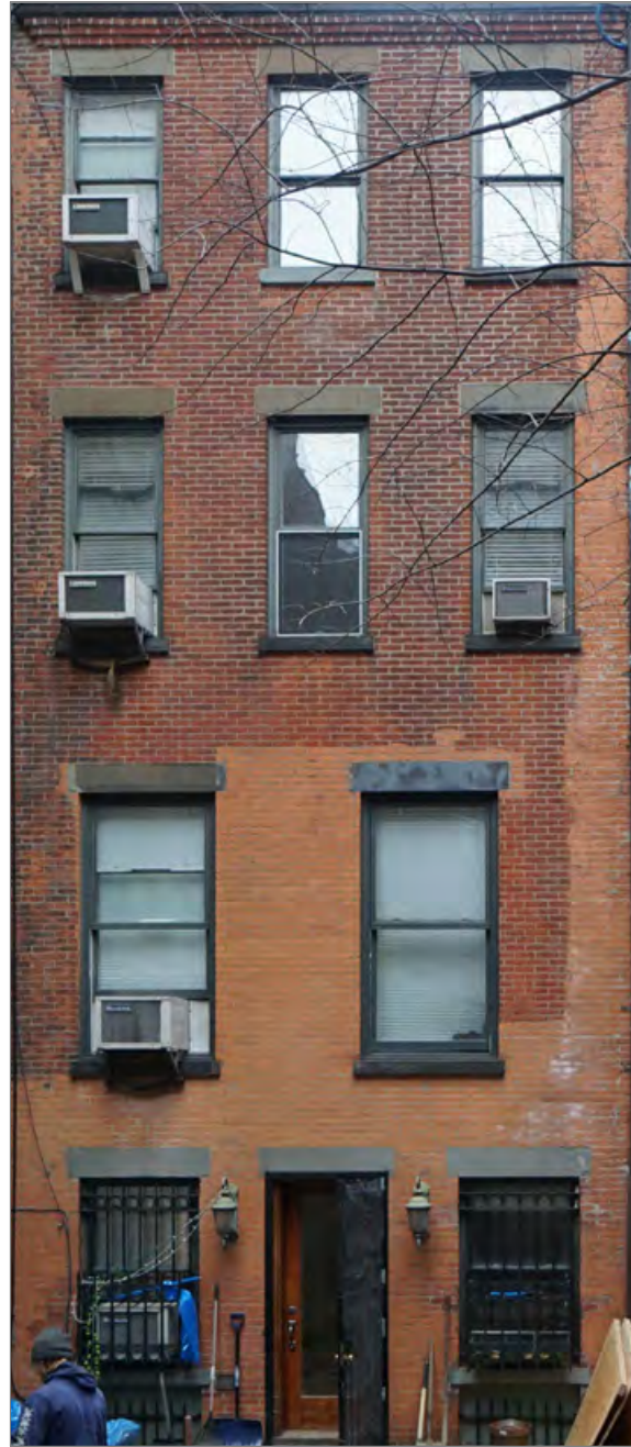
Exist. Rear Facade
