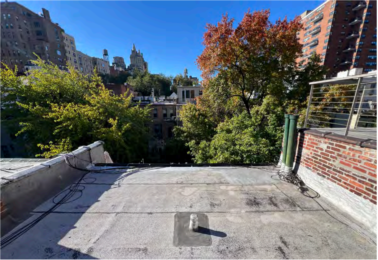
SOUTH - Looking Towards Rear Facade
