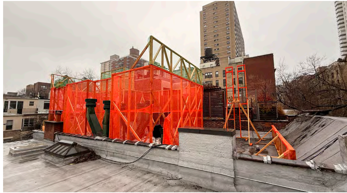
A. Front of Mockup looking SW
