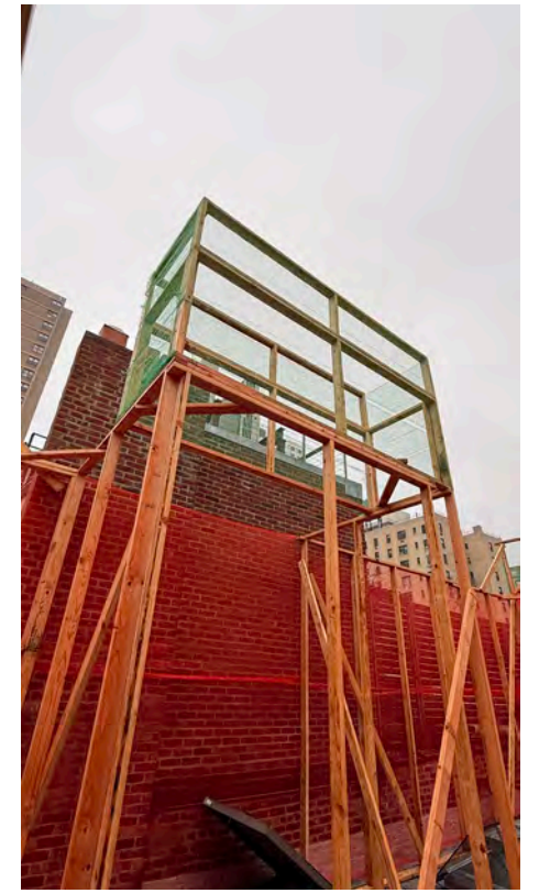
C. HVAC Unit Mockup above Addition
