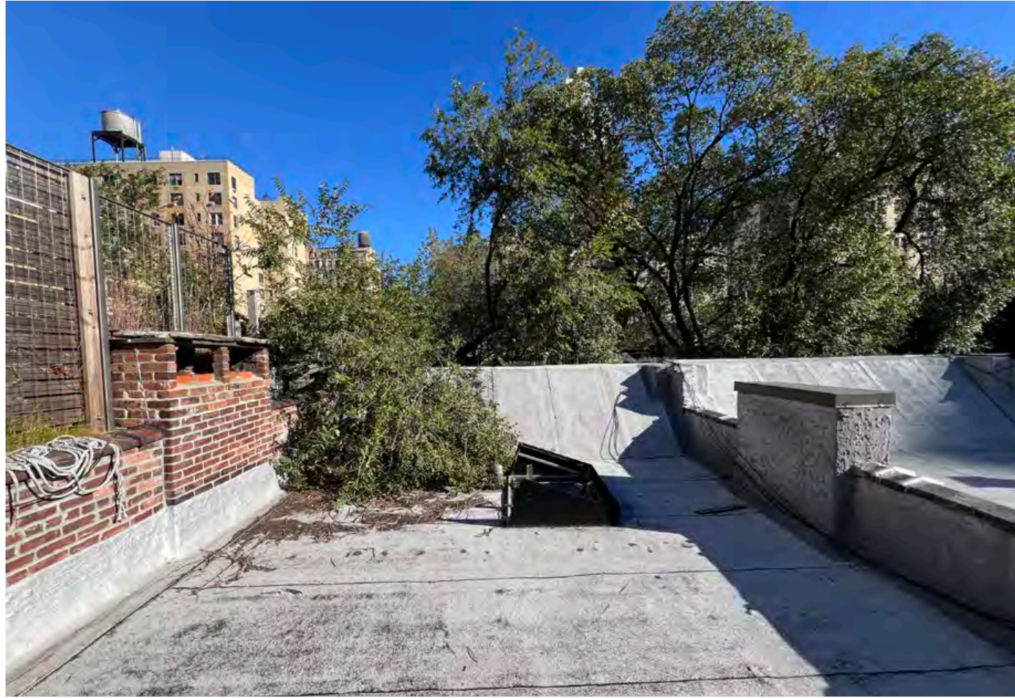
NORTH - Looking Towards Front Facade
