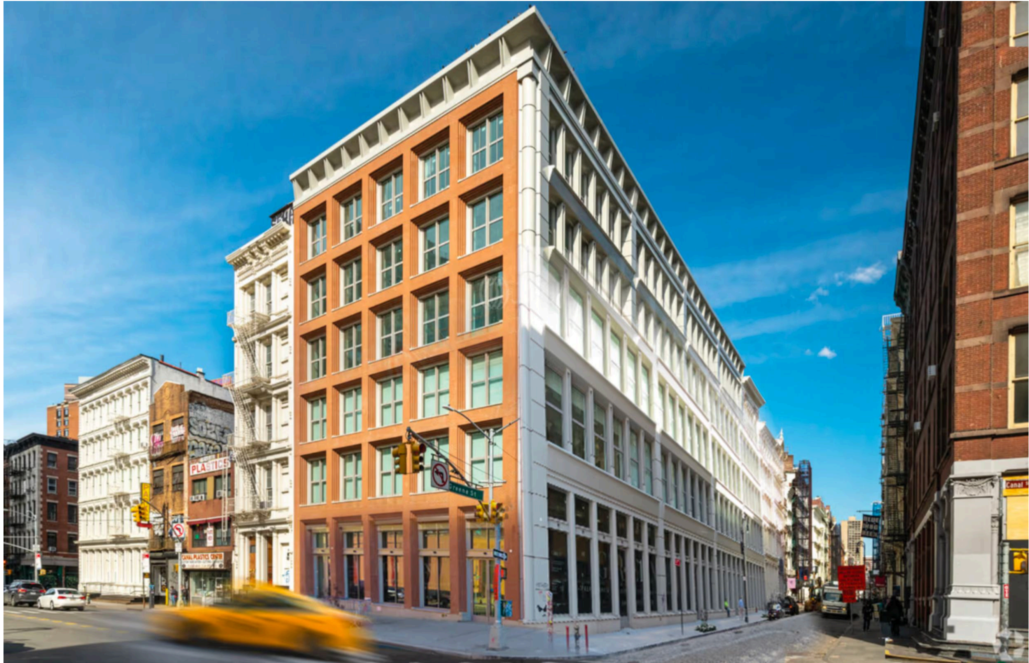
Ⓔ SoHo Cast Iron Historic District 11 Greene Street, Gene Kaufman Architect, Approved 2014
