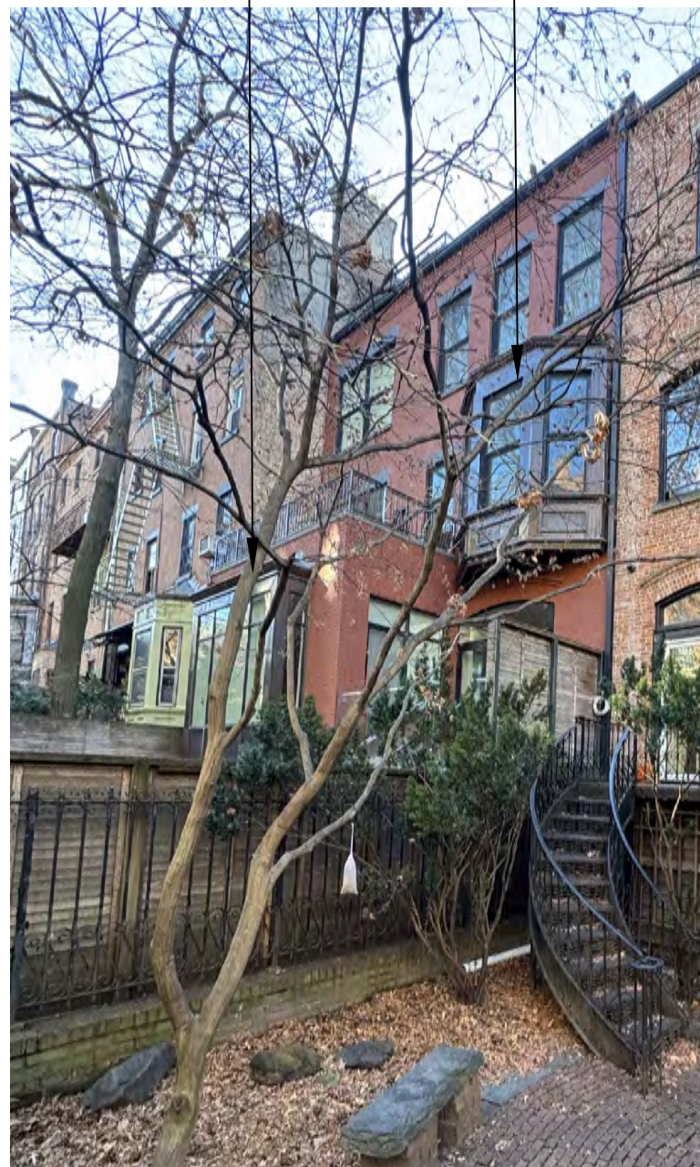
19 MONTGOMERY PL.- REAR FACADE
