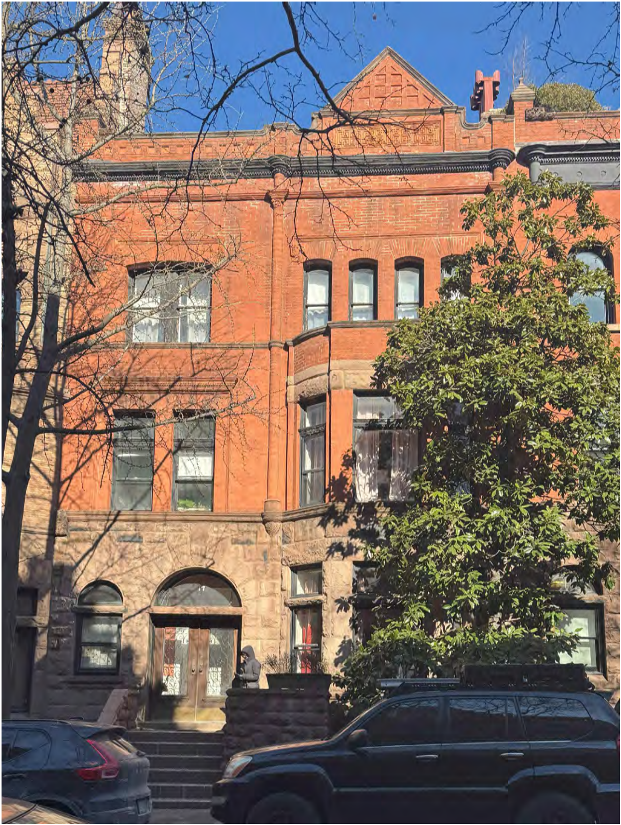
EXISTING FRONT FACADE
