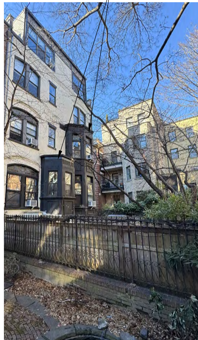
11 MONTGOMERY PL.- REAR FACADE
