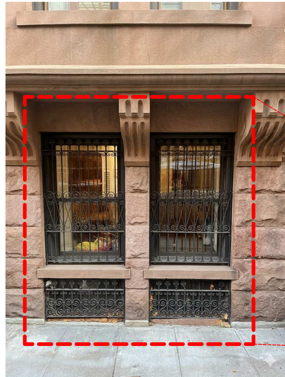
EXISTING CONDITION OF WINDOW AND IRON GRILLES
