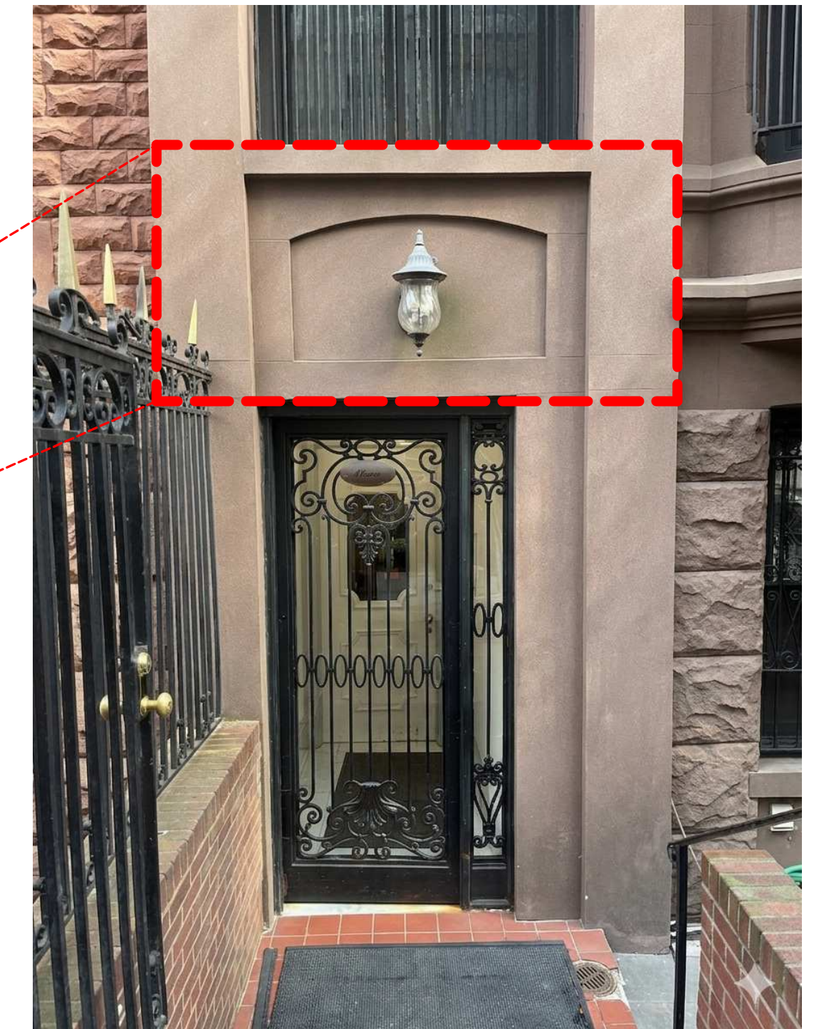
ENTRANCE CONDITION OF 11 W 74TH ST./LOT 25
