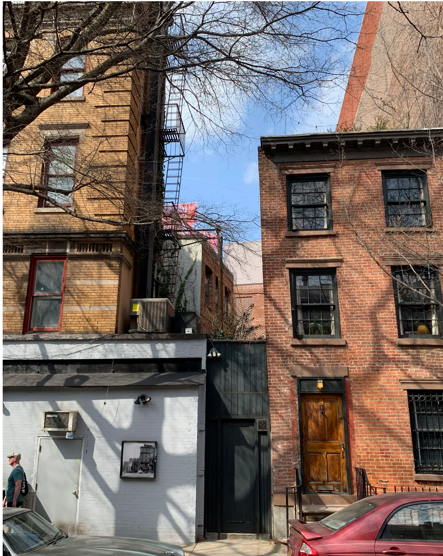
View north into corner rear yards from Bank Street with a view of the proposed stair bulkhead and mechanical enclosure
