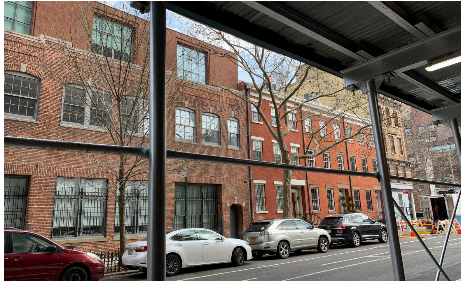
View to the southeast along Washington, guardrail is minimally visible at the primary facade roof deck
