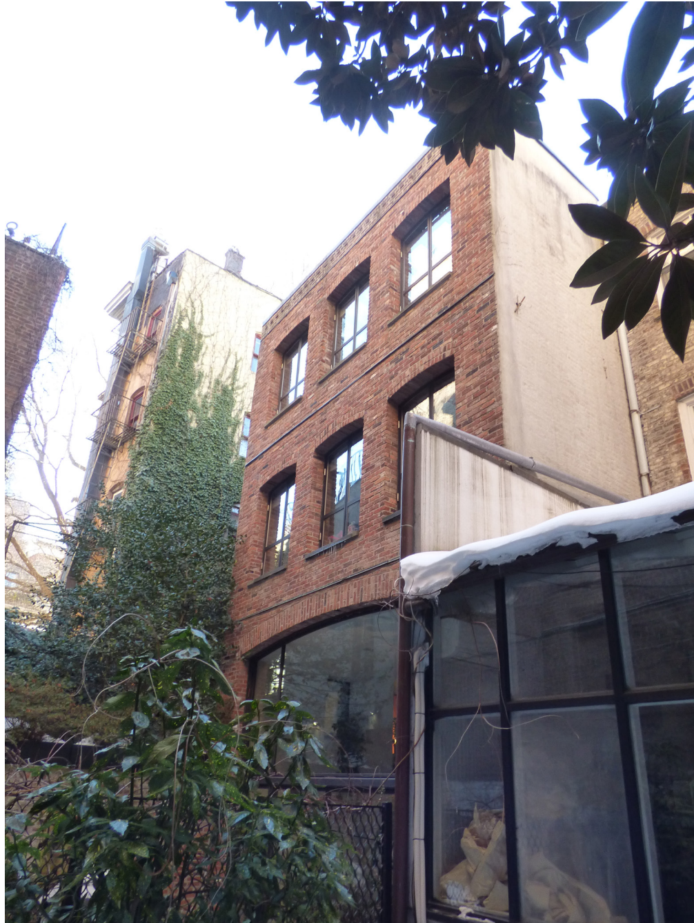
Rear yard, facing southwest
