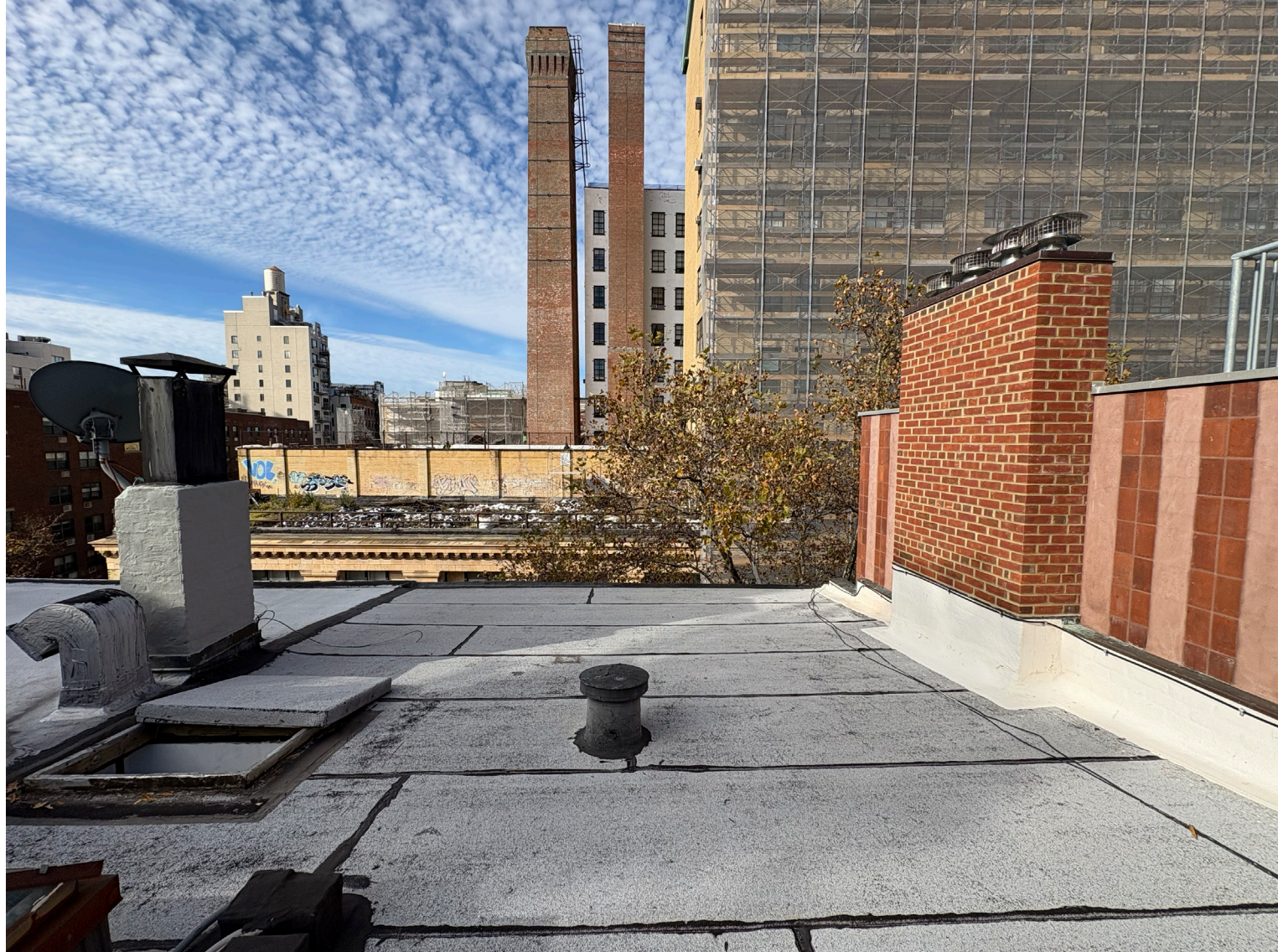
View of the roof - looking west
