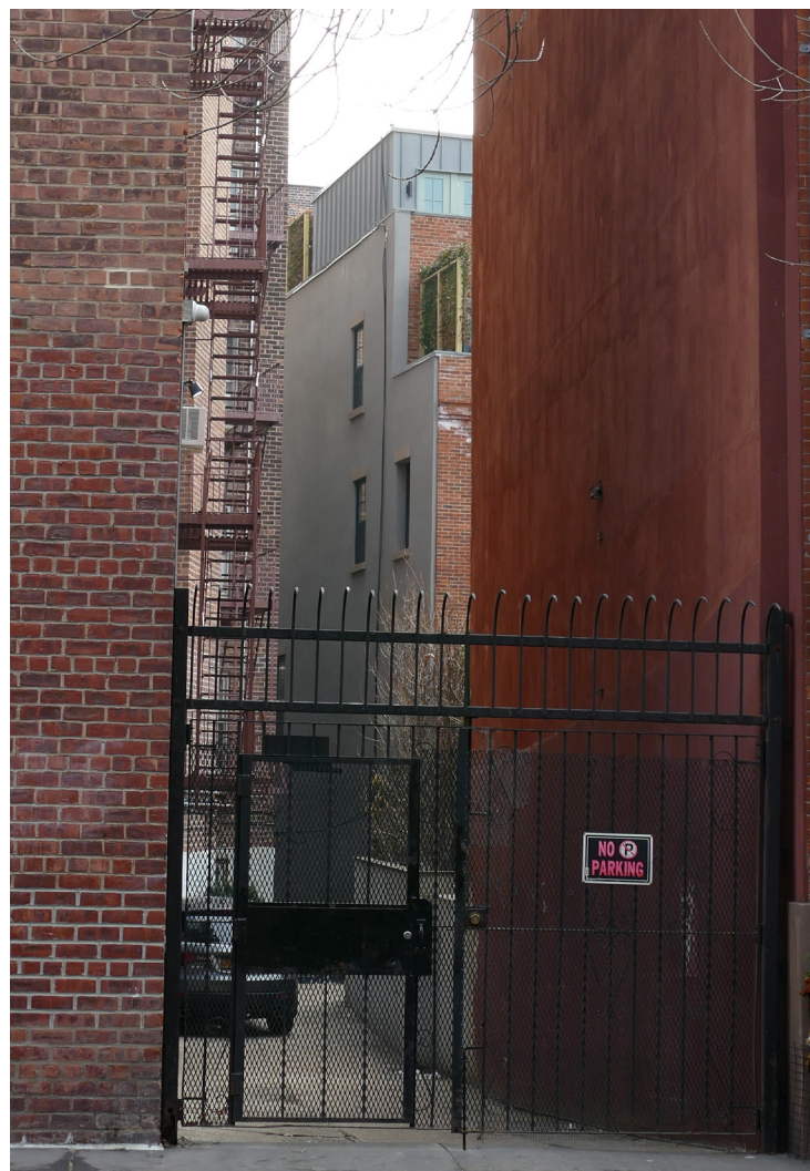
105-107 Bank Street, Rear Elevation
