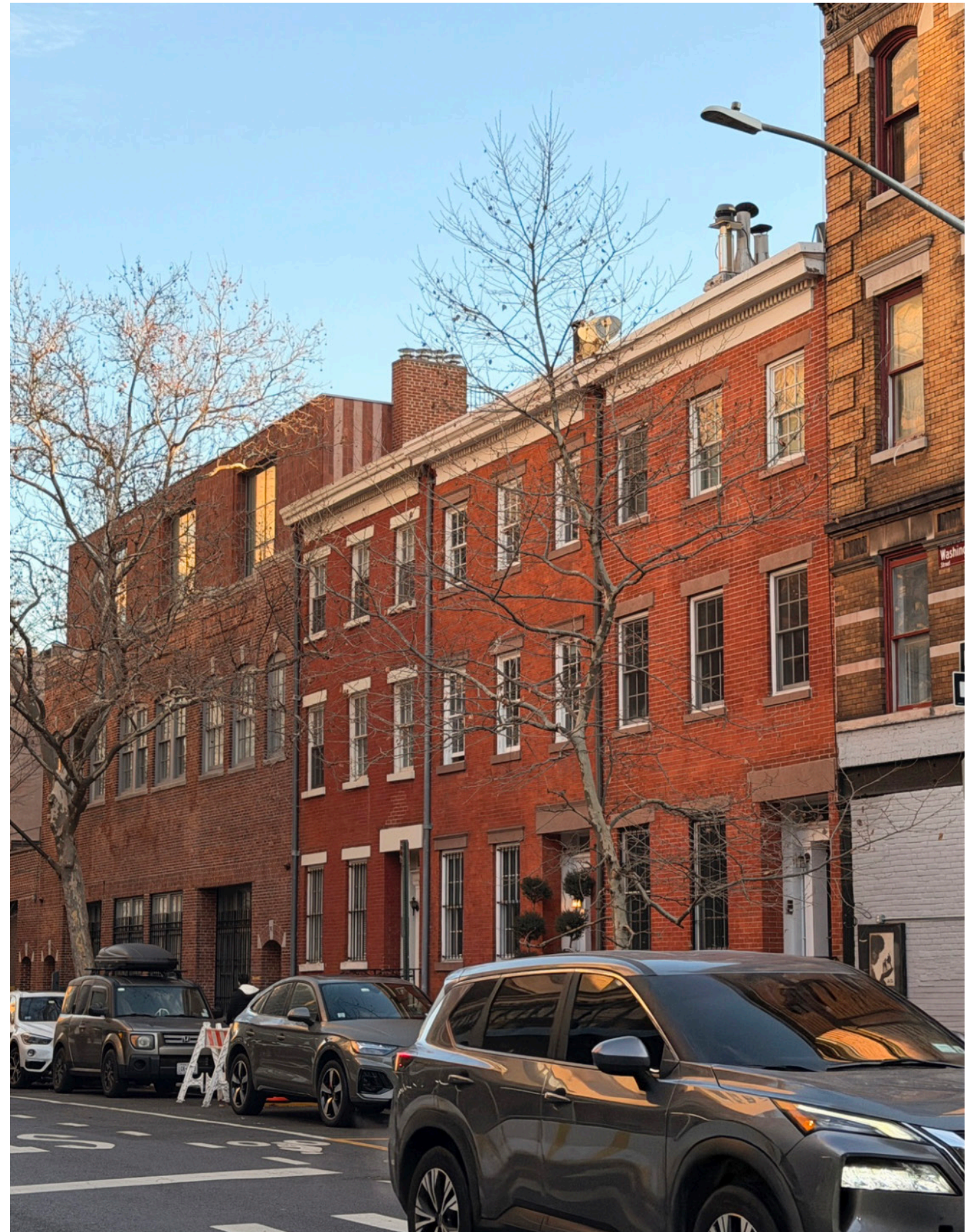
Front facade, facing northeast
