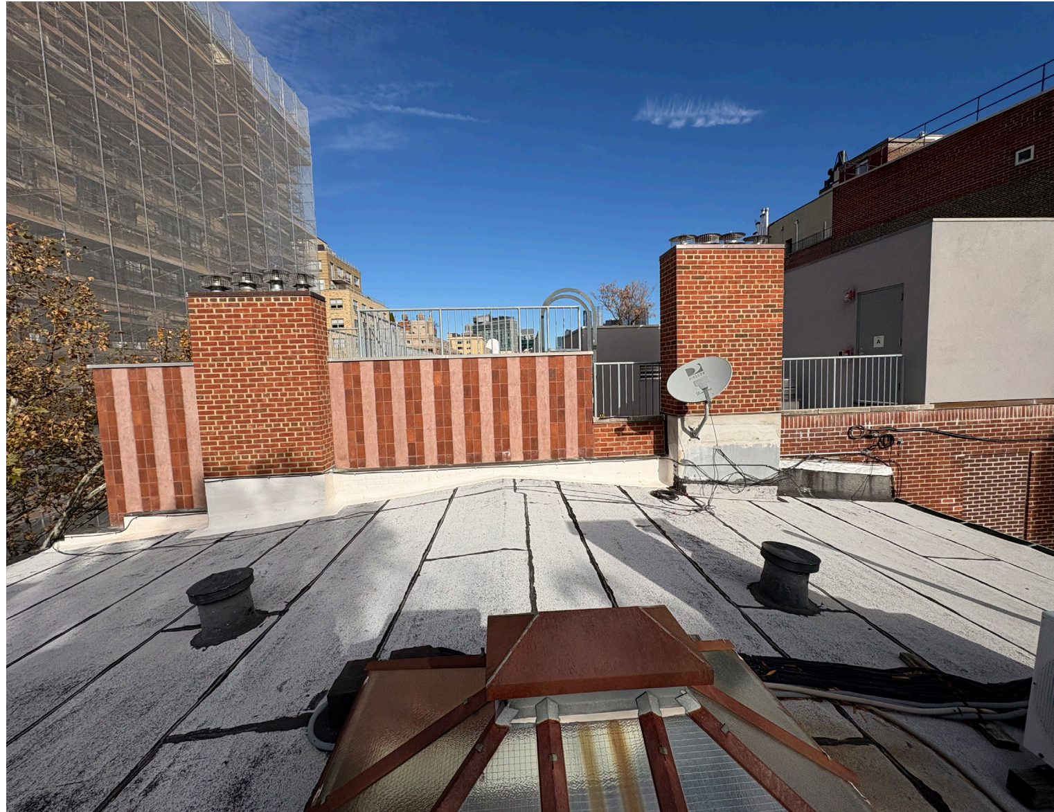
View of the roof - looking north
