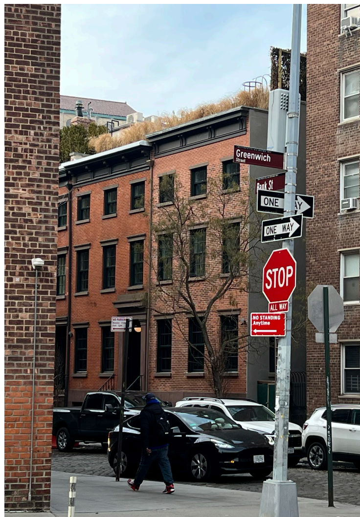
105-107 Bank Street (2022 Approval), Primary Facade
