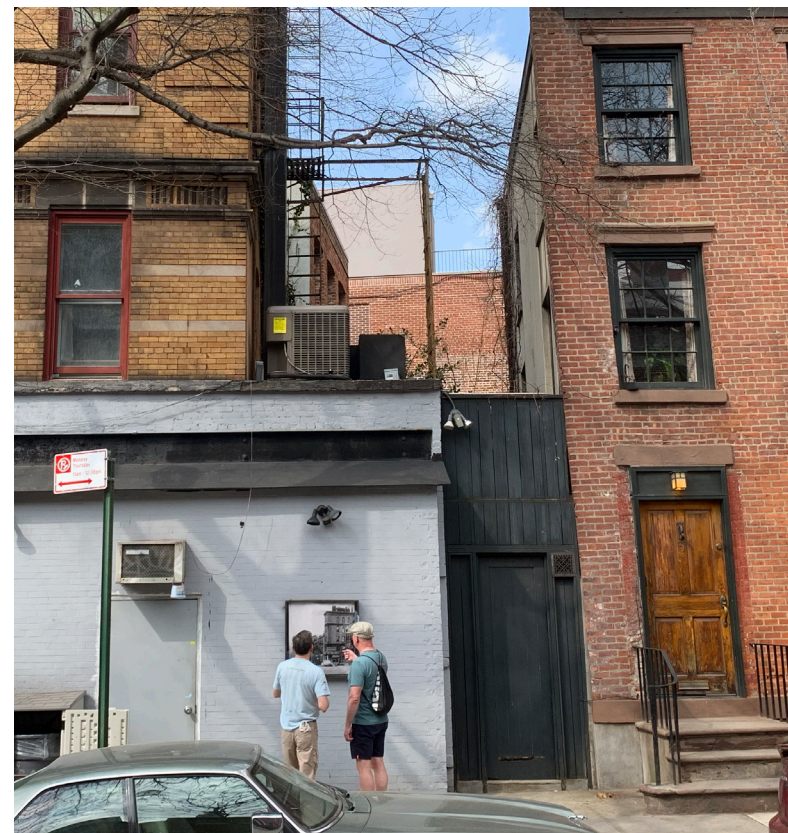
Addition is not visible from further west along Bank Street
