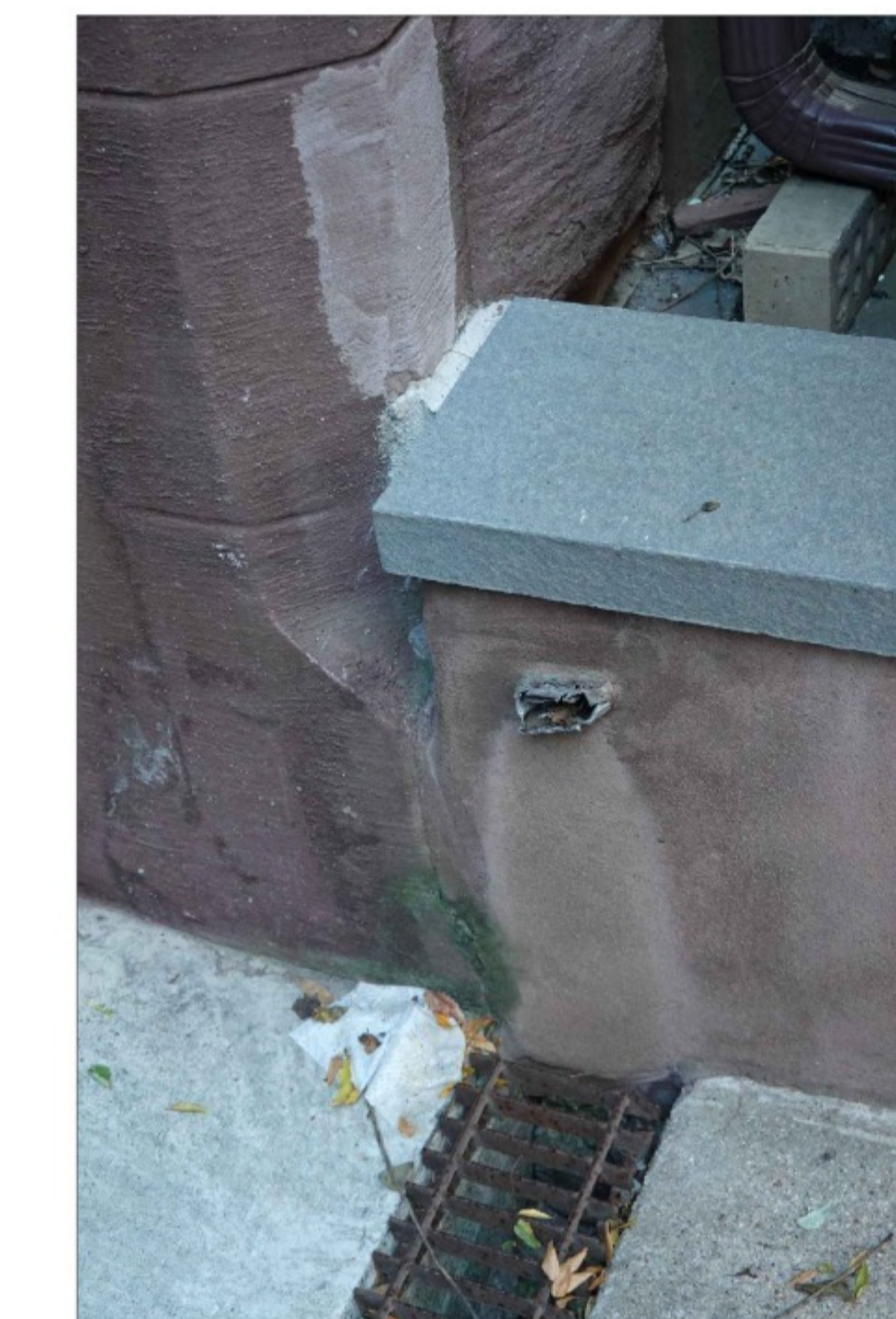
DRAINAGE CONDITION @ DRIVEWAY MKCA RECORDS 20
