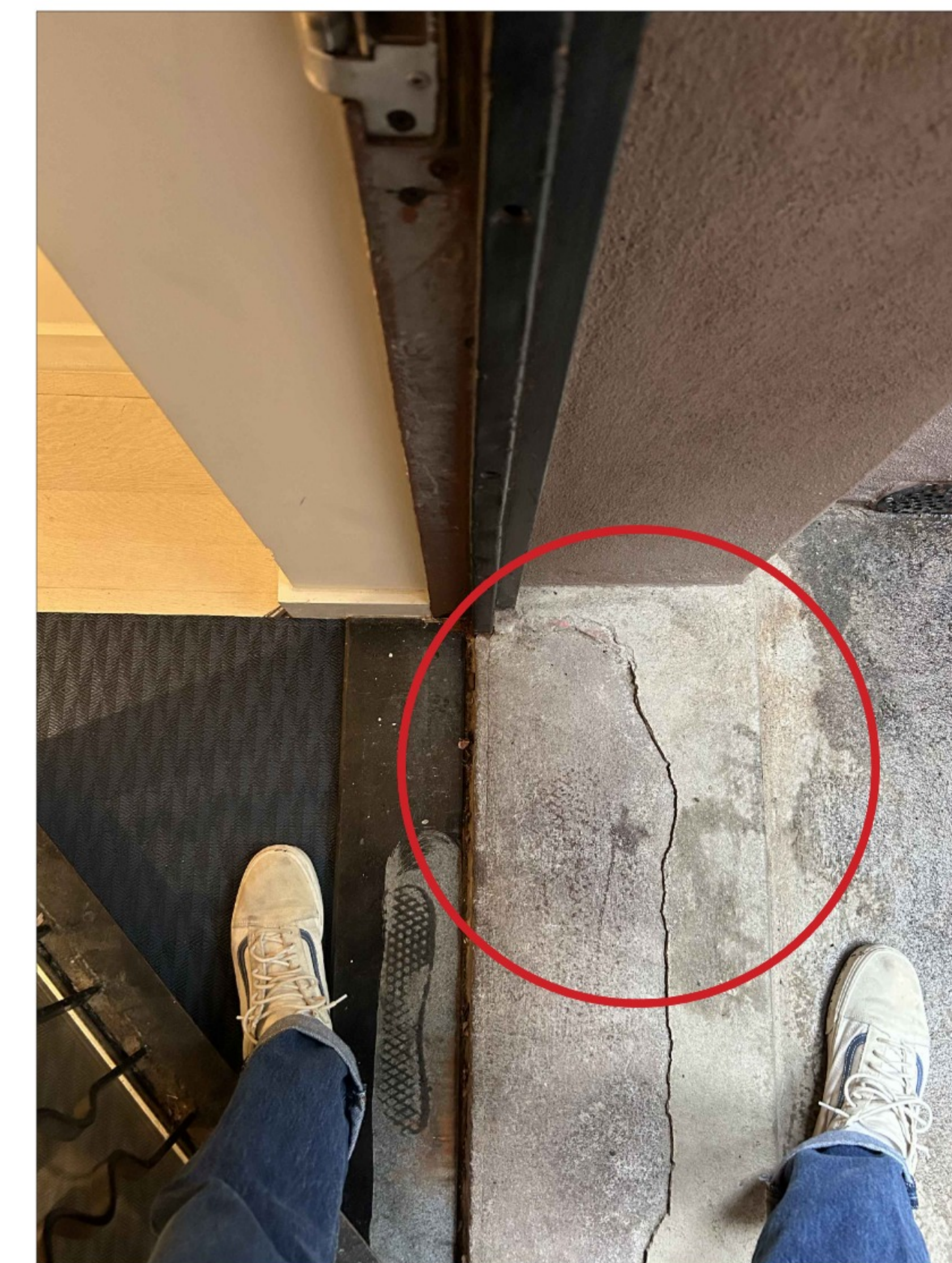
CRACKS IN STEPS AND THRESHOLD MKCA RECORDS 10
