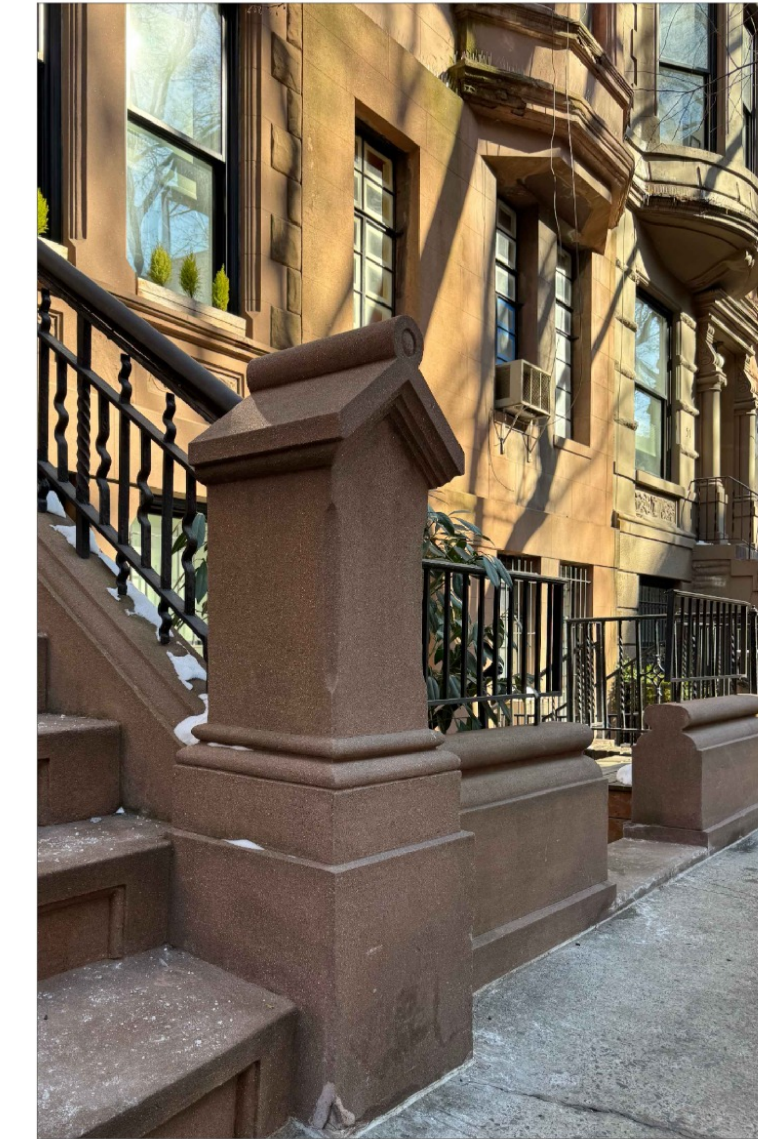
EXISTING CONCRETE RETAINING WALL & RAILING RETURN @ 55 W 90TH ST MKCA RECORDS 30
