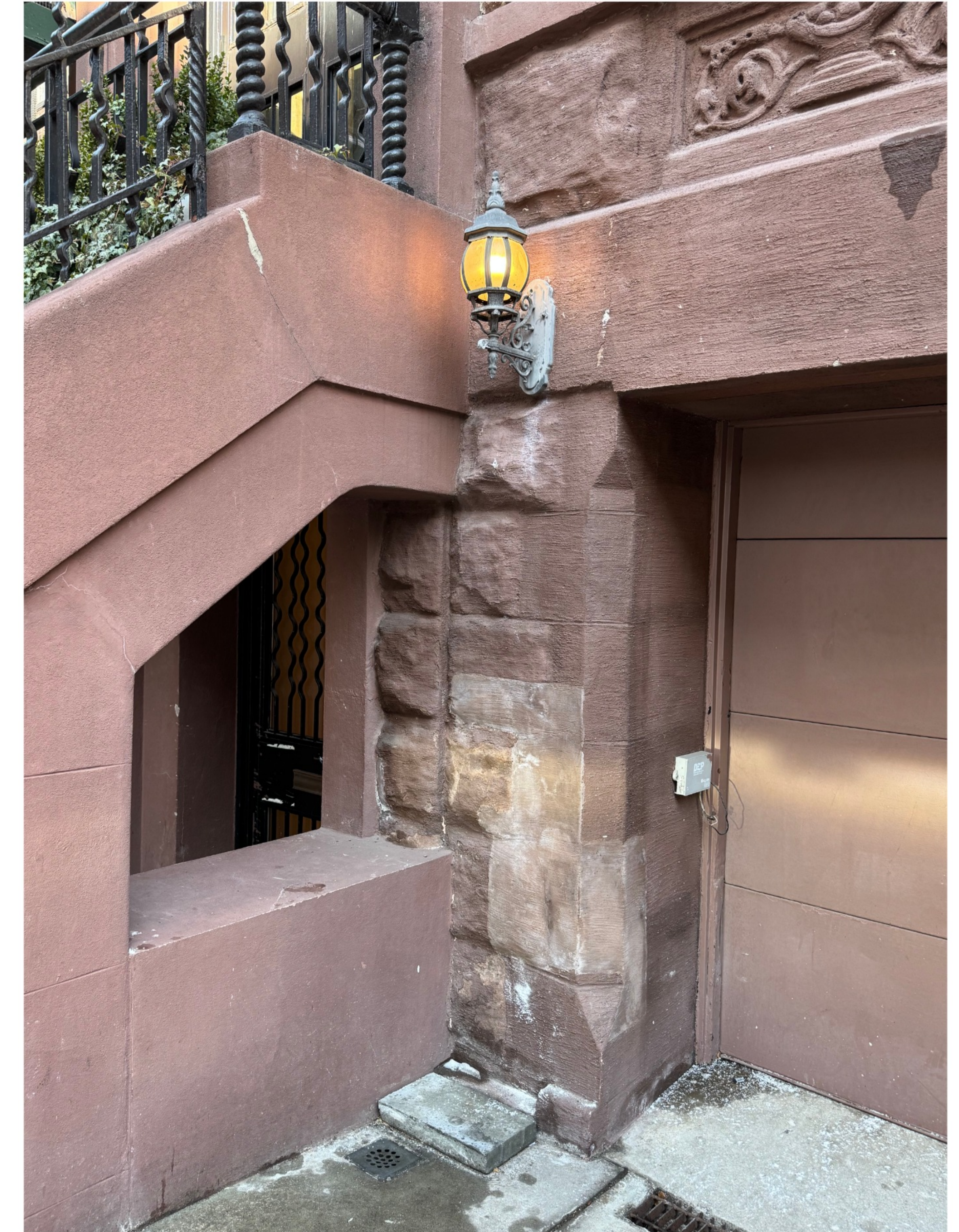
ALL SURFACES ARE STUCCO (NO ORIGINAL BROWNSTONE)
