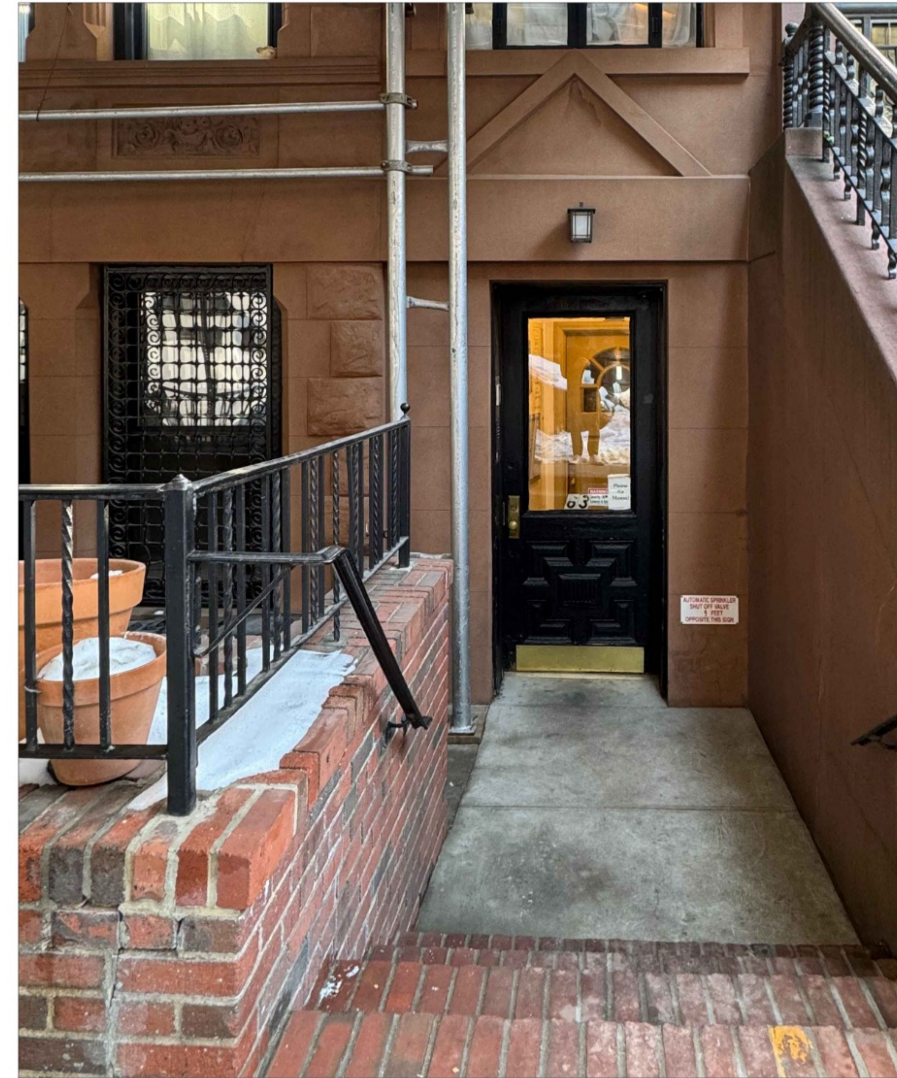
EXISTING CONCRETE RETAINING WALL & RAILING RETURN @ 63 W 90TH ST MKCA RECORDS 50
