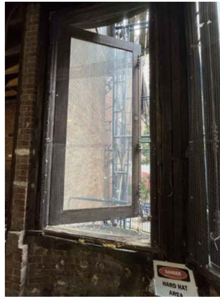
EXISTING CONDITION W28, W29 PHOTO (DATE TAKEN: SEPTEMBER 10TH, 2025)
