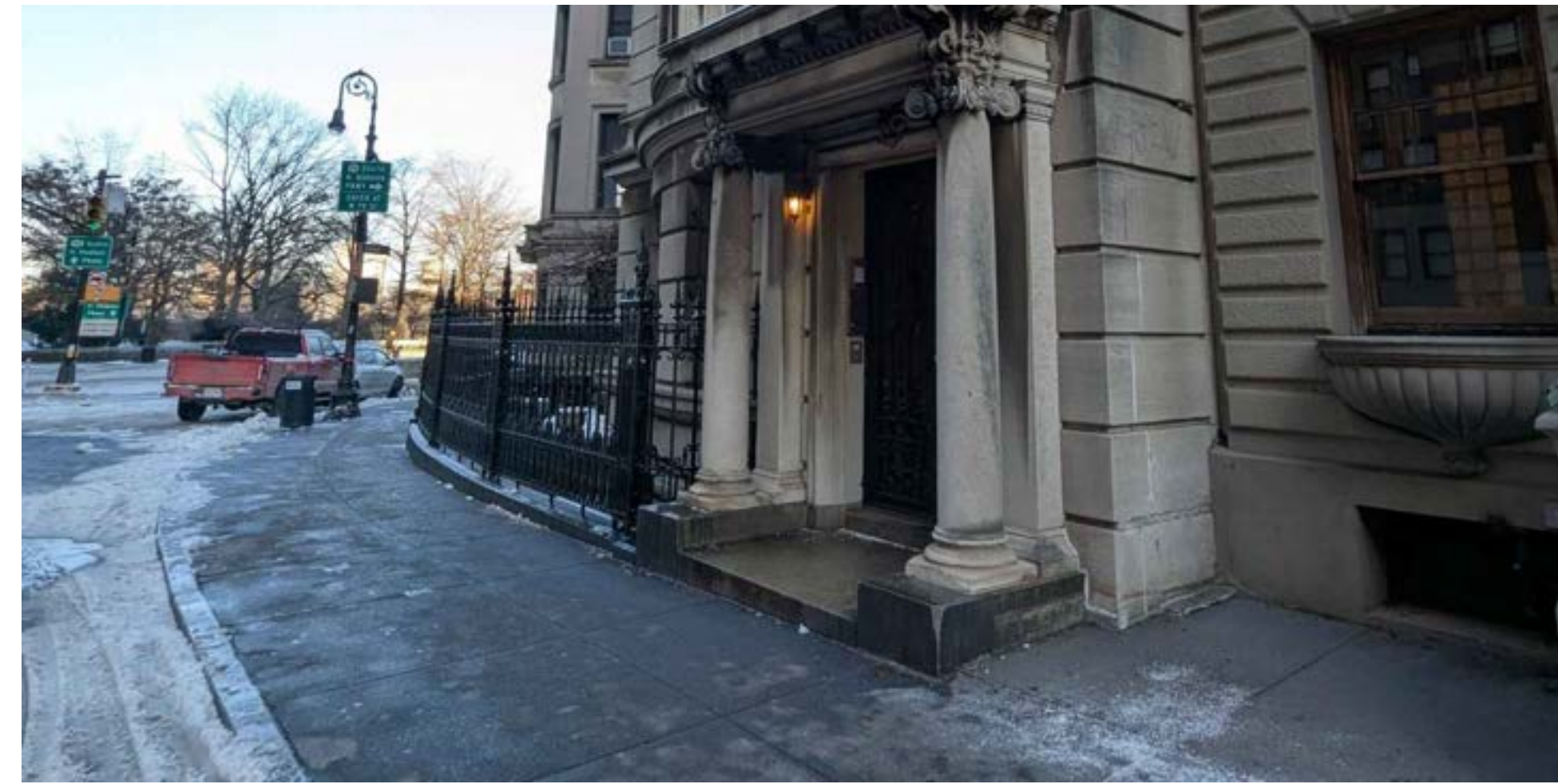
FENCE AND FRONT YARD PROTRUDING ON SIDEWALK
