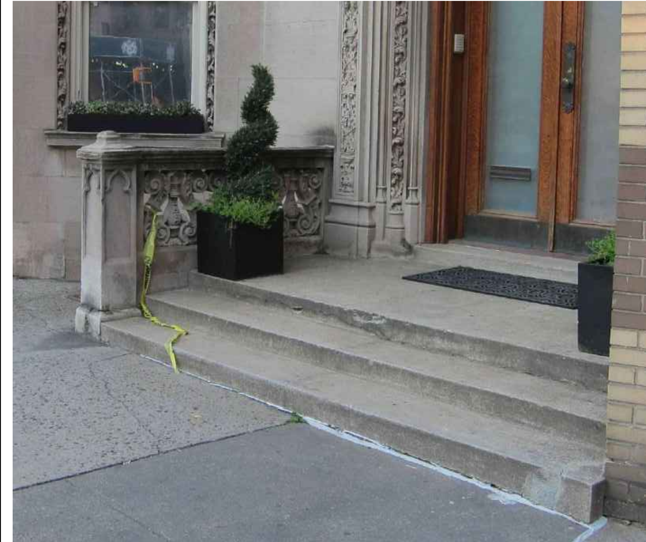
1 DEMOLISHED STONE NEWEL POST AND ORNATE BALUSTRADES SCALE: 3/8" = 1'-0"
