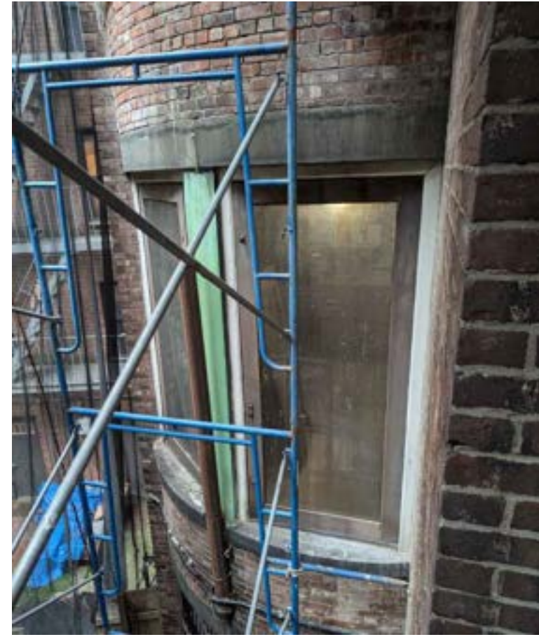
EXISTING CONDITION W28, W29 PHOTO (DATE TAKEN: OCTOBER 28TH, 2024)
