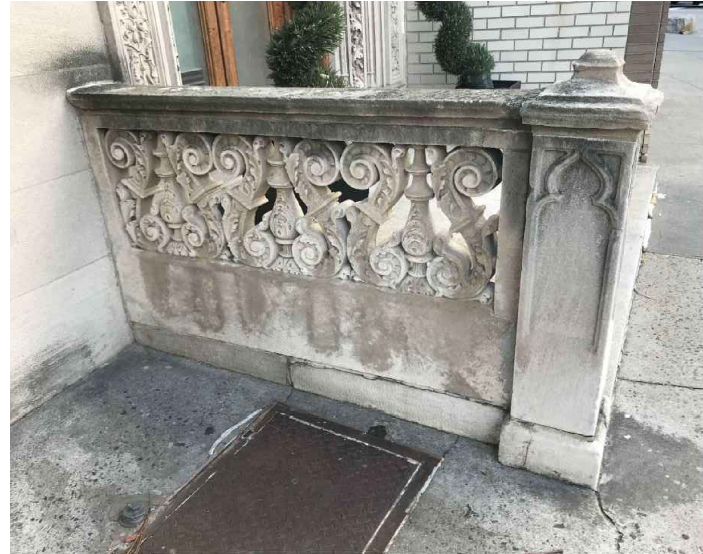
2 DEMOLISHED STONE NEWEL POST AND ORNATE BALUSTRADES SCALE: 3/8" = 1'-0"
