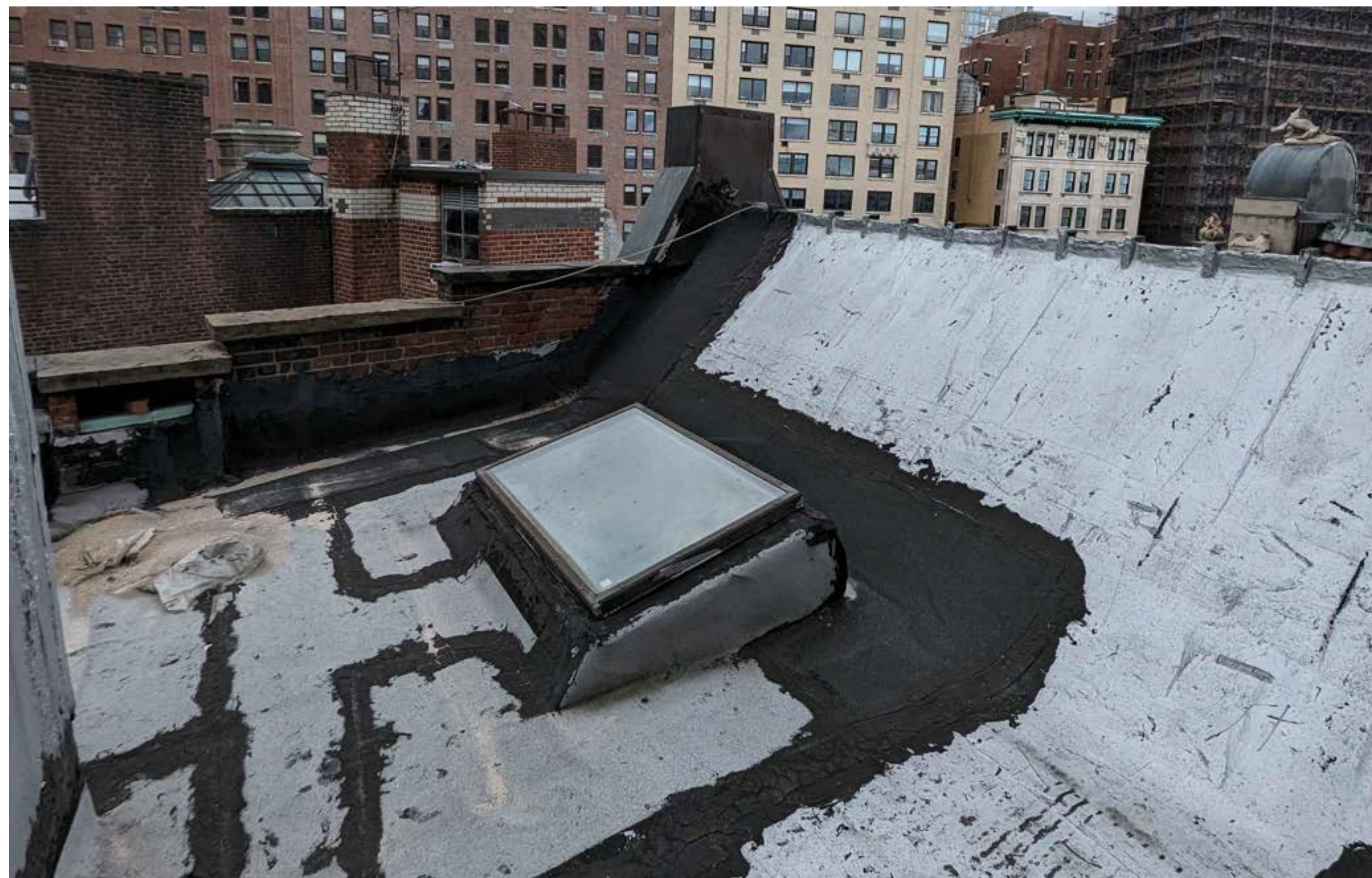
3 PHOTO OF EXISTING ROOF CONDITION SCALE: N.T.S.
