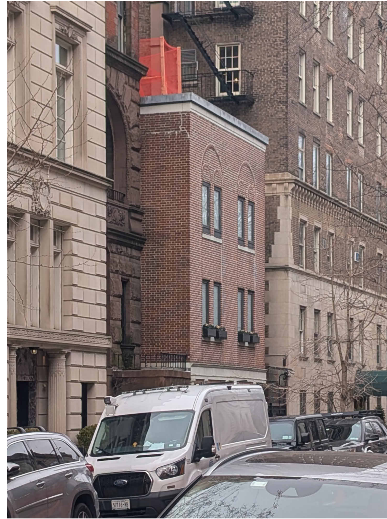
MOCKUP PHOTO: FROM NORTHEAST ON E 78TH STREET
