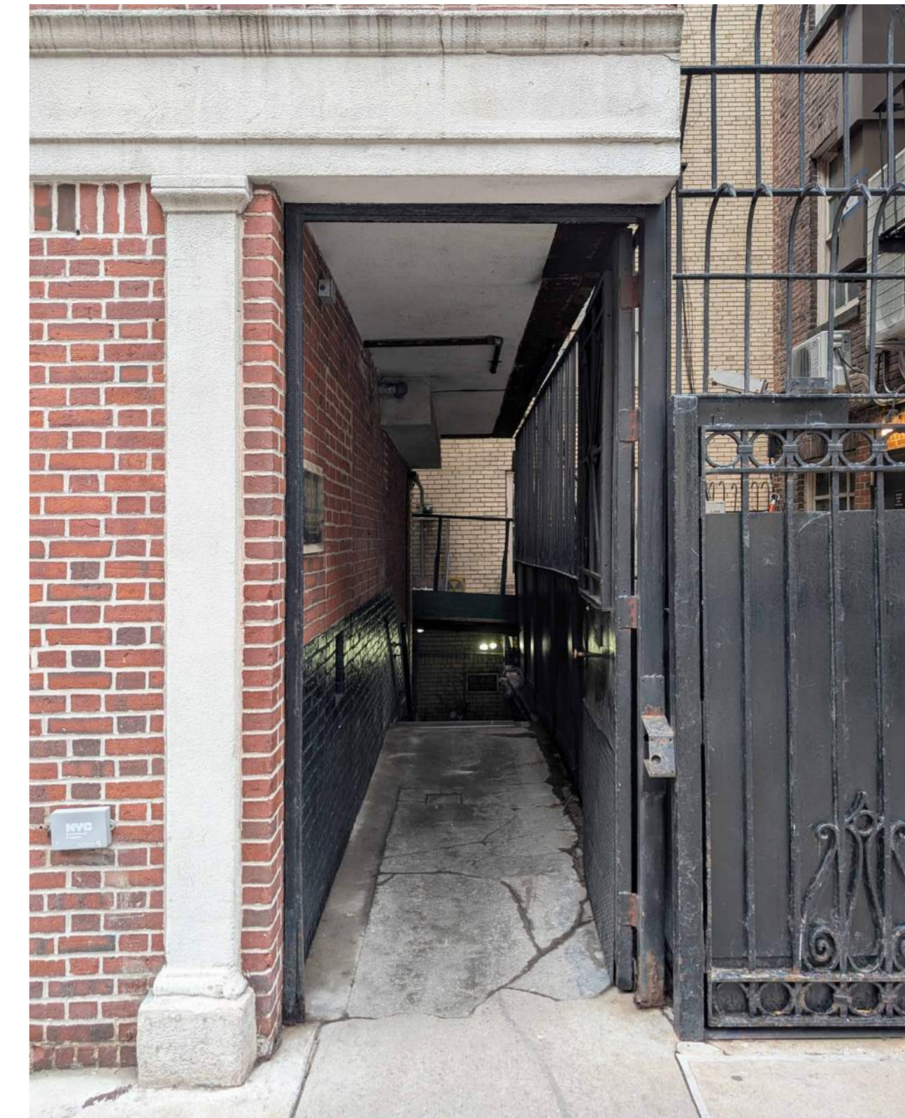
VIEW OF EXISTING SERVICE PASSAGEWAY FROM STREET
