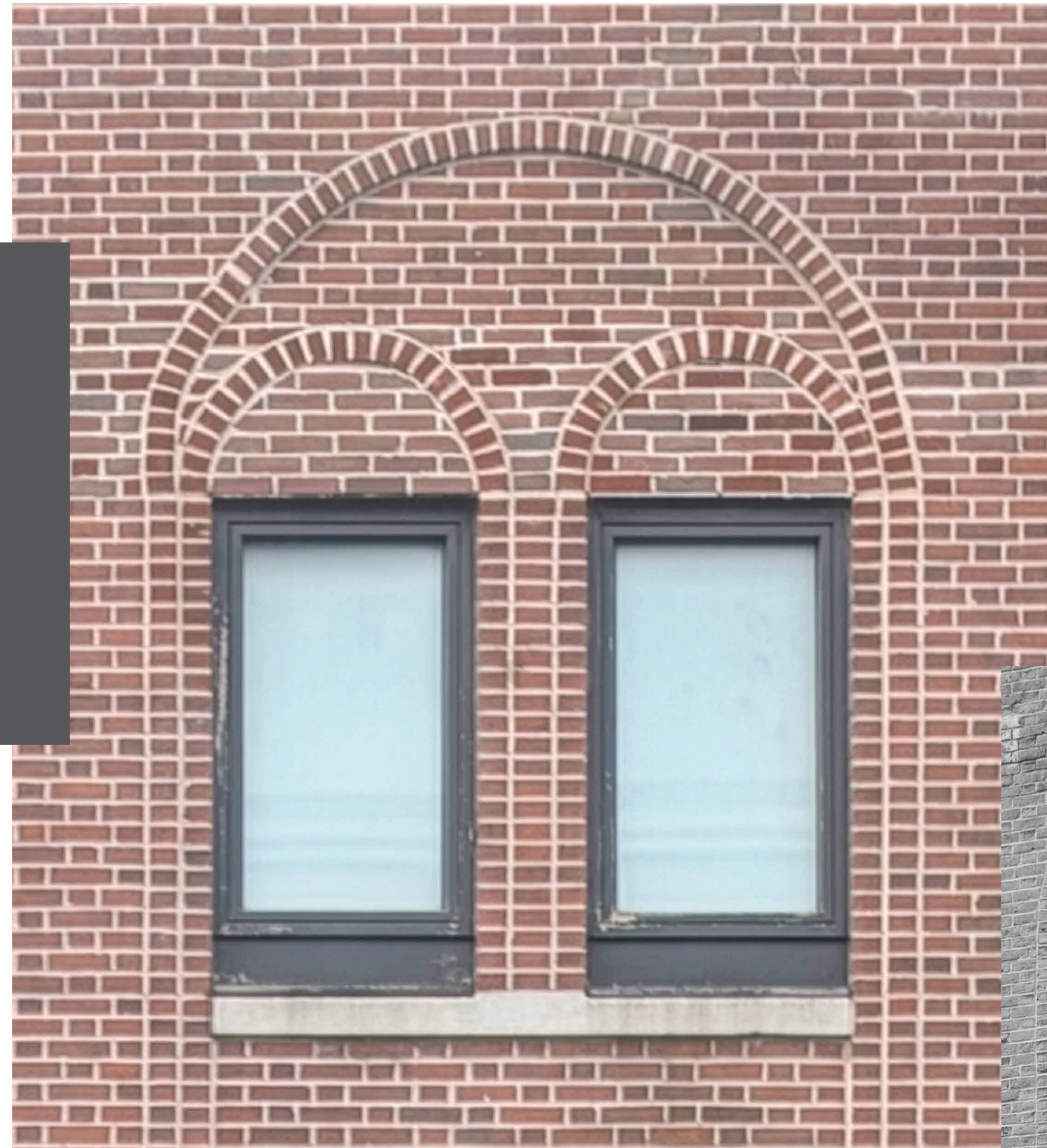
RESTORE EXISTING BRICK, REPLACE EXISTING WINDOWS AT THIRD FLOOR TO MATCH HISTORIC PHOTOS [BLACK FINISH]
