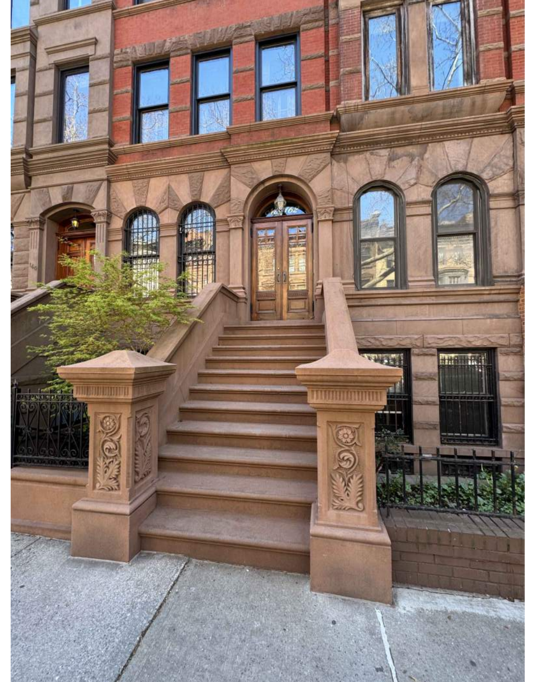
162 W 88TH STREET NEIGHBORING STOOP, REPRESENTATIVE OF THE STANDARD CONFIGURATION FOR THE THREE REMAINING STOOPS IN THE ROW, ALL DESIGNED BY GILBERT A SCHELLENGER.
