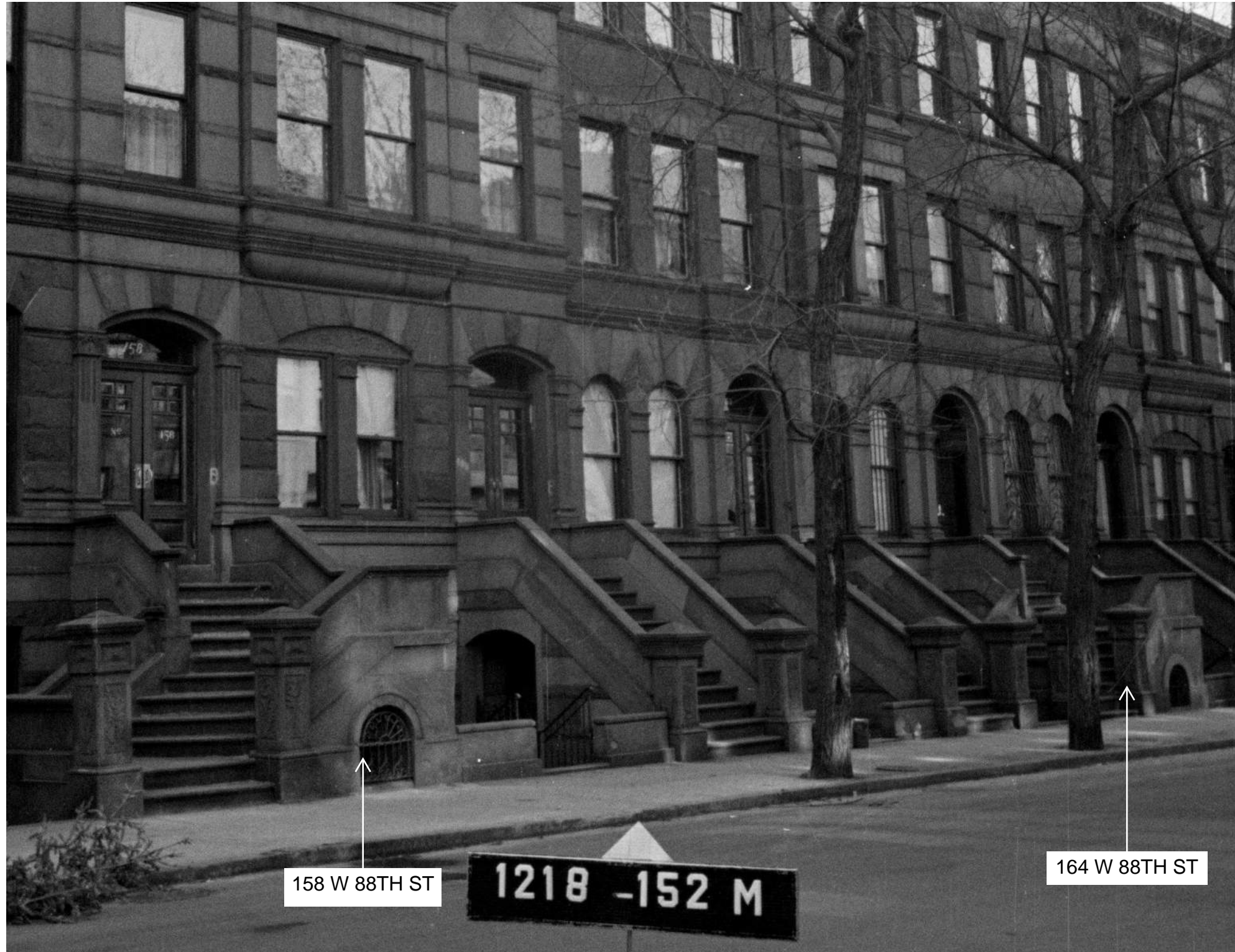
HISTORIC TAX LOT PHOTOGRAPH DEPICTING THE ONLY TWO DOG-LEG STOOPS ON WEST 88TH ST (BLOCK 1218).
