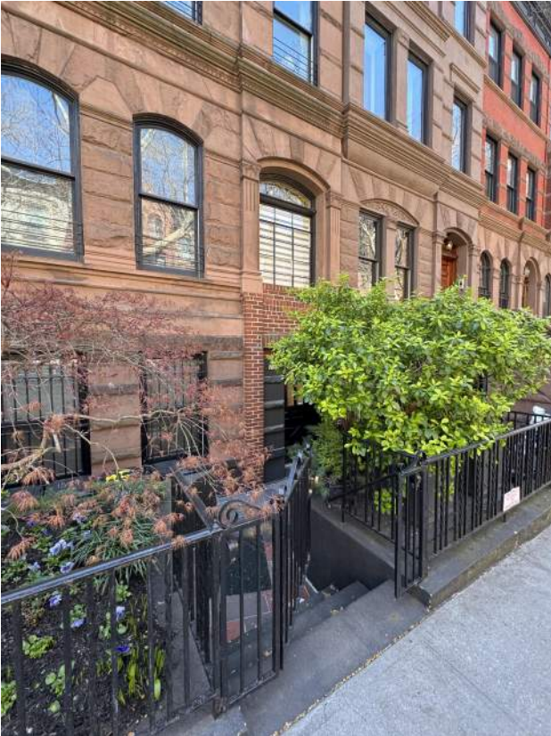
158 W 88TH STREET DOG-LEG STOOP REMOVED PRIOR TO LANDMARK DESIGNATION
