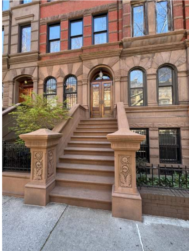
162 W 88TH STREET EXISTING STRAIGHT STOOP
