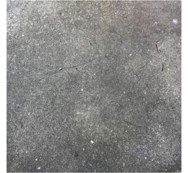
EXISTING CONCRETE PAVING IN AREAWAY (TO BE REMOVED)
