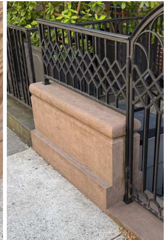
PROFILE OF BROWNSTONE FENCE AND IRON FENCE AT 160 W 88TH ST
