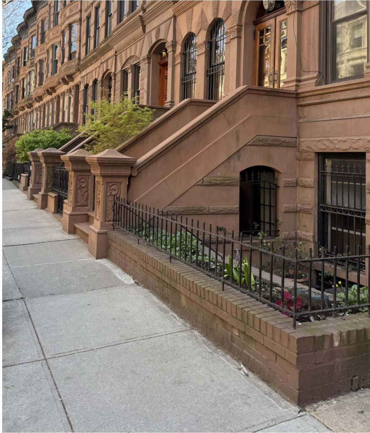
EXISTING CONCRETE SIDEWALK
