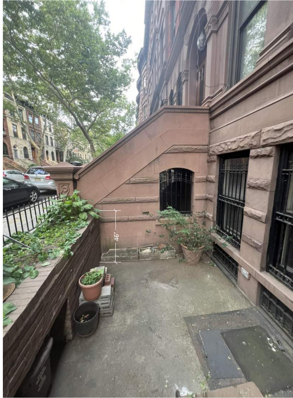
EXISTING FRONT AREAWAY
