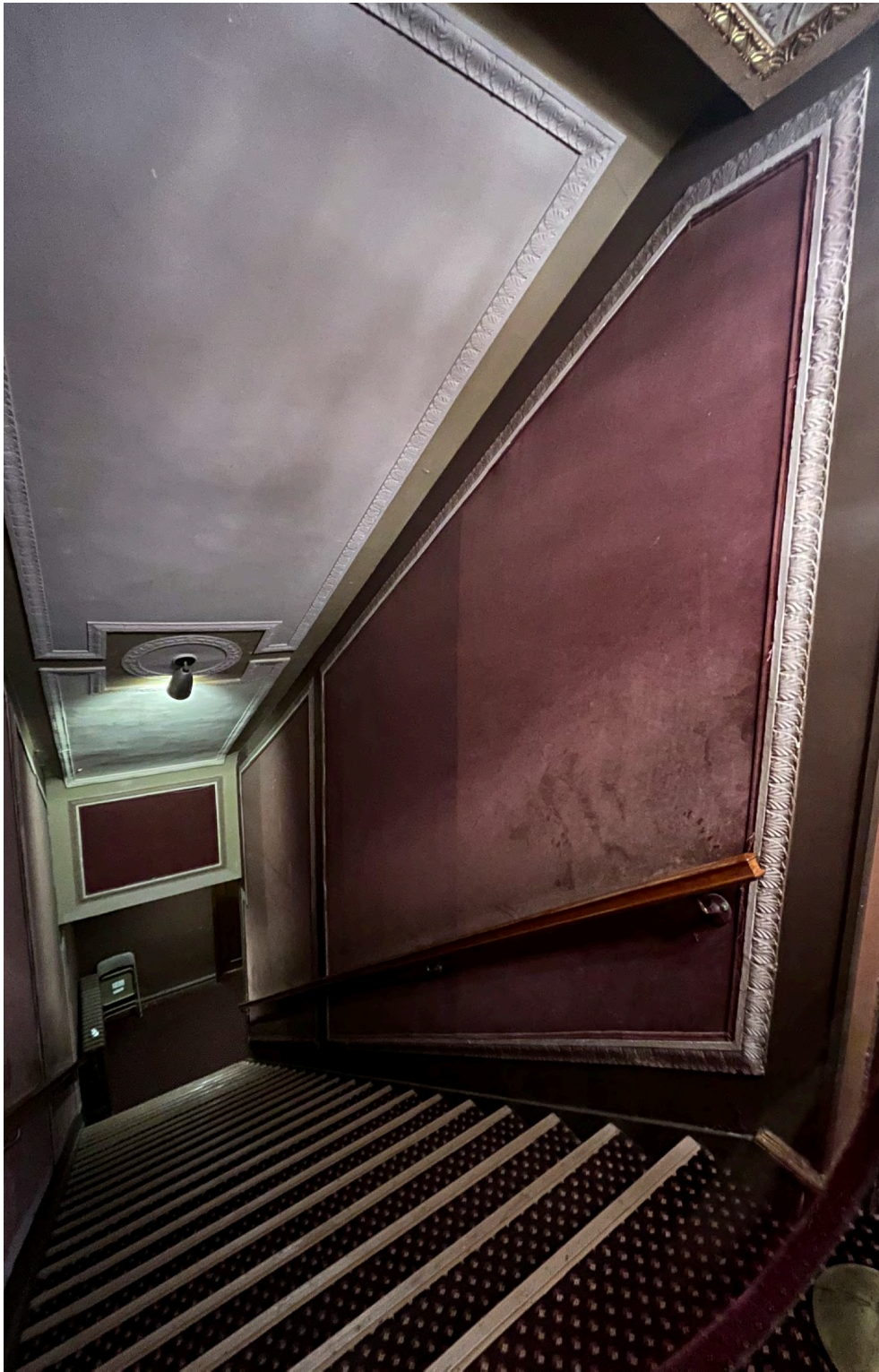
Existing House Left Stair
