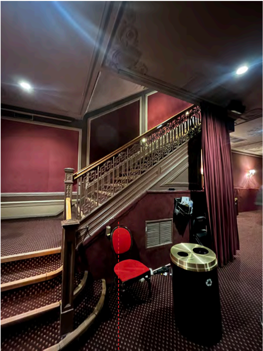
Existing House Right Stair
