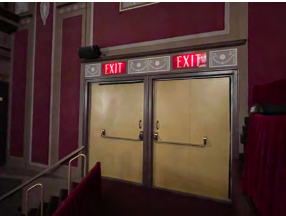
Existing House Right Emergency Doors
