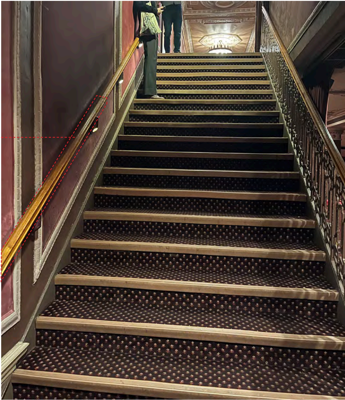
Photo looking up the House Right Stair
