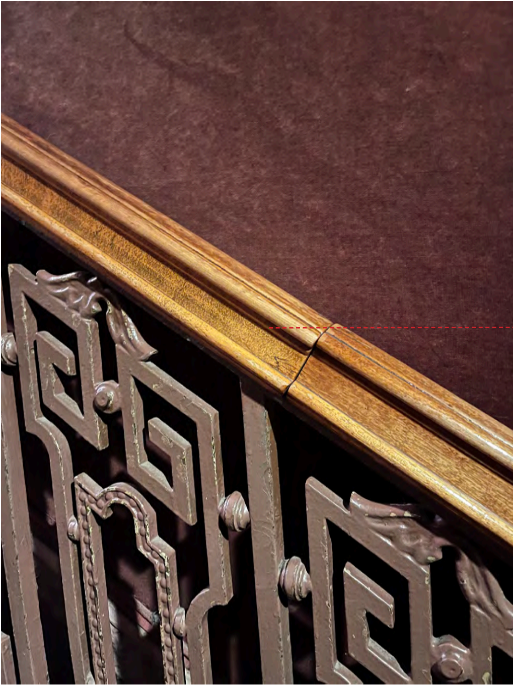
Close-up of the House Right Wood Cap above the decorative metal railing
