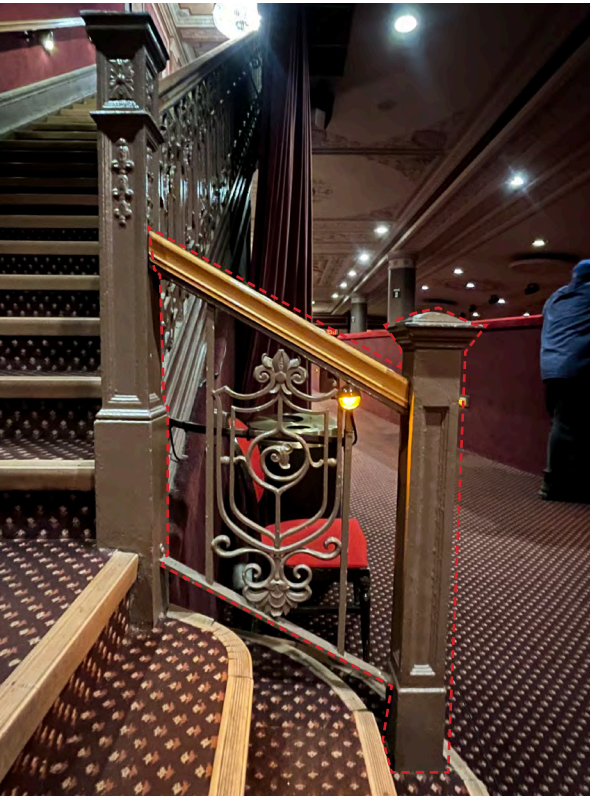
Lower portion of railing will not be reused
