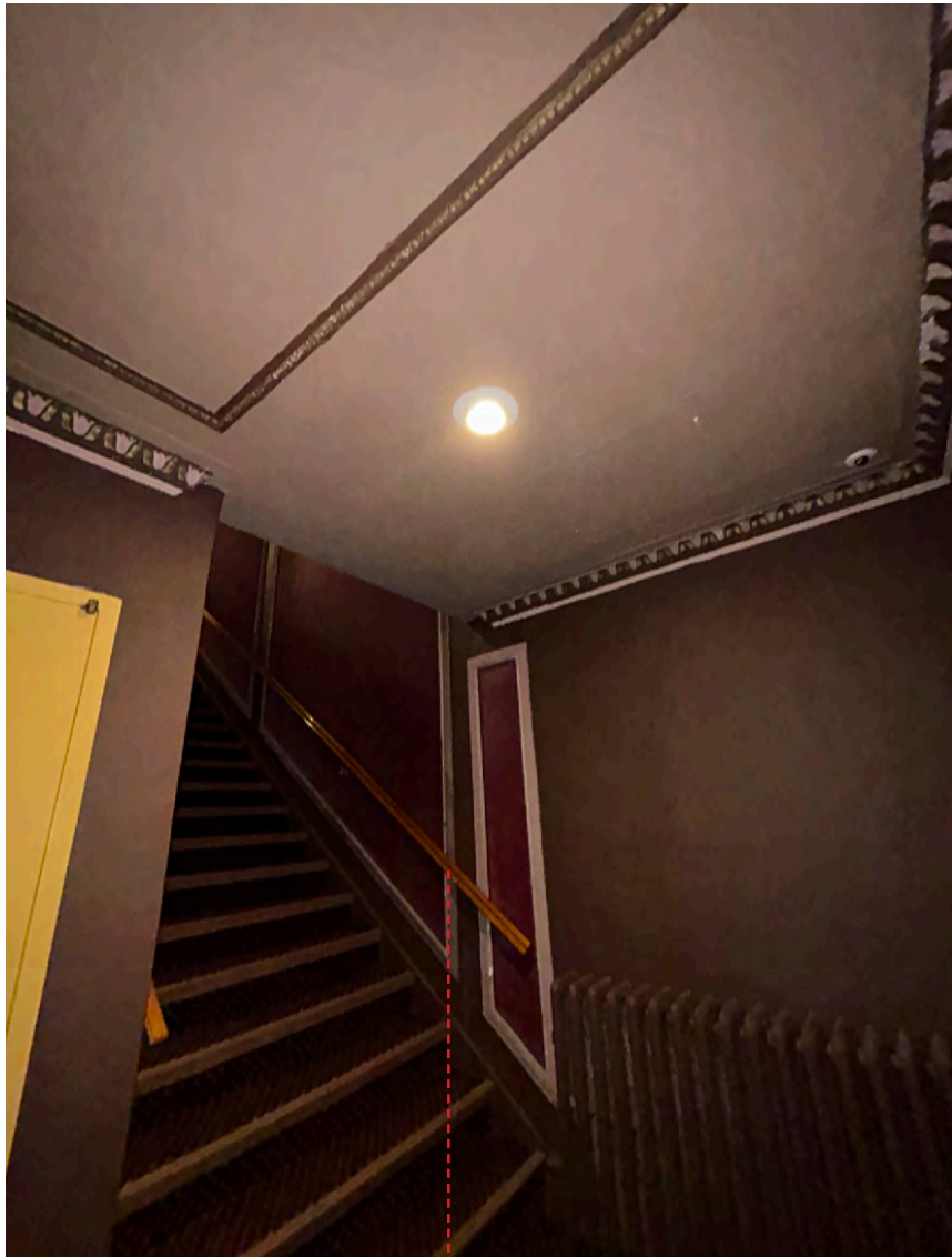
Existing House Left Stair
