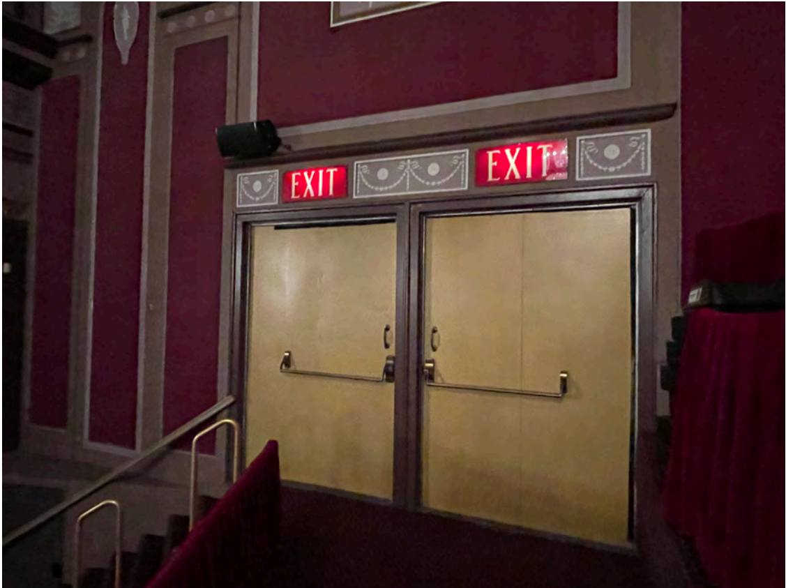
Existing Balcony House Right Emergency Doors
