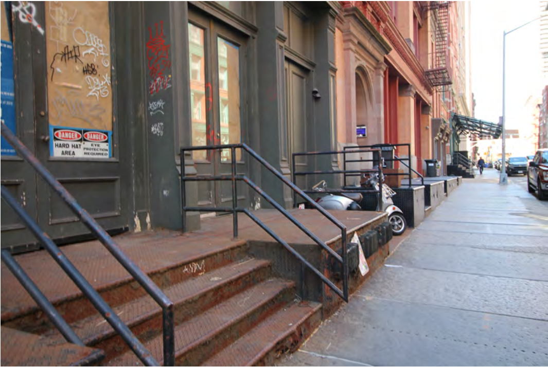
CONTEMPORARY SIDEWALK PHOTO #3 - EXISTING DIAMOND PLATE DOCKING & HISTORIC GRANIT SLAB SIDEWALK
