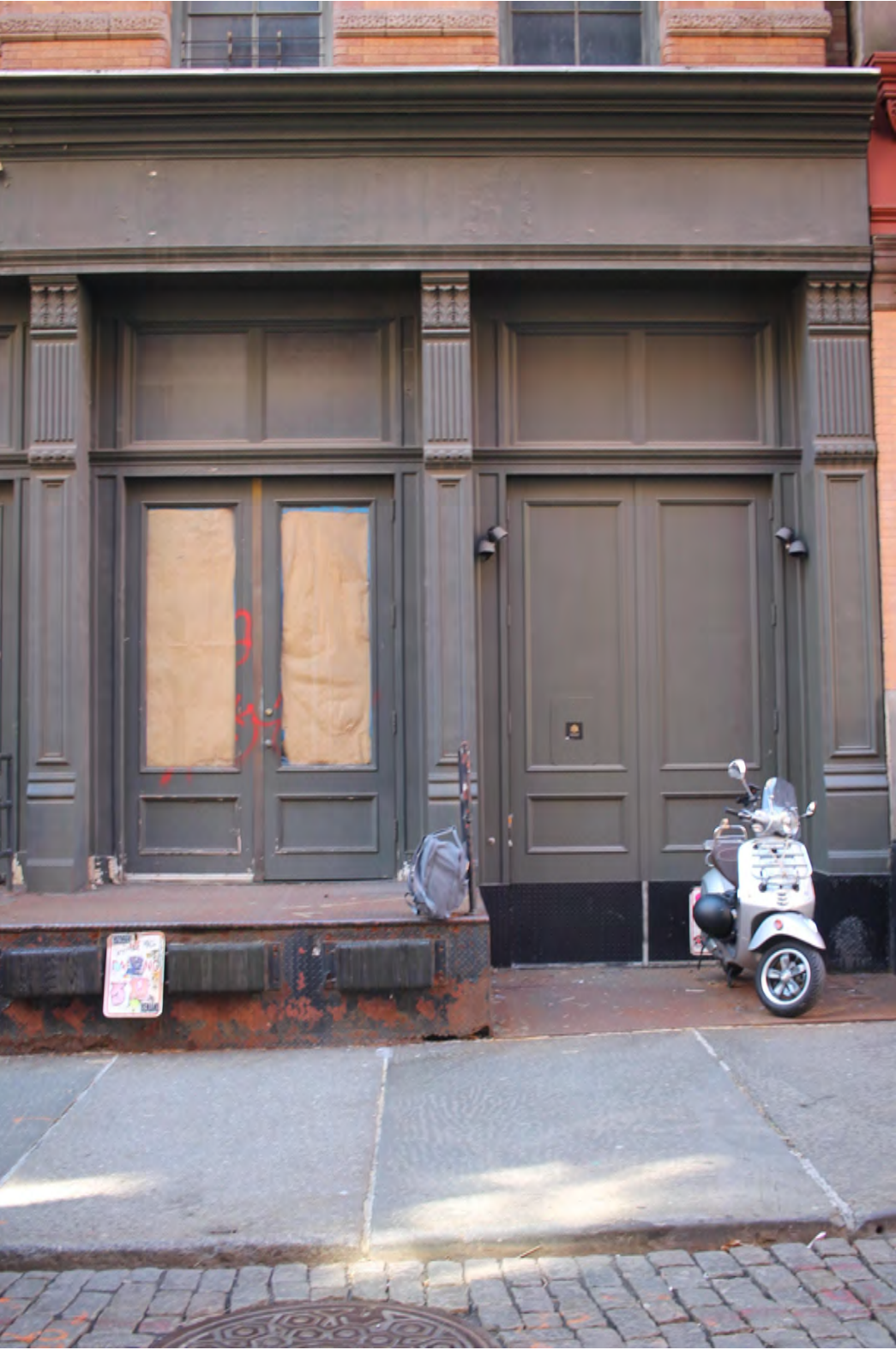
CONTEMPORARY SIDEWALK PHOTO #1 GROUND-LEVEL BUILDING ENTRY WITH FLUSH STEEL DIAMOND-PLATE THRESHOLD AT SIDEWALK GRADE
