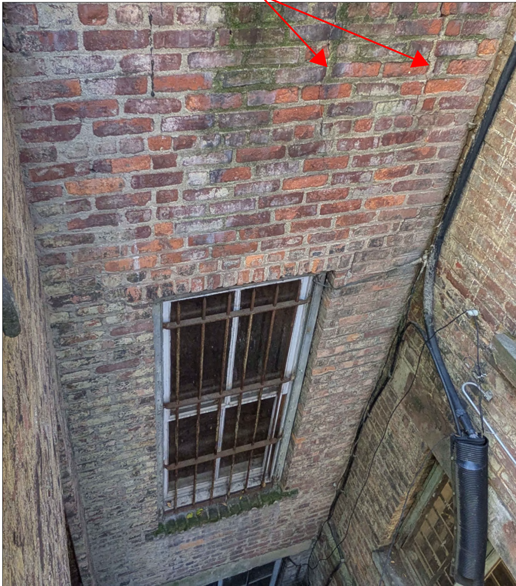
LIGHTWELL ADJACENT TO ORIGINAL REAR FACADE; CONFIGURATION DIRECTS STORM DRAINAGE INTO CELLAR AREAWAY - NOTE VERTICAL CRACKING THROUGH SEVERAL COURSES OF BRICK
