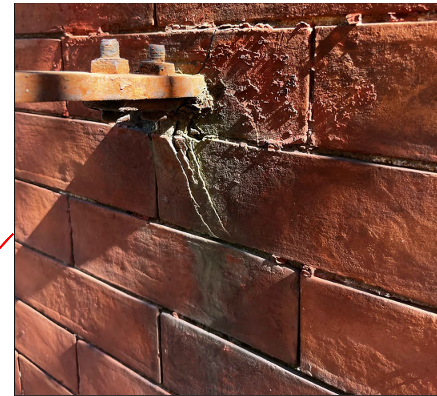
DAMAGED BRICK & RUSTING AT FIRE ESCAPE ATTACHMENT POINTS
