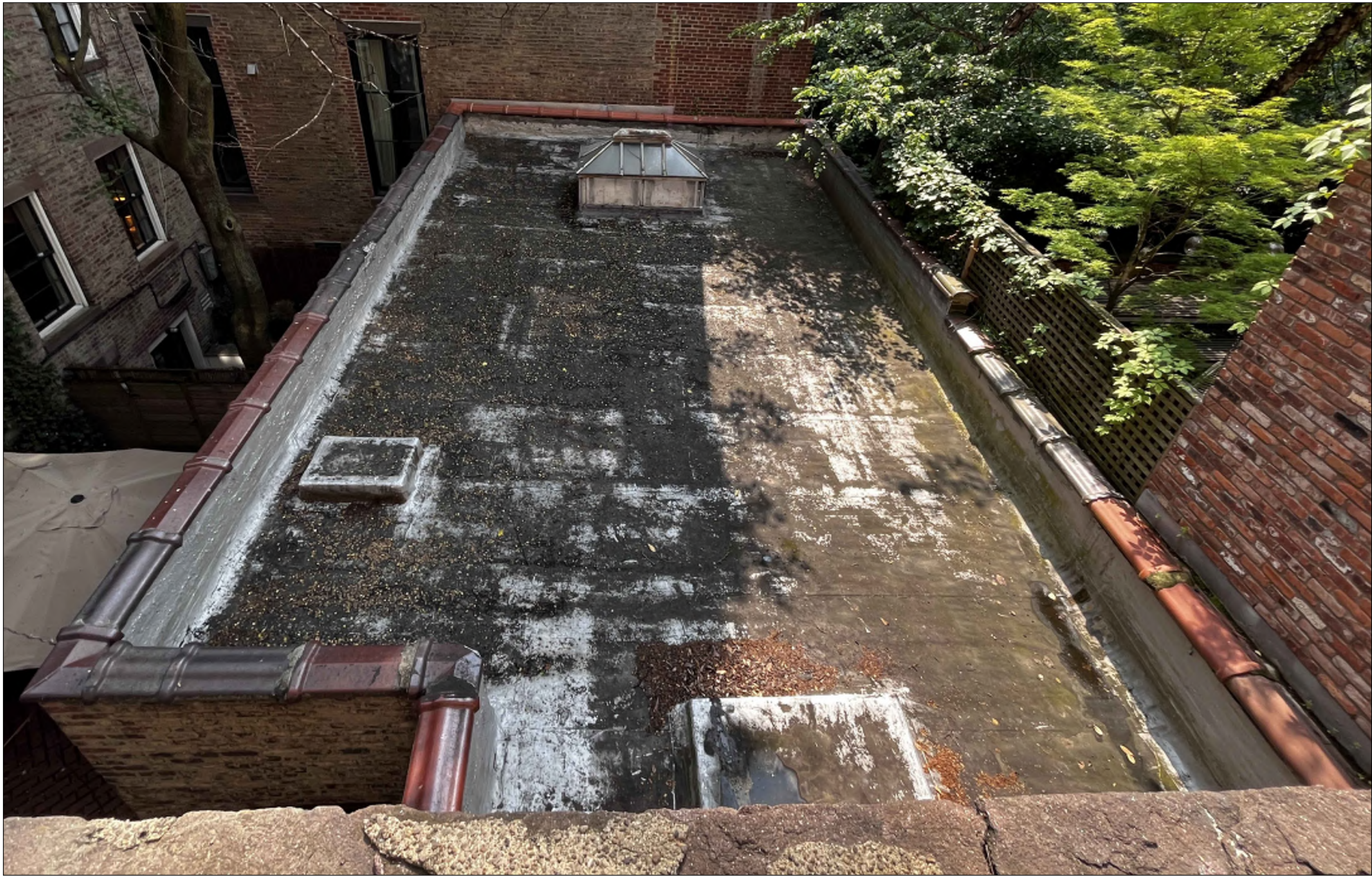
LIGHTWELL ADJACENT TO ORIGINAL REAR FACADE; CONFIGURATION DIRECTS STORM DRAINAGE INTO CELLAR AREAWAY - NOTE VERTICAL CRACKING THROUGH SEVERAL COURSES OF BRICK
