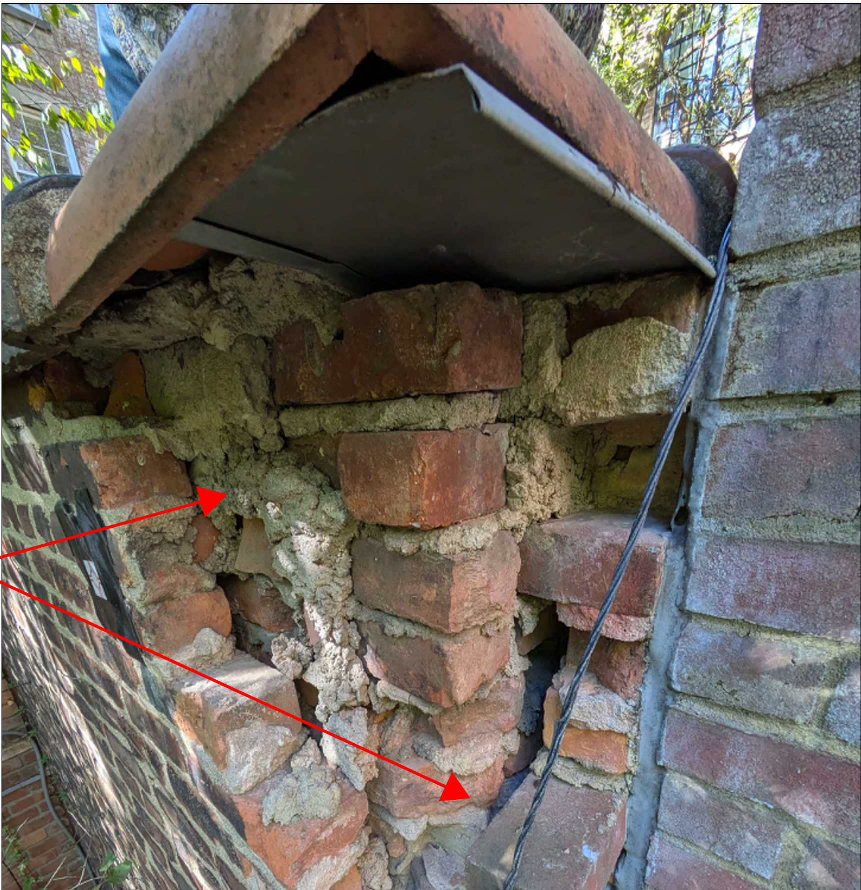
EXISTING AREAS OF REMOVAL AT EAST FACADE REVEAL A RUDIMENTARY TWO WYTHER WALL ASSEMBLY WITH LARGE VOIDS AT THE SLUSH JOINTS.
