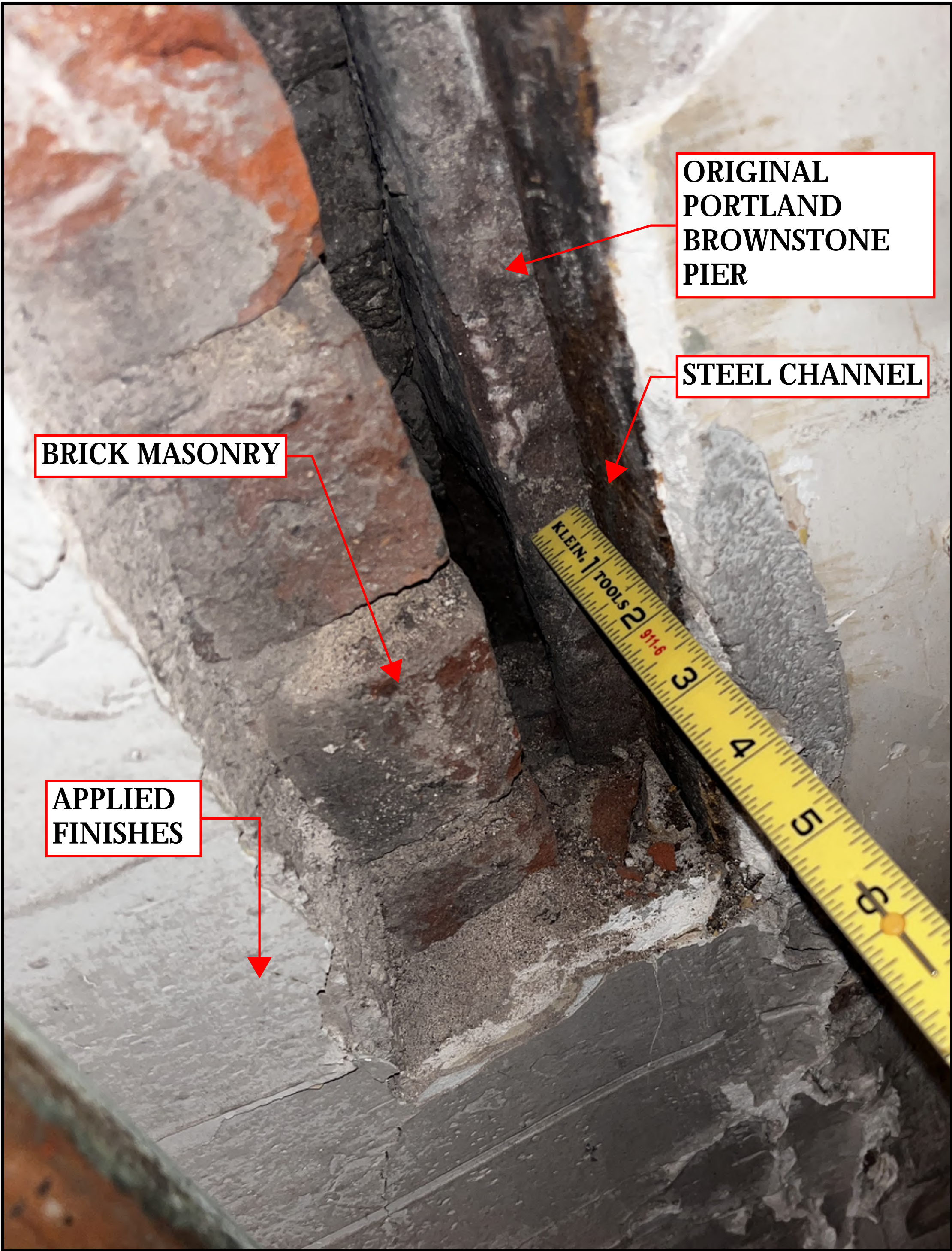
PROBE THROUGH APPLIED FINISHES REVEALS ORIGINAL PORTLAND BROWNSTONE PIER WITH LATER INTERIOR STEEL CHANNEL FOR STOREFRONT FINISHES.
