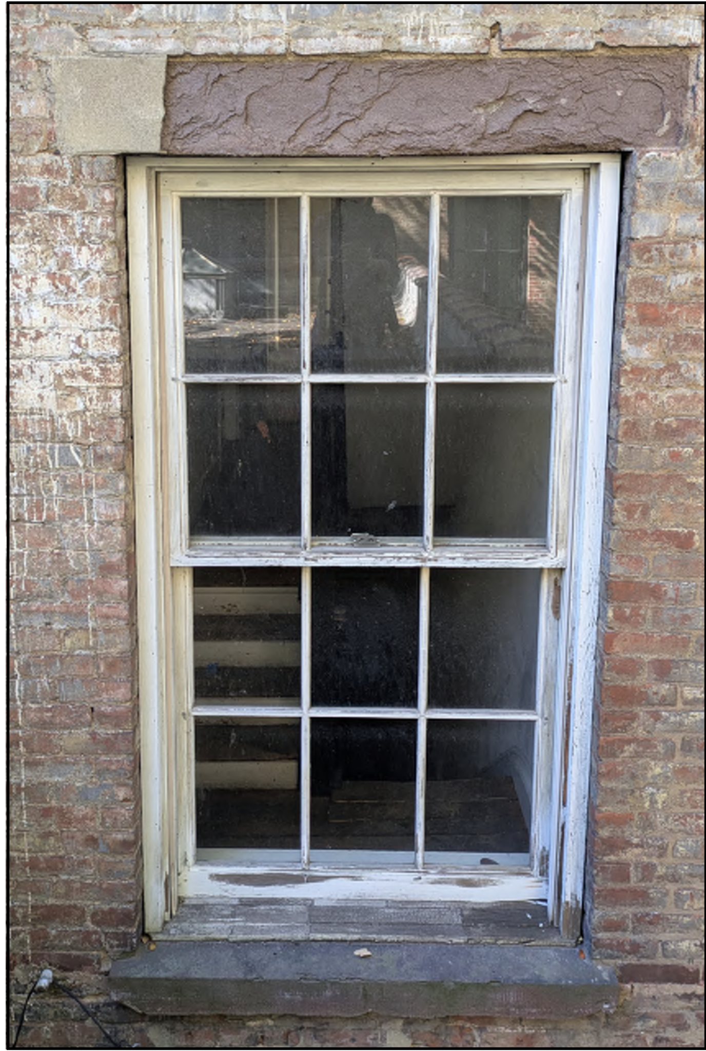
REAR FAÇADE – 2ND FLOOR STAIRWELL: NON-ORIGINAL 6-OVER-6 DOUBLE-HUNG WOOD WINDOW w/APPLIED EXTERIOR 'STORM' PANELS & FINGER-JOINTED CARPENTRY.
