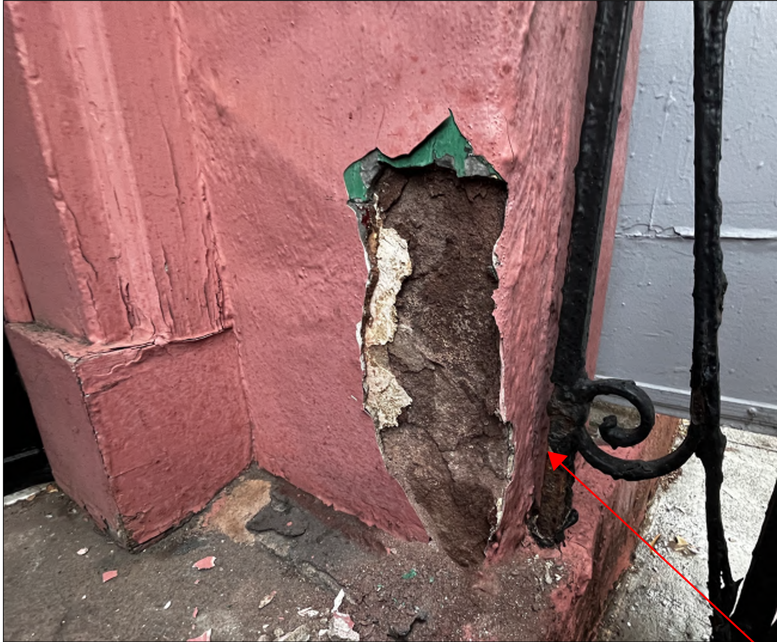
FRONT FAÇADE, GROUND FLOOR NORTH ENTRY – SOUTH PIER: REMOVAL OF NON-ORIGINAL PAINTED STUCCO REVEALS ORIGINAL PORTLAND BROWNSTONE PIER.
