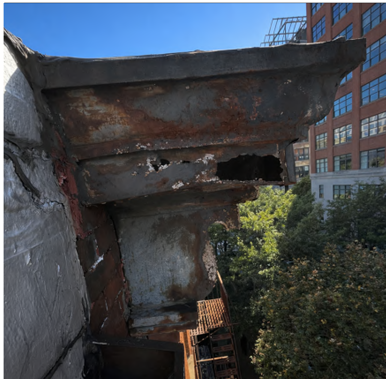
WIDESPREAD CORROSION & SECTION LOSS AT PAINTED GALVANIZED METAL CORNICE
