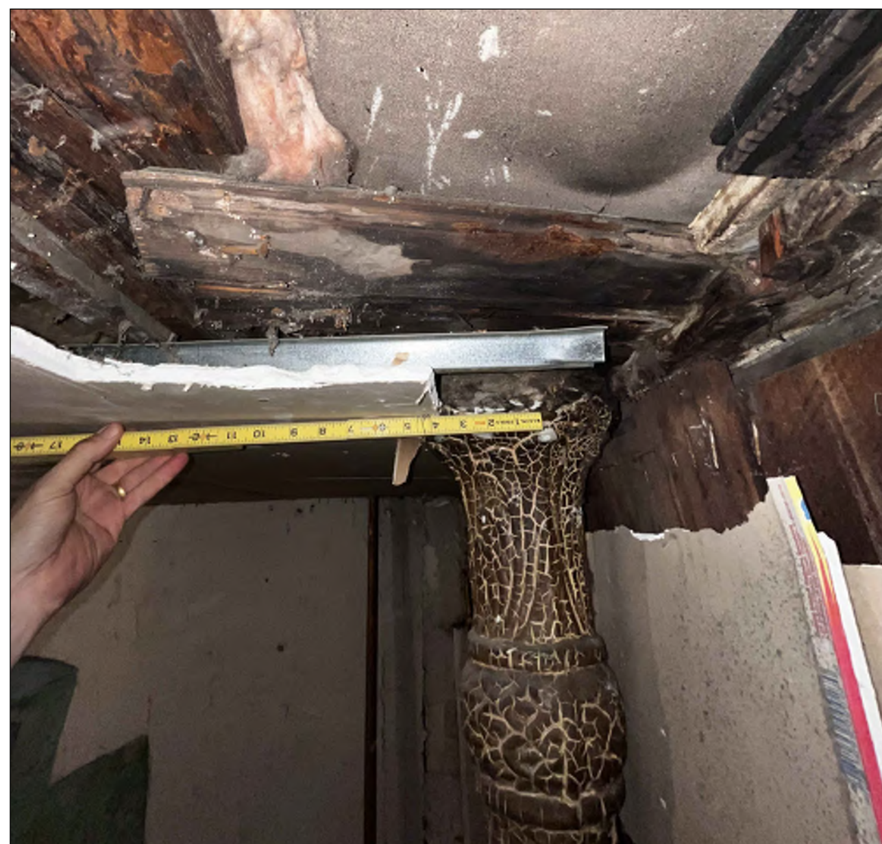
EXISTING CAST IRON COLUMNS SUPPORTING BROWNSTONE LINTEL BEHIND STUCCO FACADE
