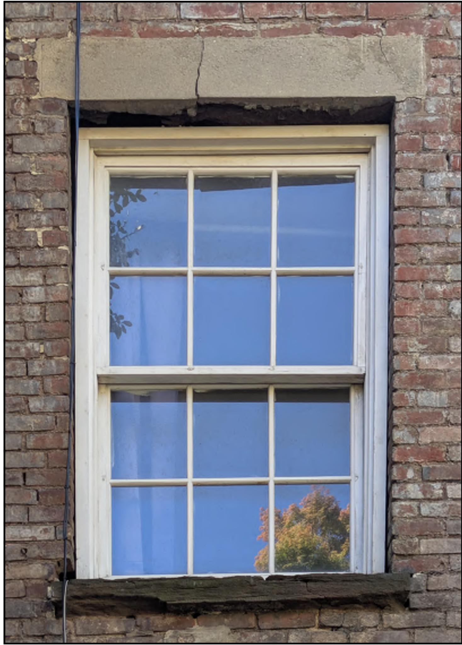
REAR FAÇADE – 3RD FLOOR STAIRWELL: NON-ORIGINAL 6-OVER-6 DOUBLE-HUNG WOOD WINDOW w/APPLIED EXTERIOR 'STORM' PANELS & FINGER-JOINTED CARPENTRY.
