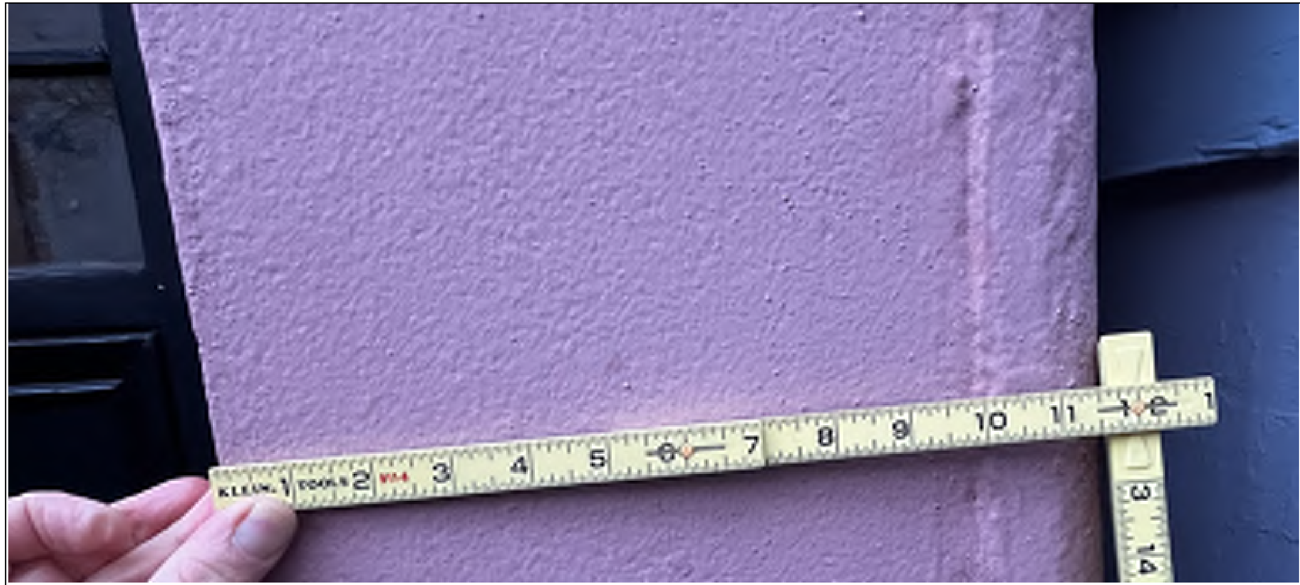
FRONT FAÇADE, GROUND FLOOR NORTH ENTRY – SOUTH PIER: 10" WIDE PIER IS INTACT THOUGH WILL LIKELY REQUIRE PARTIAL REPLACEMENT/RETOOLING.
