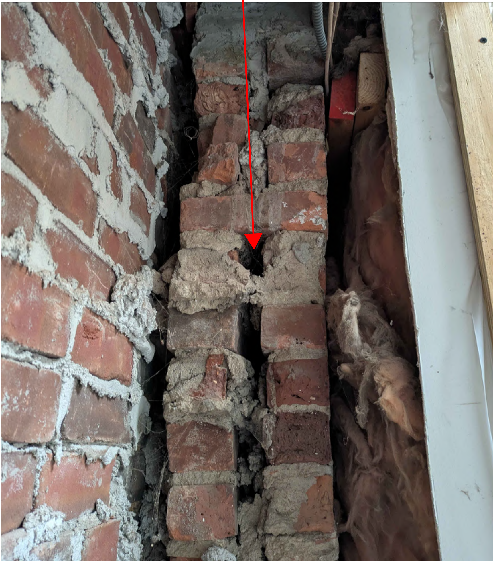
EXISTING AREAS OF REMOVAL AT EAST FACADE REVEAL A RUDIMENTARY TWO WYTHER WALL ASSEMBLY WITH LARGE VOIDS AT THE SLUSH JOINTS.
