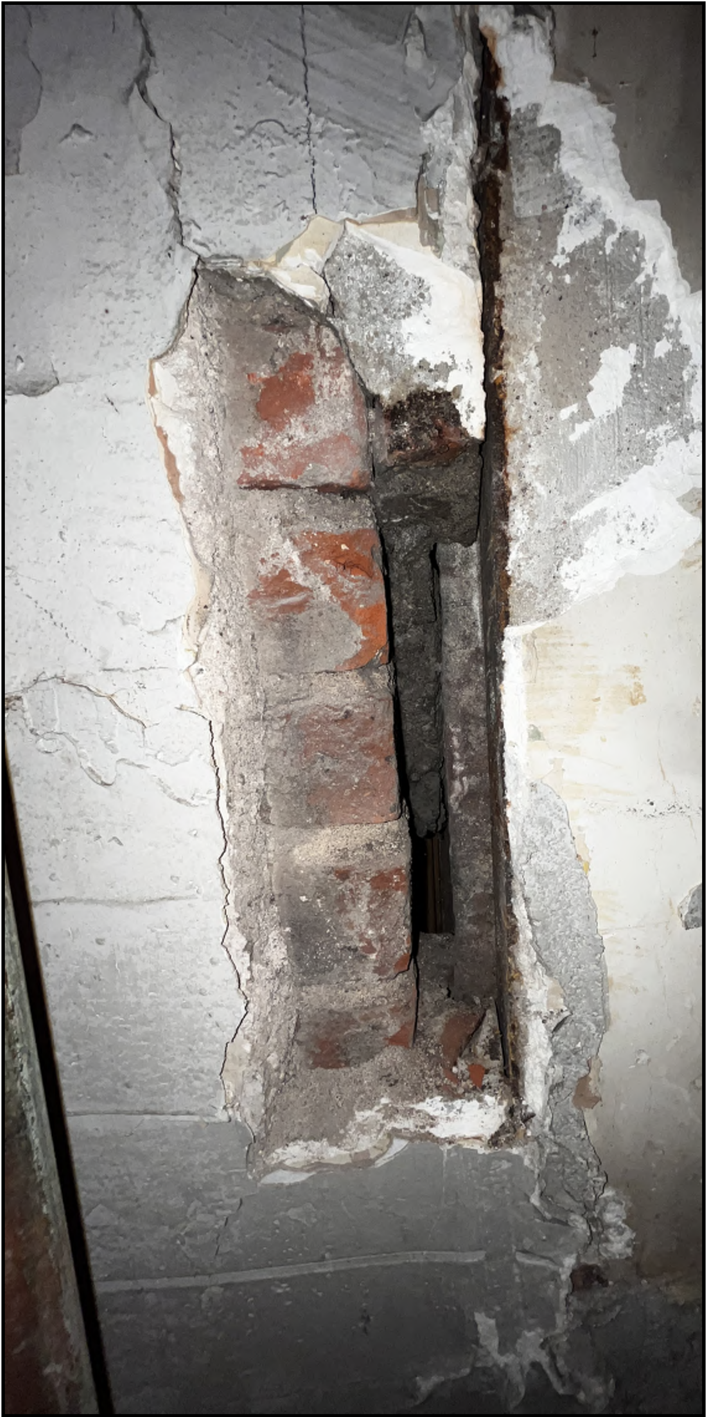
PROBE LOCATION AT SOUTH PARTY WALL TO VERIFY BROWNSTONE PIER VS. CAST IRON COLUMN.
