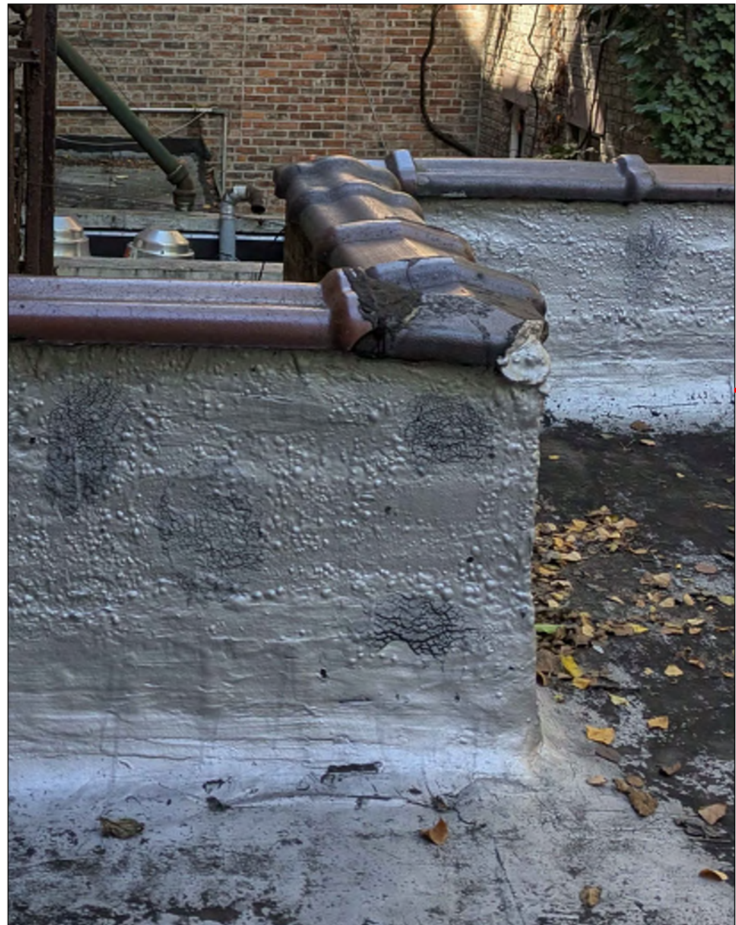
ROOFING & PARAPET IN POOR CONDITION
