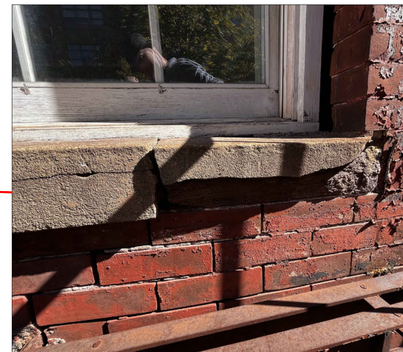
CRACKED, DISLOCATED & SPALLED CEMENTITIOUS PARGING OVER BROWNSTONE WINDOW SILLS
