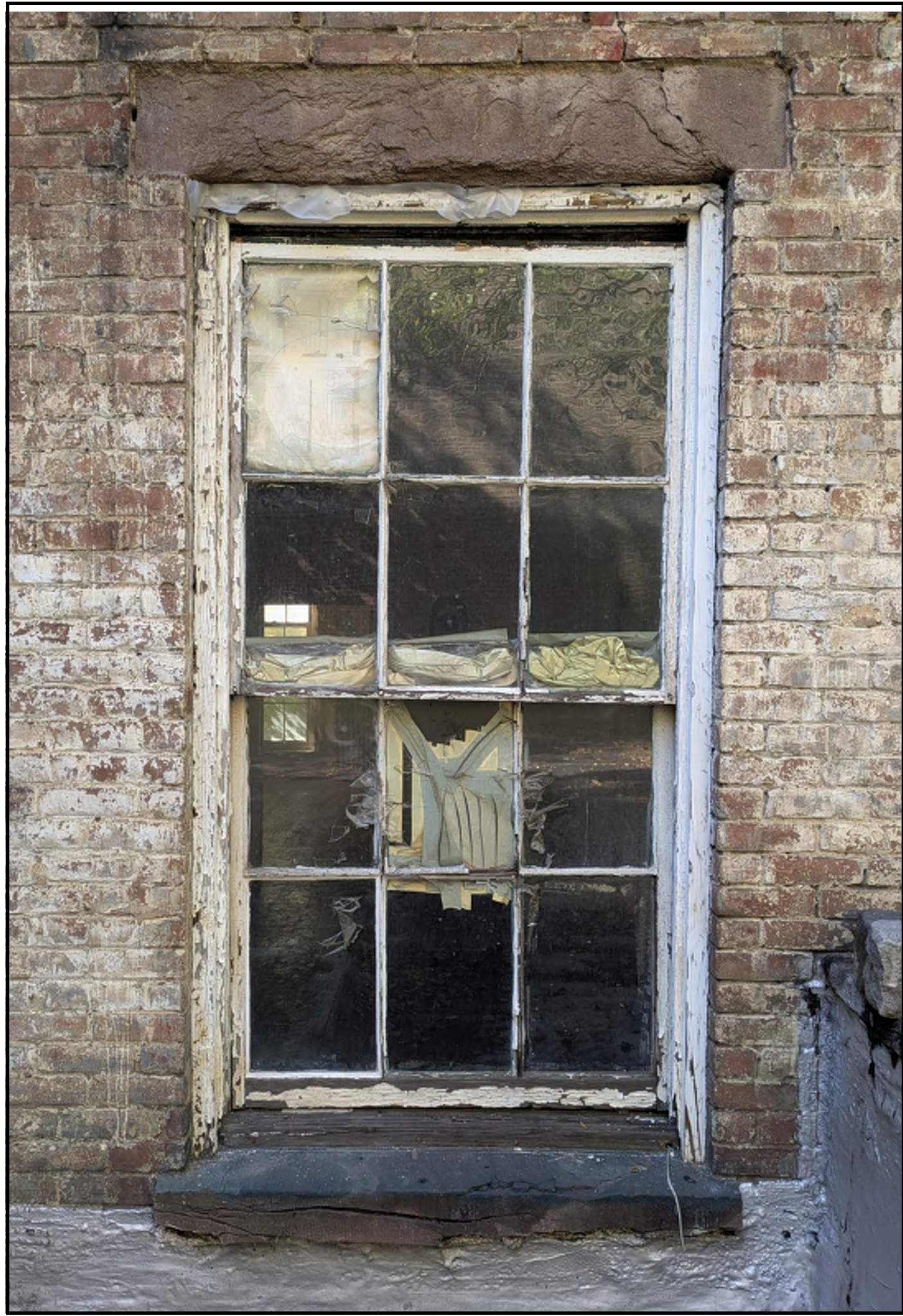
REAR FAÇADE – 2ND FLOOR: HISTORIC 6-OVER-6 DOUBLE-HUNG WOOD WINDOW w/PEGGED JOINERY. TO BE USED AS REFERENCE FOR PROPOSED FRONT & REAR
