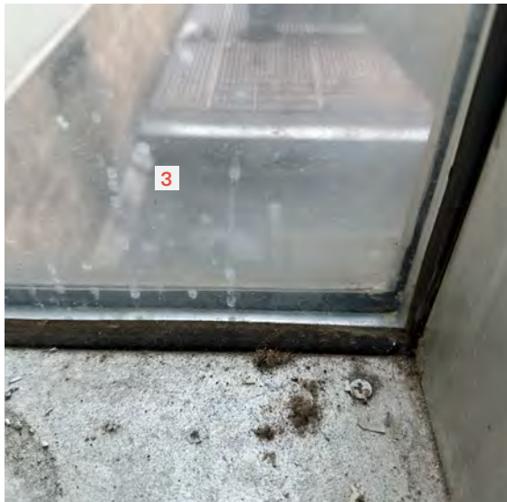
Existing IGU with foggy internal cavity
