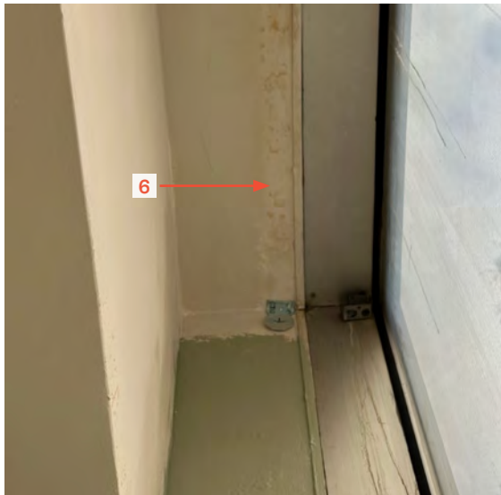
Condensation and interior finish damage
