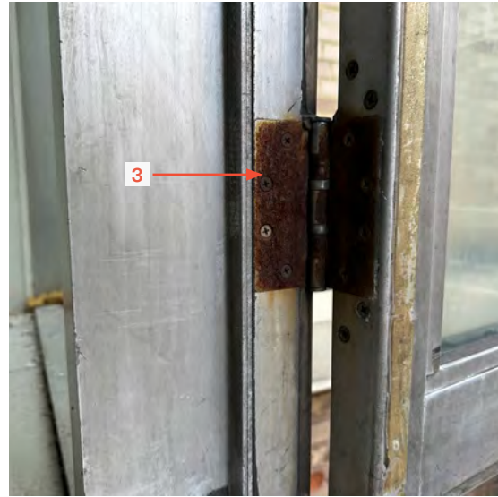
Non-thermally broken aluminum window
