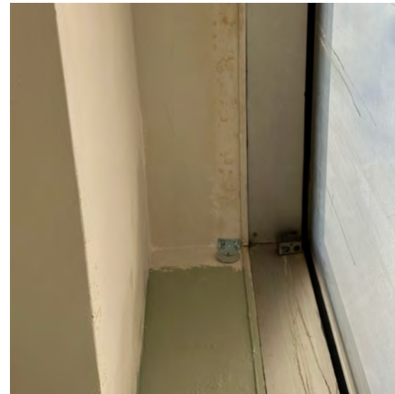
Condensation and interior finish damage
