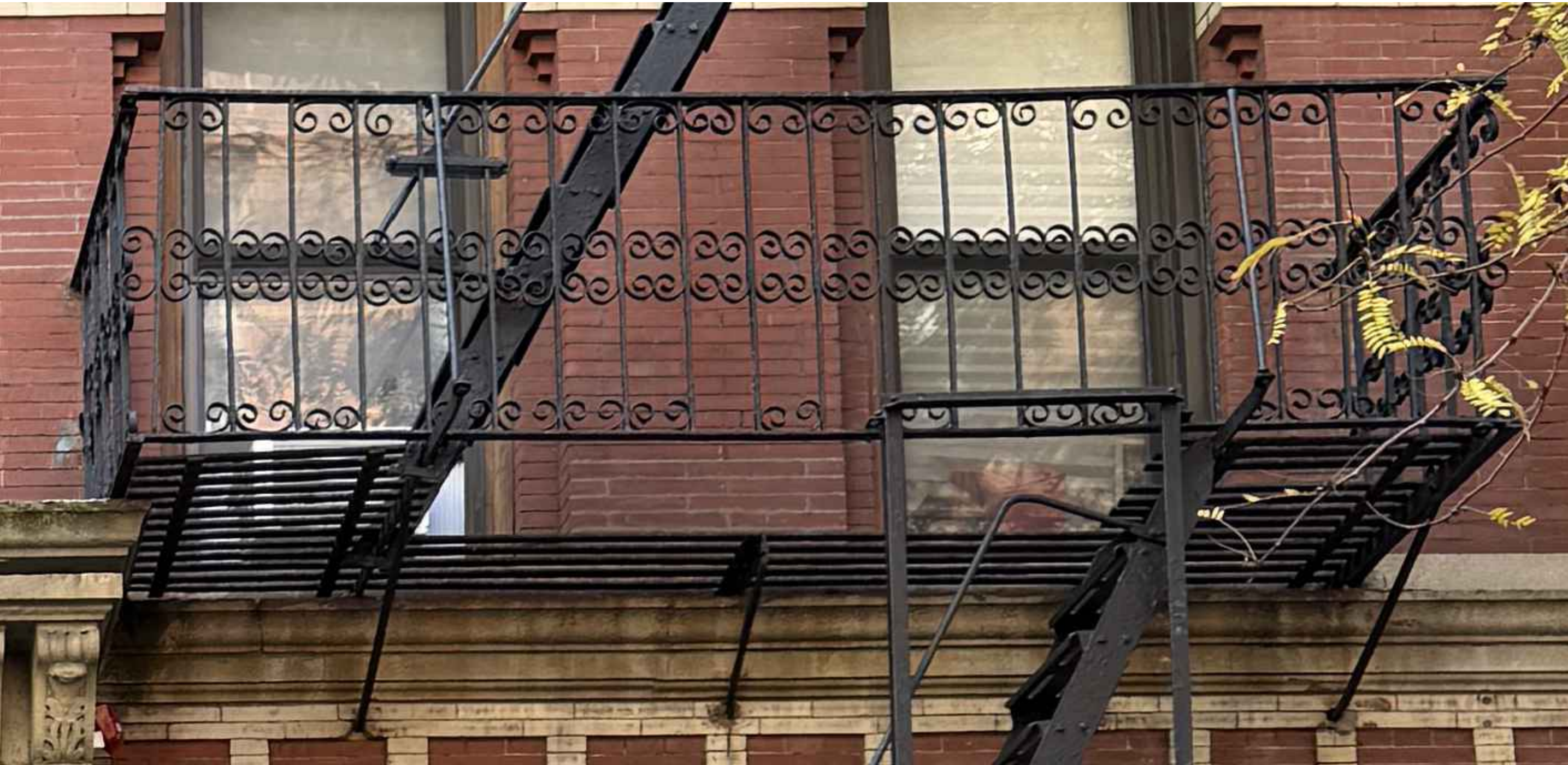
EXISTING FIRE ESCAPE RAILING
