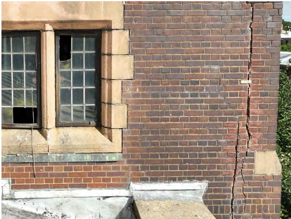
Brick cracking & leaking at underlying steel structure
