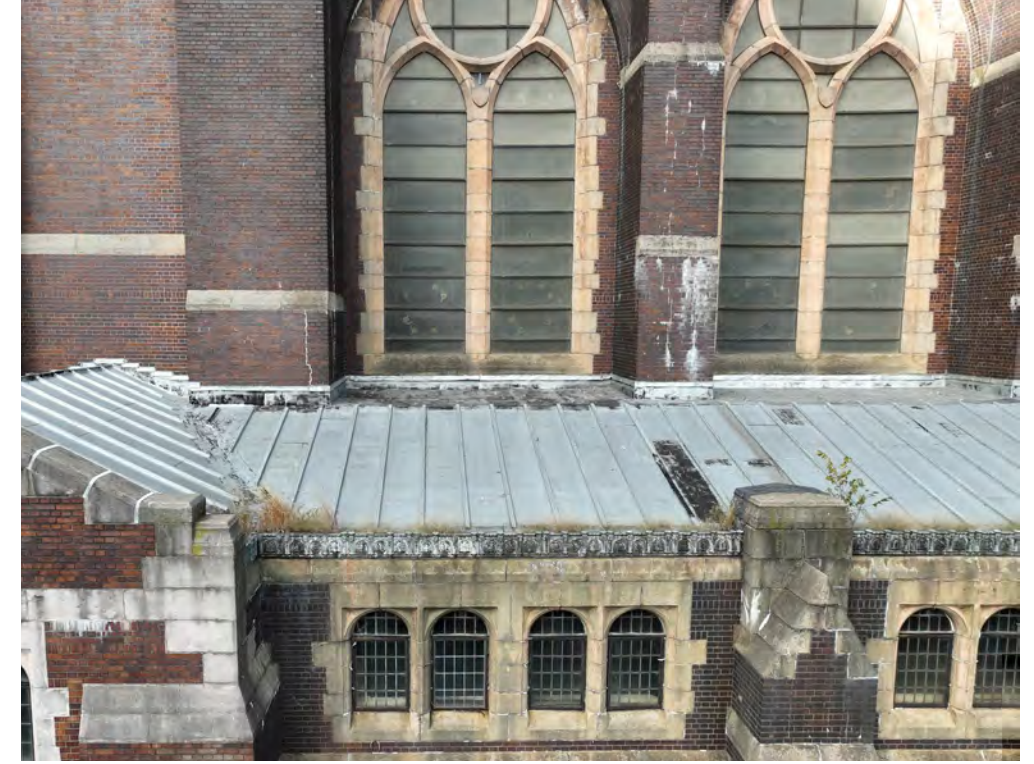
Terra cotta type cast stone tracery
