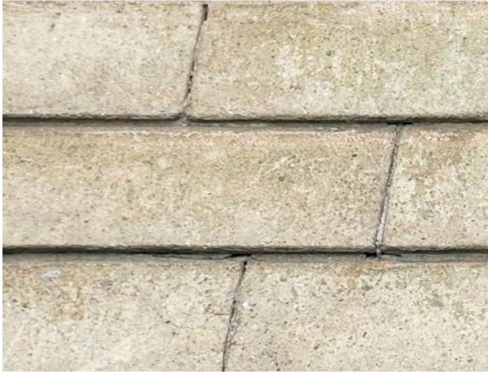
Limestone type cast stone bands
