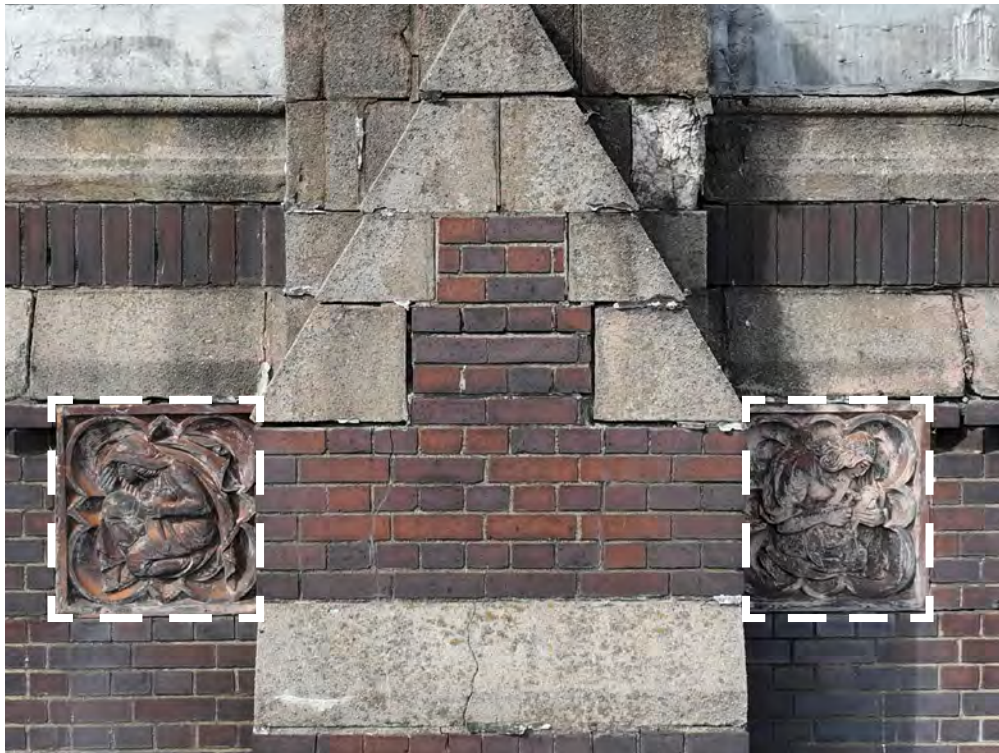
Terra cotta type cast stone plaques
