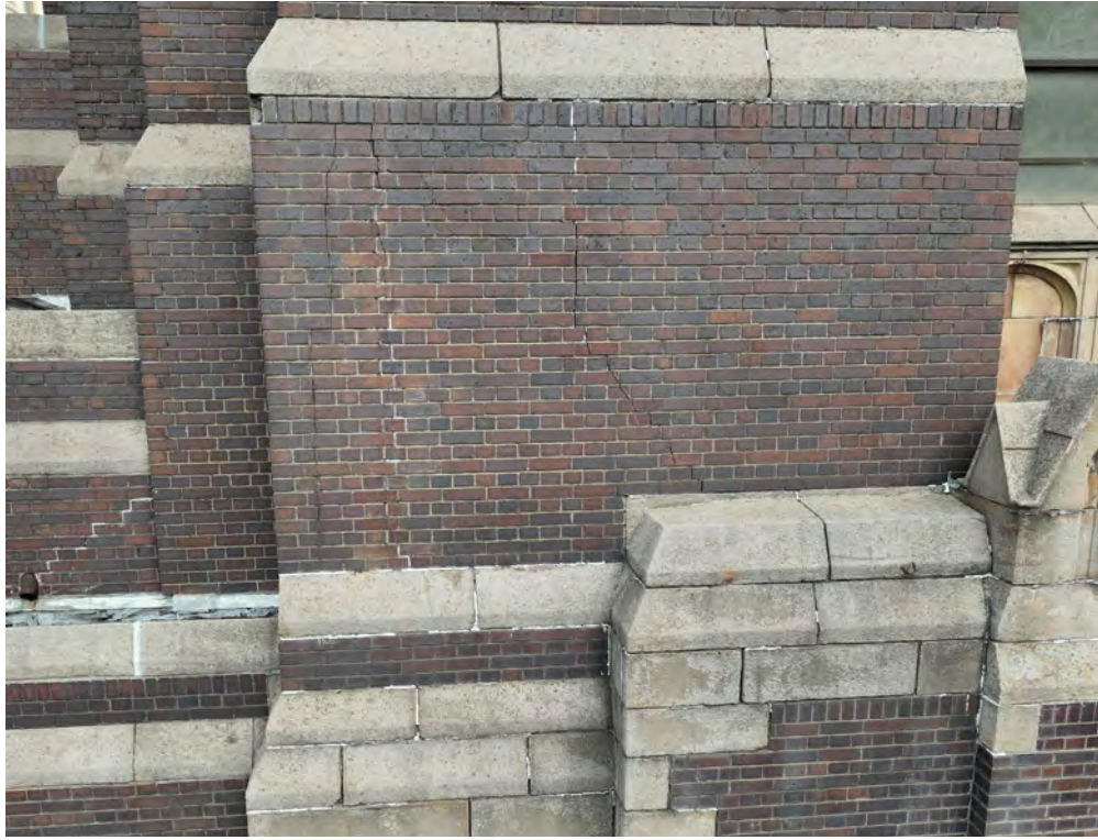
Limestone type cast stone bands
