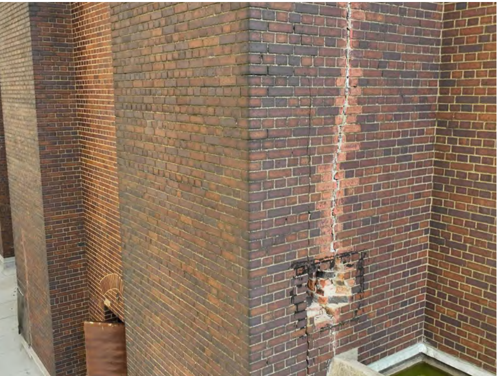
Missing brick and exposed steel structure
