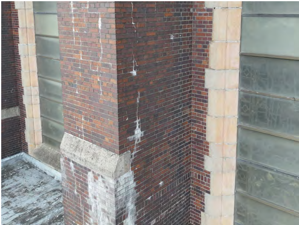
Brick cracking and major efflorescence
