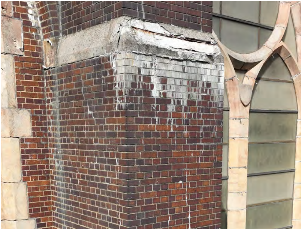
Spalling cast stone
