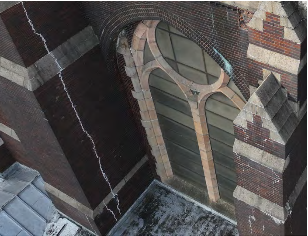
Major brick cracking
