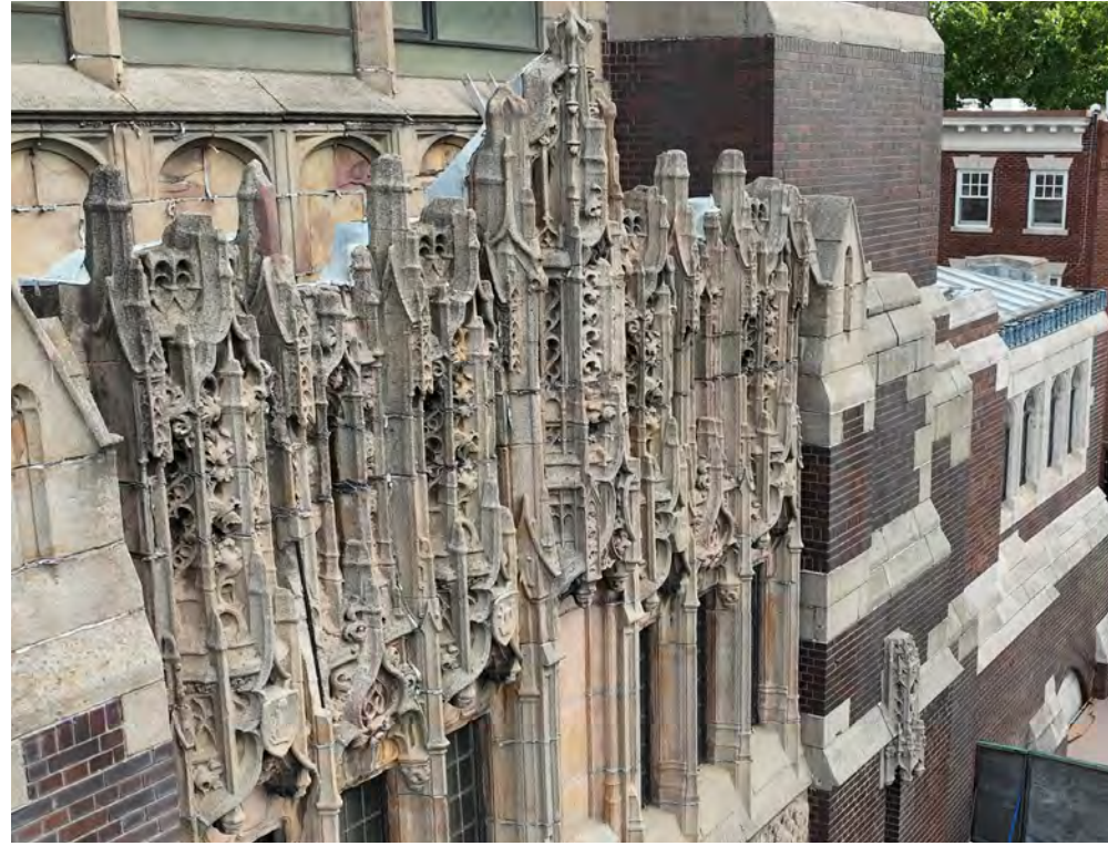
Terra cotta type cast stone tracery
