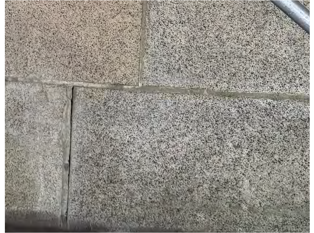
Granite type cast stone base
