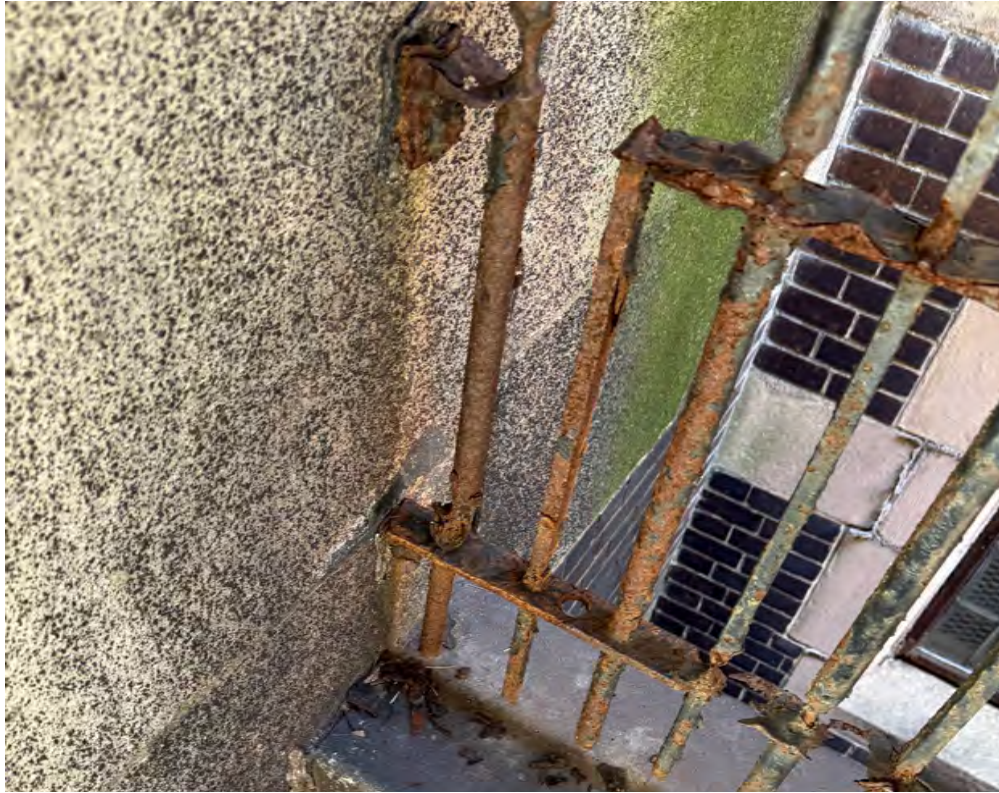
Corroded metal railing
