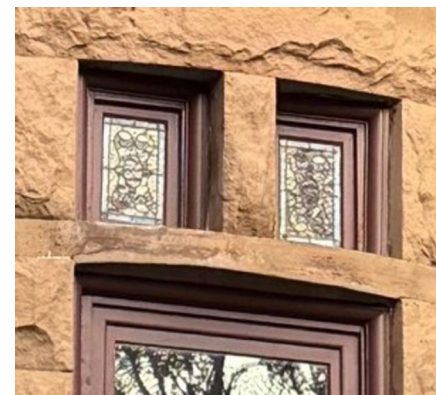
REINSTALLED TRANSOMS - PARLOR FLOOR
