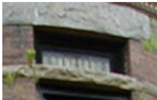
REMOVED TRANSOM - SECOND FLOOR
