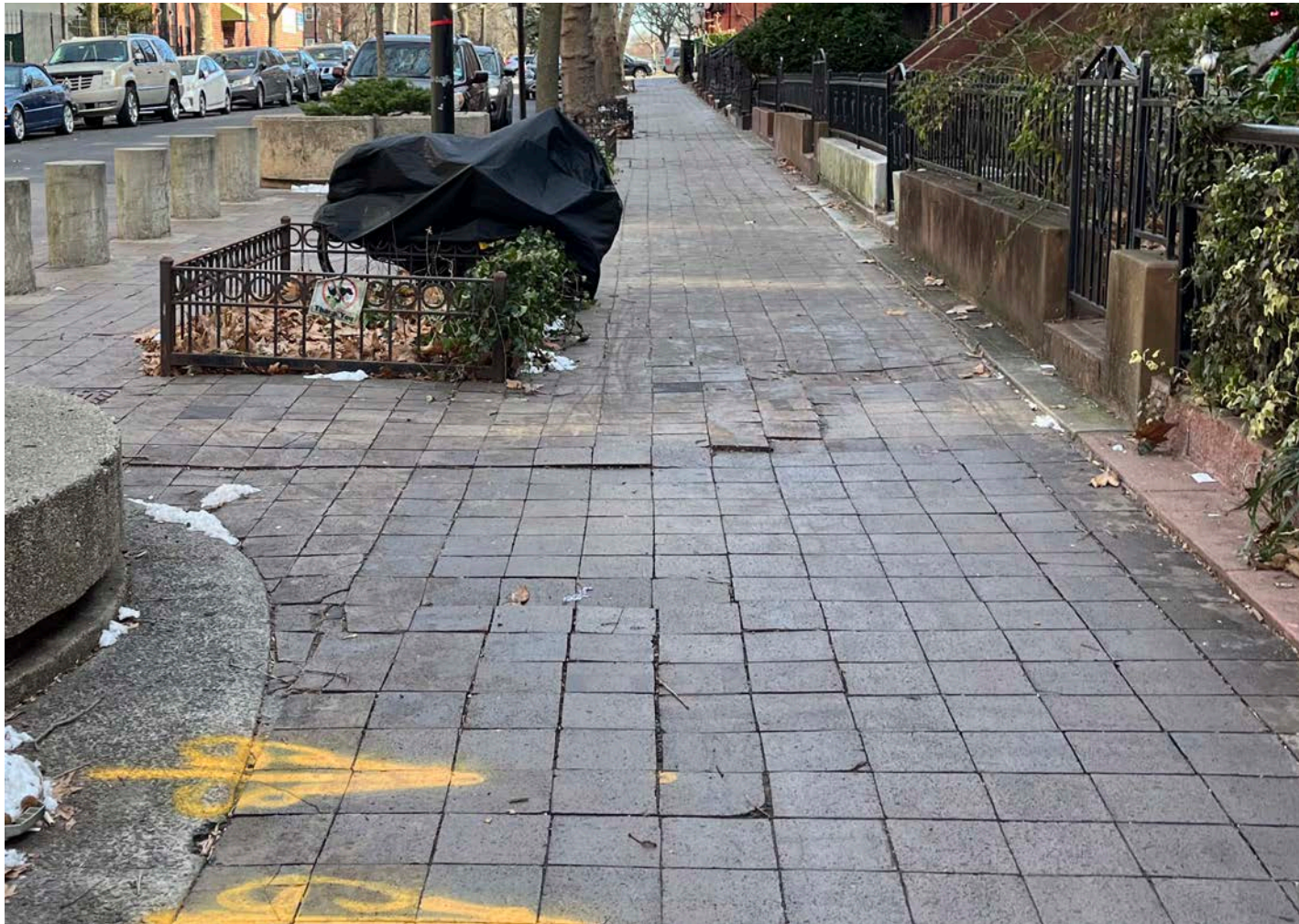
1 - Prospect Place - Example of Uneven and Damaged Brick Pavers
