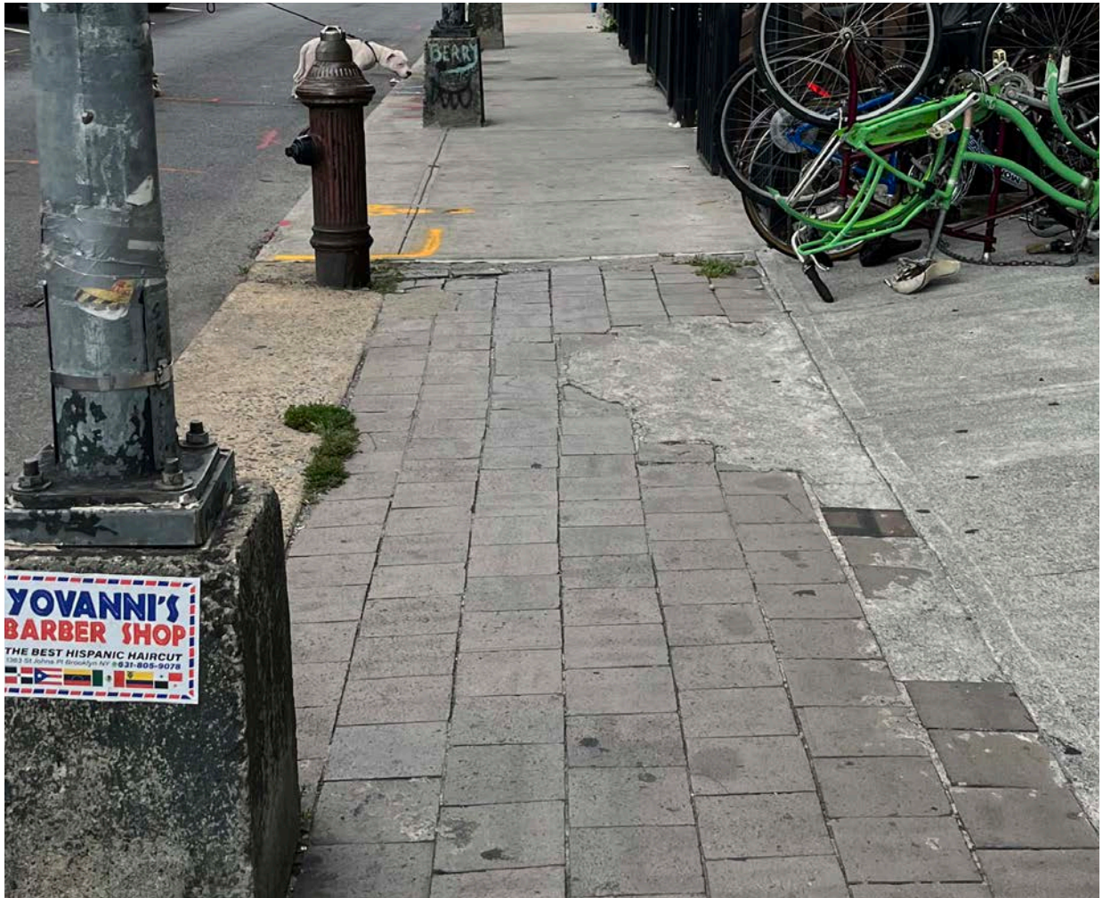
3 - St. Mark's - Original Patched Pavers abutting Redone, Natural Gray Concrete
