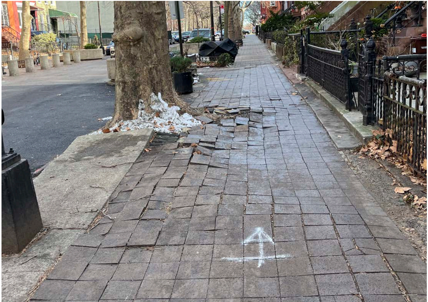
2 - Prospect Place - Example of Uneven and Damaged Brick Pavers
