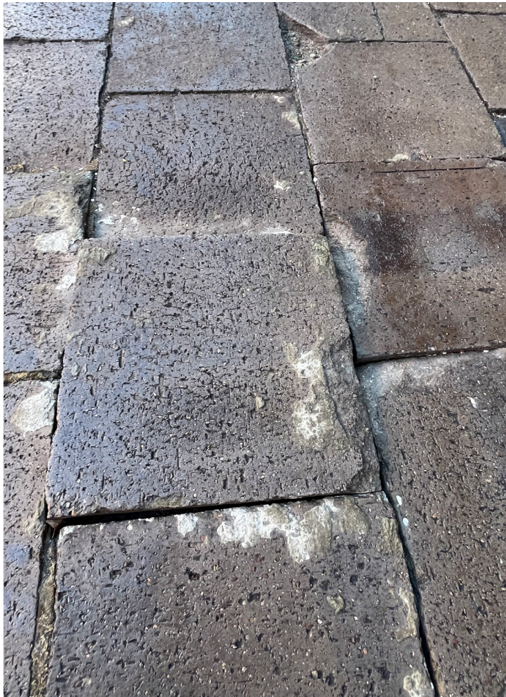
1 - St. Marks - Original, Uneven, Cracked, Broken, Existing Pavers on St. Mark's (2025)
