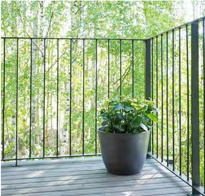
TERRACE RAILINGS ALUMINUM WITH CHARCOAL PAINT FINISH
