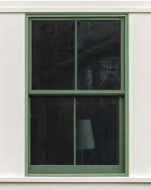
FRONT FACADE WINDOWS MARVIN WOOD DOUBLE HUNG G2 WINDOW, PAINTED GREEN TO MATCH EXISTING
