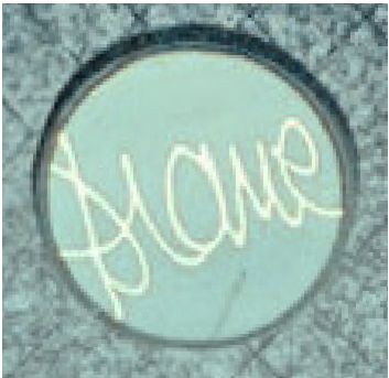
Original signage applied to clear glass oculus
